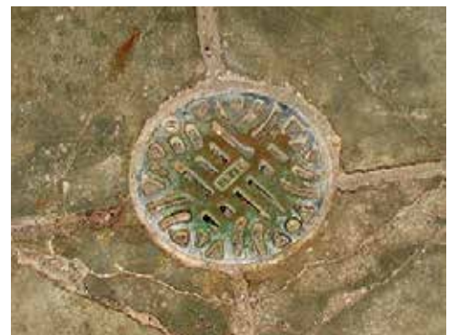
Filled in floor drain.
