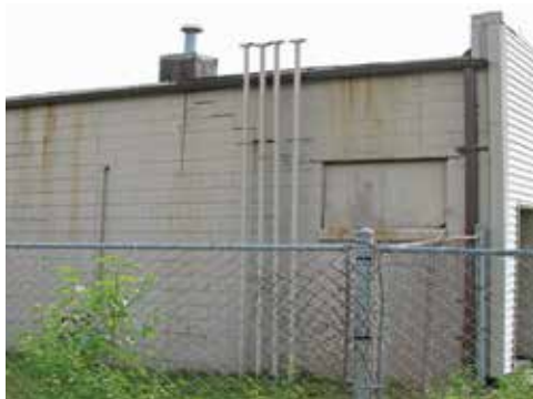
Vent lines for a UST.
