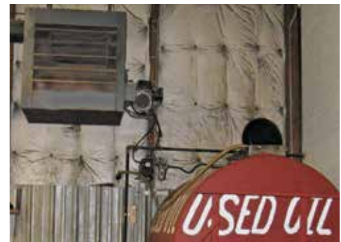
Space heater with labeled used oil storage tank.
