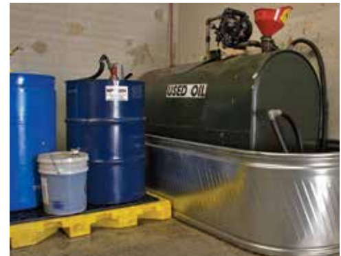
Used oil storage tank in secondary containment.
