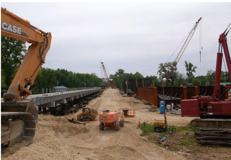
The elevated approach to the new bridge awaits installation of the through-plate girder bridge spans, in right foreground. The old bridge superstructure is in right background.
