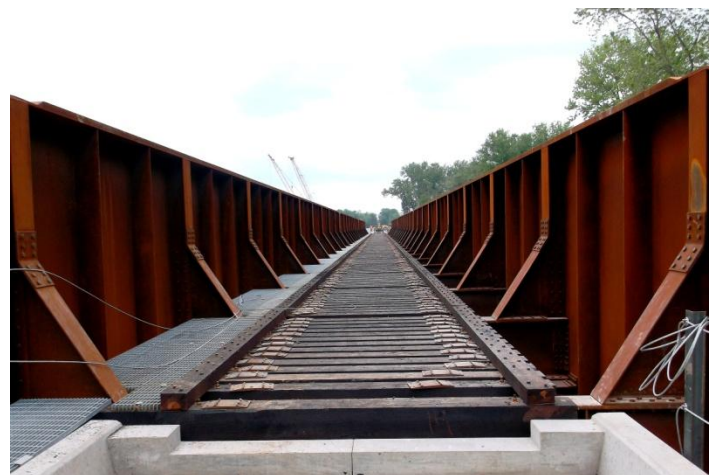
The new bridge span awaits installation of rails.
