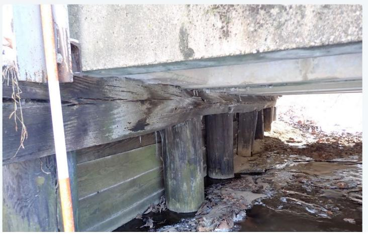
Channel beam bridge with timber abutment caps. East abutment cap has crushed from 12" in depth at the ends to a minimum of 7" in depth in the middle of the structure. West abutment cap appears in GOOD condition. The bituminous wearing surface on the bridge is new and smooth without significant dips.
