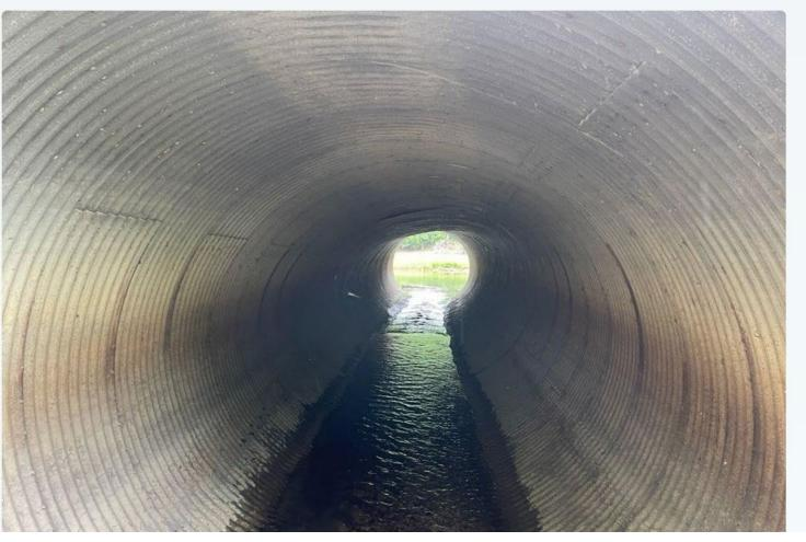
Three-barrel corrugated metal pipe bridge. One of the three pipes shows significant deflection. Little to no corrosion observed in the pipe. Photos from the previous four routine inspections show a similar deflection.
