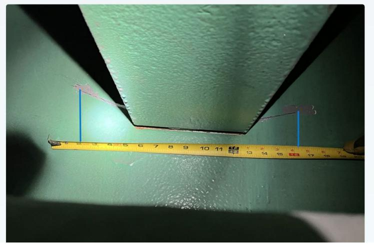
Steel beam bridge with steel diaphragms. Vehicular impact to the exterior beam pushed the diaphragm into the web of the second interior beam cracking it. Bridge is not NSTM. No other beams were damaged by the vehicular impact.
