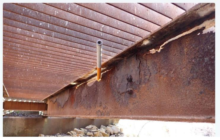
Weathering steel beam bridge with a steel grid deck. Carries rural traffic over a waterway. Beam number 5 of 9 shown. Total separation between the top flange and the web over 90% the length of the beam. Adjacent beams show measurable section loss, but not as severe as this one.
