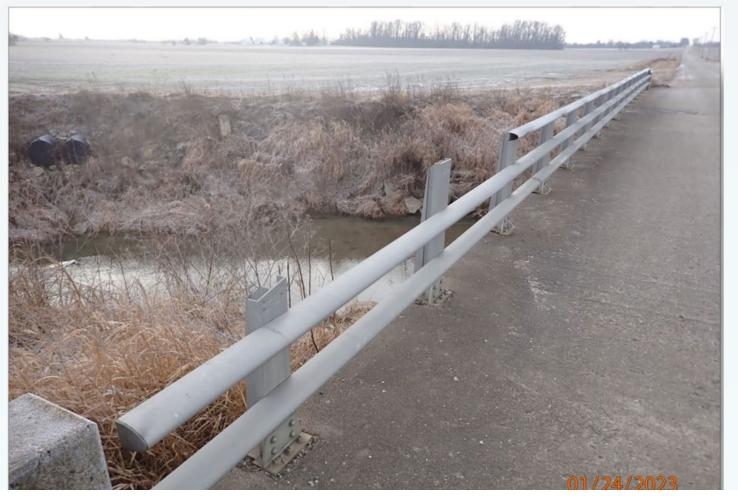
Reinforced Concrete Slab bridge over a waterway. Uppermost section of 3-part bridge rail is missing over end 15' of structure. Deck-mounted rail attachments are in GOOD condition.
