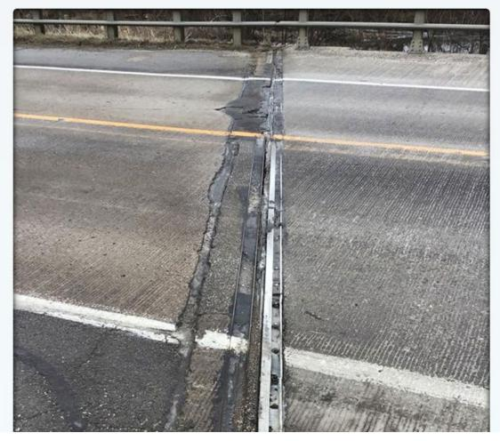
Deteriorated bridge joint. Water infiltration is evident when looking from under the bridge. Joint failed full width with small patched and spalls.
