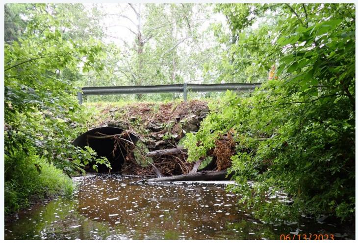
Two-barrel Corrugated Metal Pipe bridge carrying rural road. Left pipe is 30% blocked by drift, and the right pipe is 80% blocked by debris. No active scour was observed at the pipe inlets.
