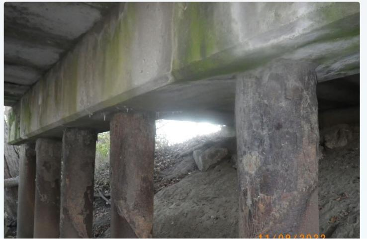
Adjacent PCBB bridge on open pile piers. Steel piles are severely corroded at the pier caps with more than 50% section loss. Some holes observed completely through the steel. Bridge plans show shell piles are filled with reinforced concrete.
