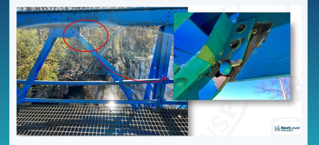
Single-Span steel truss bridge. Vehicle impact damaged one of the diagonal members. In the left photo, the damaged member is one panel to the left of midspan. Detail photo shows two broken rivets and a fracture in the diagonal member.
