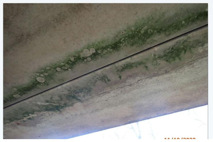
Adjacent PCBB bridge. One new longitudinal crack observed in the exterior beam. Bridge is not currently required to be posted for load.
