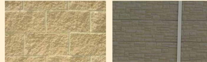
Noise barriers typically consist of concrete panels placed between steel supports. The height and location of a barrier is determined by the TNM analysis. The color and texture can vary, and INDOT seeks the input of adjacent property owners.
