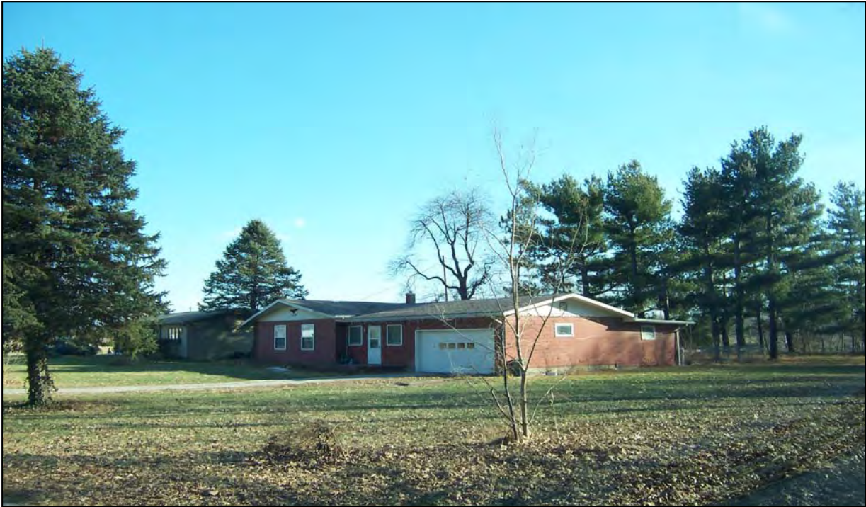
Looking southeast at currently occupied residence (120 Aretz Lane)
