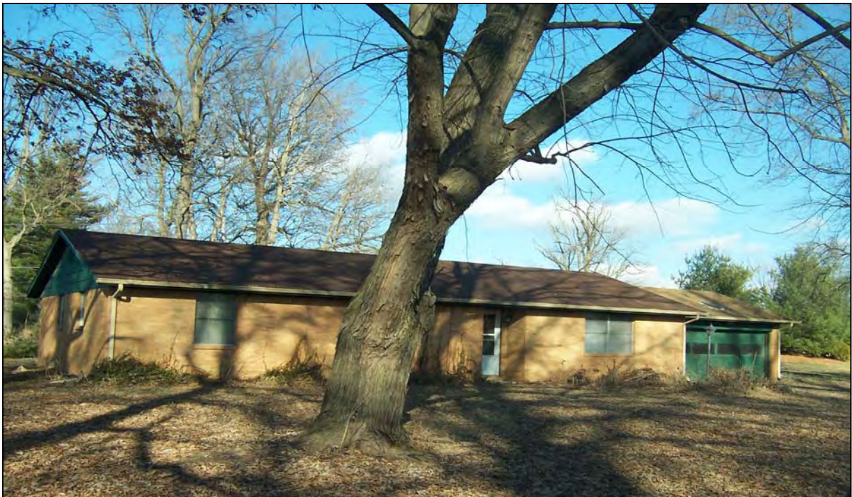
Looking north at apparently abandoned residence (50 Aretz Lane)
