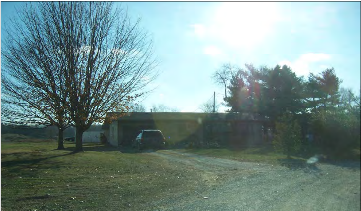
Looking south at currently occupied residence (130 Aretz Lane)
