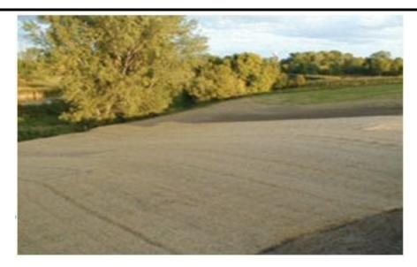
Rolled erosion control products provide numerous benefits: immediate bank protection and stabilization; protection of vegetation as it becomes established; providing a stable microclimate for enhanced growth; and increased soil infiltration which promotes improved drainage and vegetation growth. These materials are often used in conjunction with other bioengineered materials such as A-jacks and live fascines.
