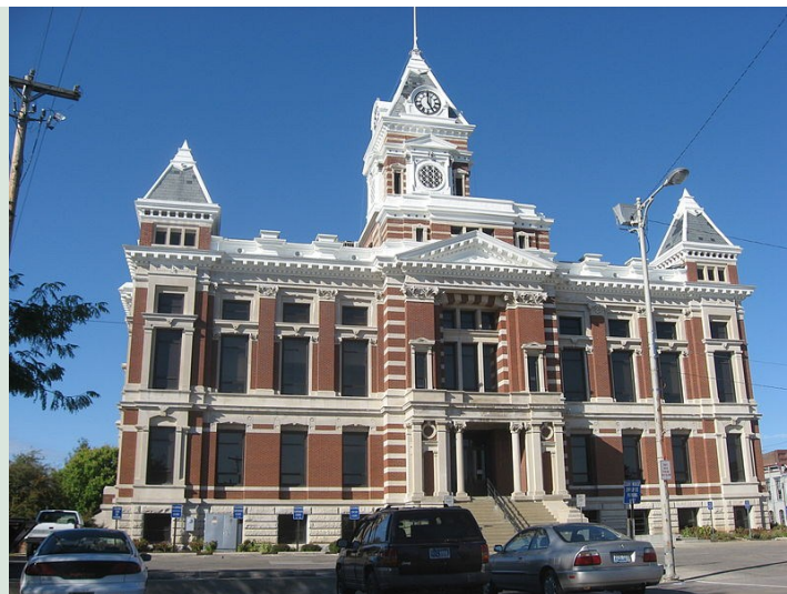
Johnson County Courthouse. Source: Wikimedia.org
