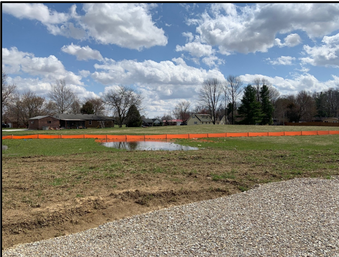
View from parking lot area, looking east at Blue River Trails (Staff Photograph – March 2021)
