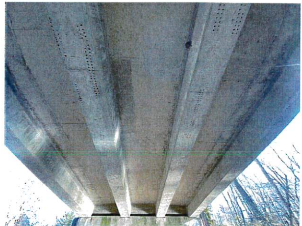
Looking at Bottom of Beams and Deck Span B
