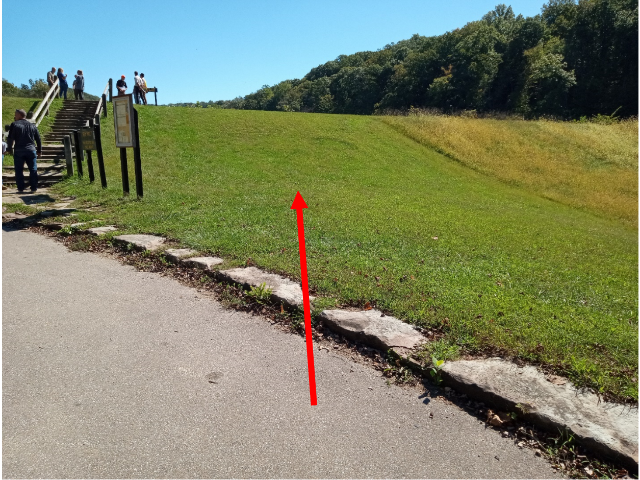
Dam crest access location. Contractor to protect asphalt parking and stone curb. Return back to existing condition.
