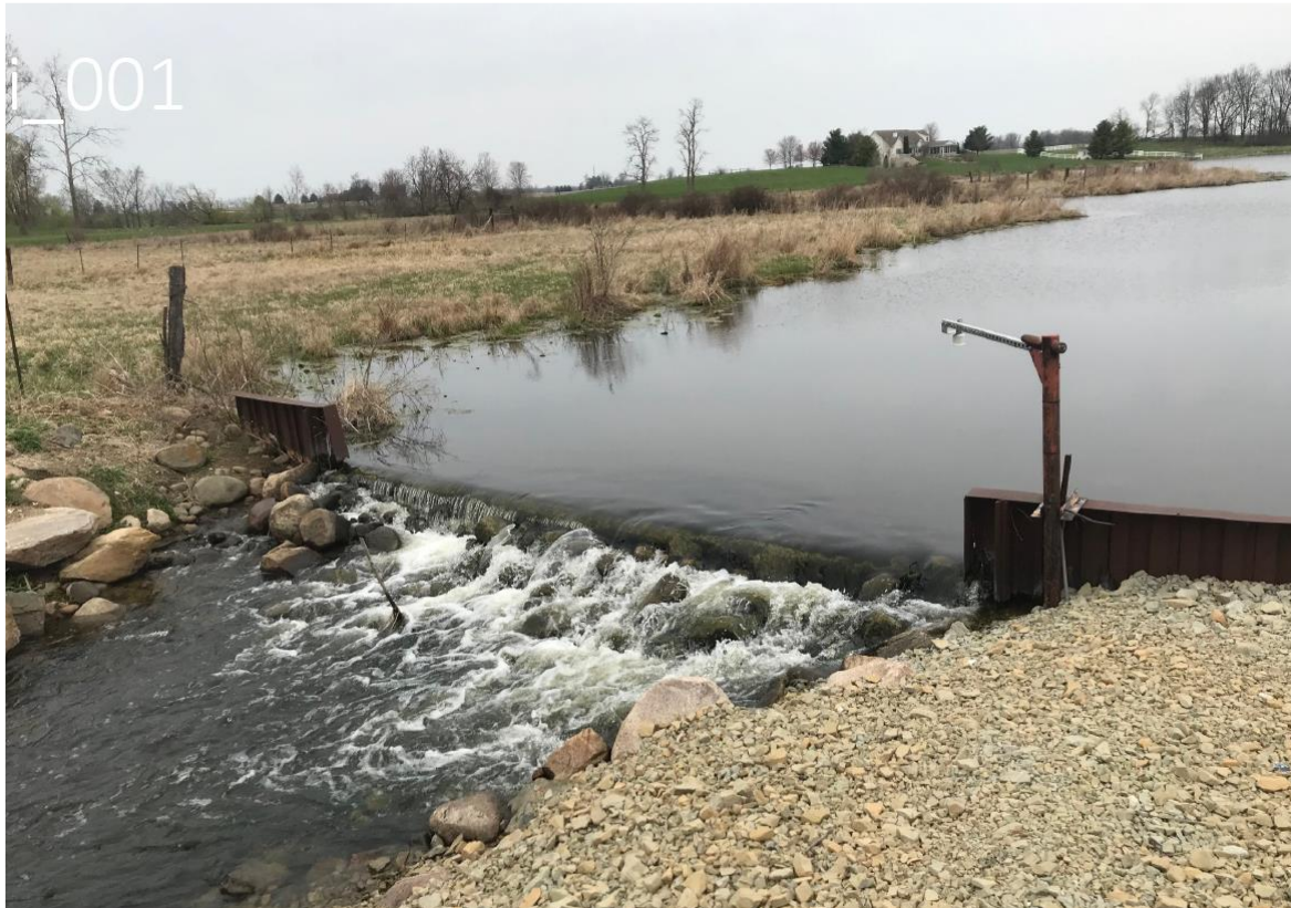
Figure 1: Existing Dam – Taken from East Bent Looking North
