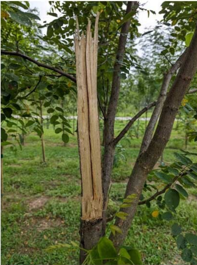
Photo 6 - A wider shot showing the damage and poor form caused after possible locust borer damage plus wind damage.
