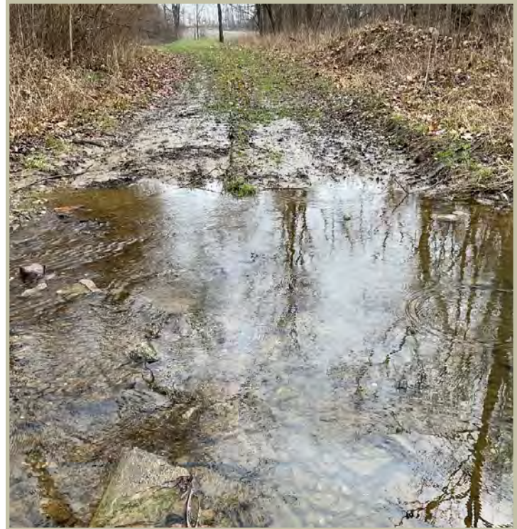
This low ford crossing is well done, with the exception that water should have been diverted prior to crossing. Photo taken on private property by Duane McCoy, DNR.
