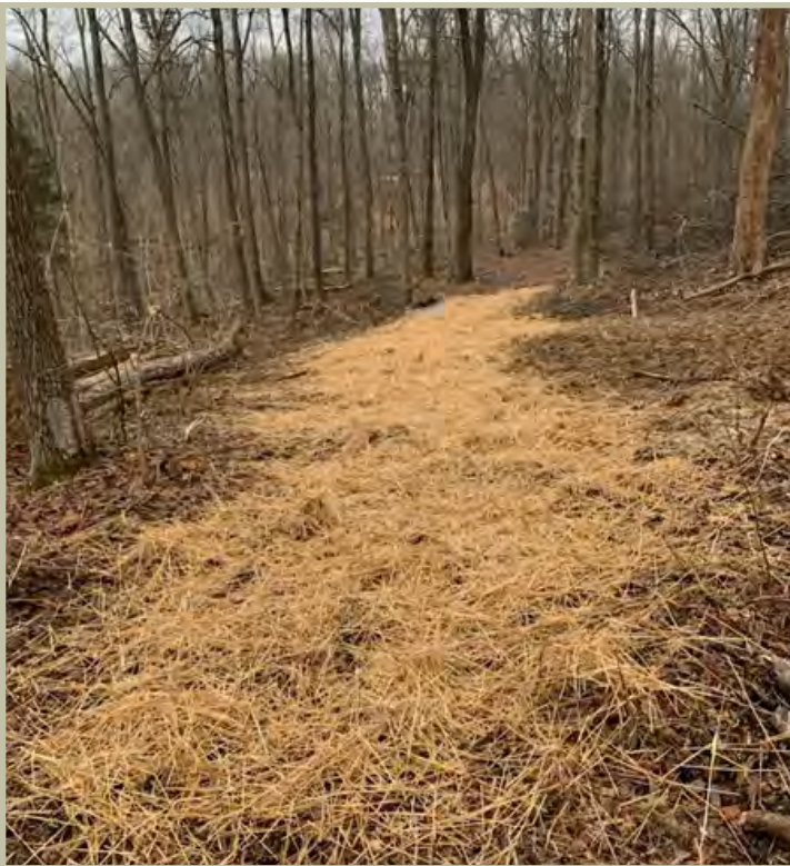
This skid trail was mulched with straw after a harvest on state forest land. Photo by Duane McCoy, DNR
