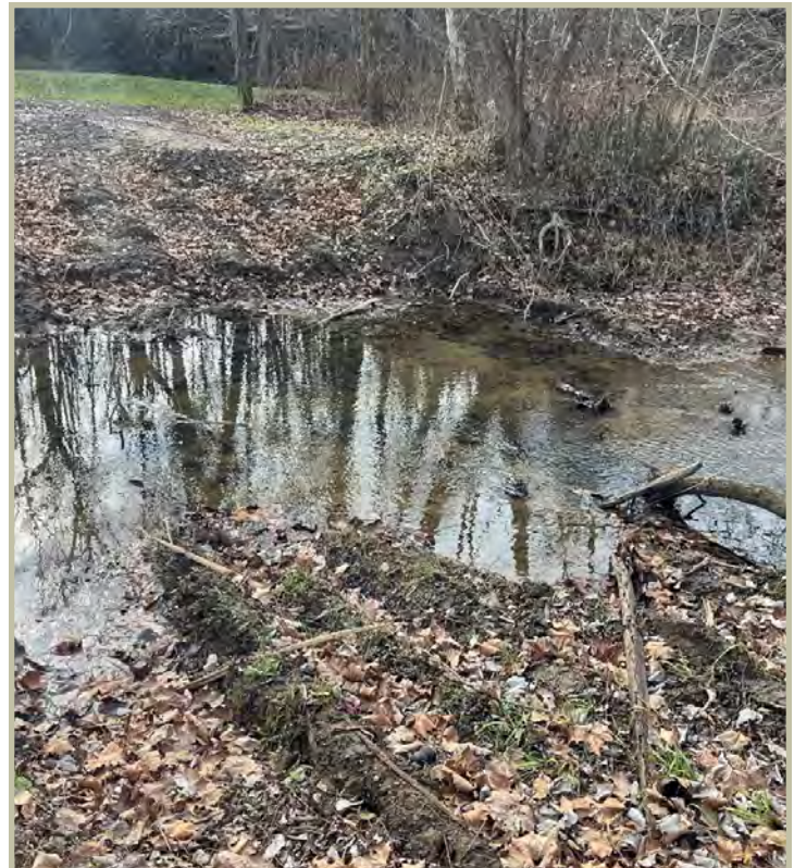
While it appears some sort of bridge or mat was used to cross this stream, it was not smoothed or stabilized after closeout, which will cause erosion for years to come. Taken on private property by Jennifer Sobecki, DNR.
