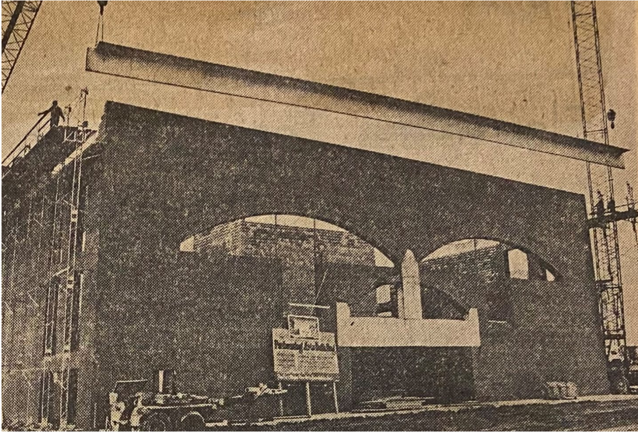
Figure 19. A concrete tee beam is lowered into place during construction of the Fort Wayne Performing Arts Theatre, as published in the Fort Wayne News-Sentinel , 24 October 1972. (Source: Arts United Center Archives.)
