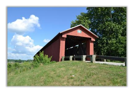
The general terrain around the bridge is flat agricultural land. The stone abutments and tapered center pier are composed of cut stone. The heavy oak timber frame is composed of sawn lumber. Ten panels of heavy
