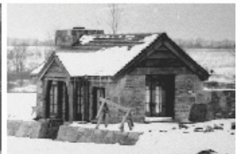
Gatehouse under construction
