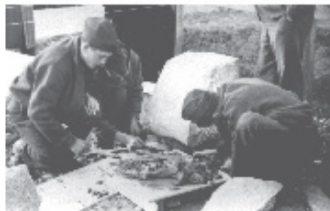
Stone masons building the Spring Shelter
