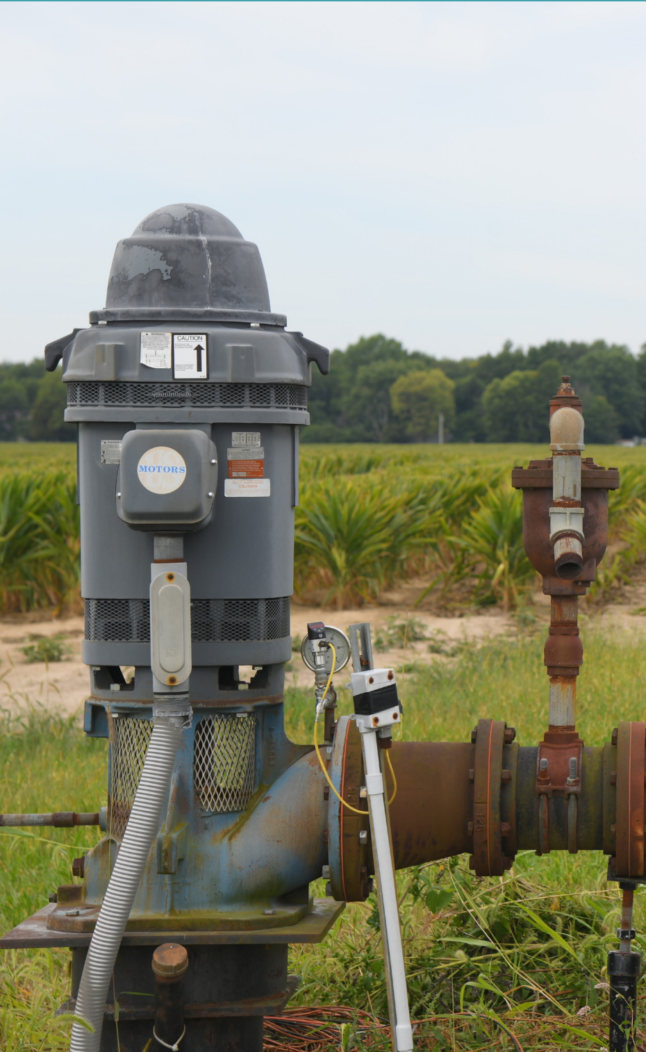
A well used to water agricultural fields in Hamilton County.
