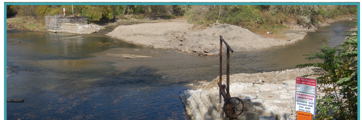
The low head dam removal in October 2024 reinstated flow to the stream channel of the Big Blue River.
