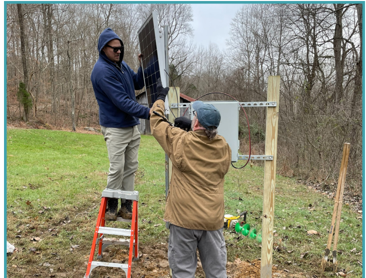
Resource Assessment section manager Garth Lindner (on ladder) and staff geologist Randy Maier install a solar panel to supply power to the telemetry pilot site in Perry County.
