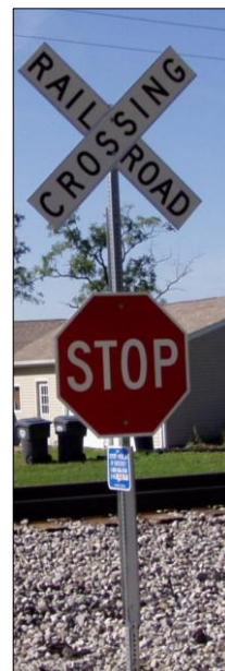
Exhibit 2 Cross Buck Installation
