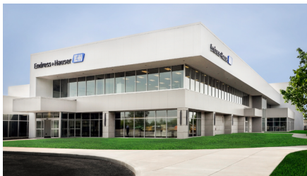
1 Endress+Hauser US (Customer Center) 2355 Endress PI
