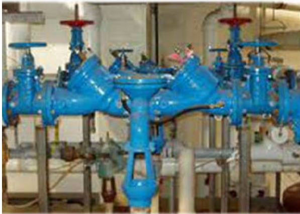
Figure 5.12 – Reduced Pressure Principle Assembly Photo
