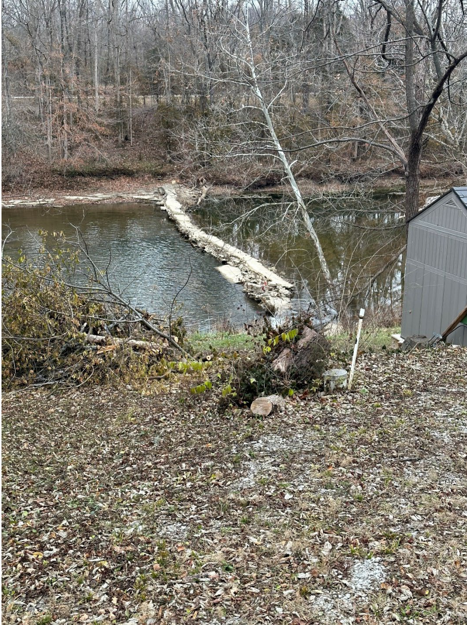
Figure 3. Downstream low-head dam in the Flatrock River at Geneva, Indiana. The dam is approximately 140 feet long and 5-feet tall and 3-feet wide with a pool length of approximately 0.75 miles long. While this is a relatively small dam, the plunge pool is dangerous and a fish passage barrier. There have been no recorded deaths, but injuries have occurred at this dam.
