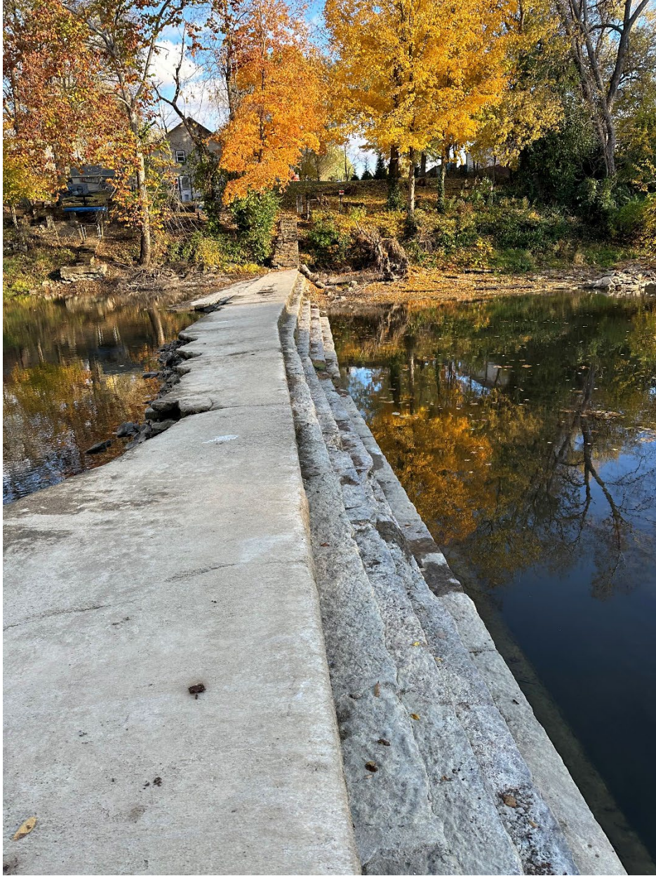
Figure 2. Upstream low-head dam in the Flatrock River at Geneva, Indiana. The dam is approximately 170-feet long and 6-feet tall and 5-feet wide with a pool length of 1.5 miles. This dam is made of cut limestone slabs that will be individually removed. The plunge pool below this dam is dangerous and is a fish passage barrier. There has been a recent death at this dam.
