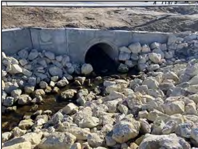
PP5, Looking at Stream 1 culvert (12/13/23)
