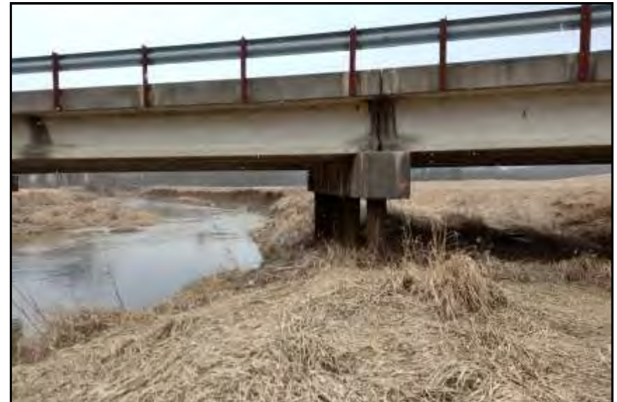
DP01, View Looking West
