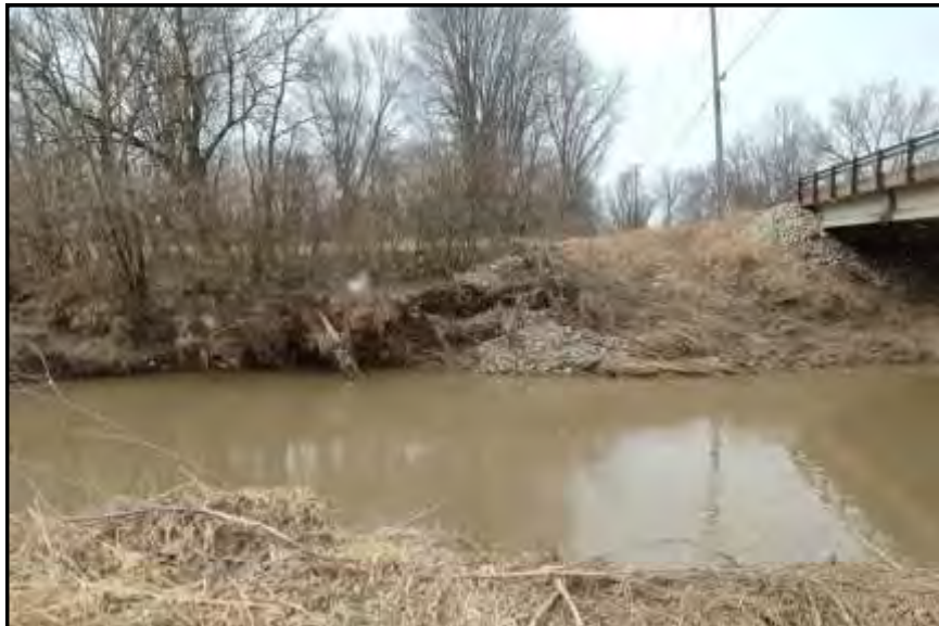
DP01, View Looking South
