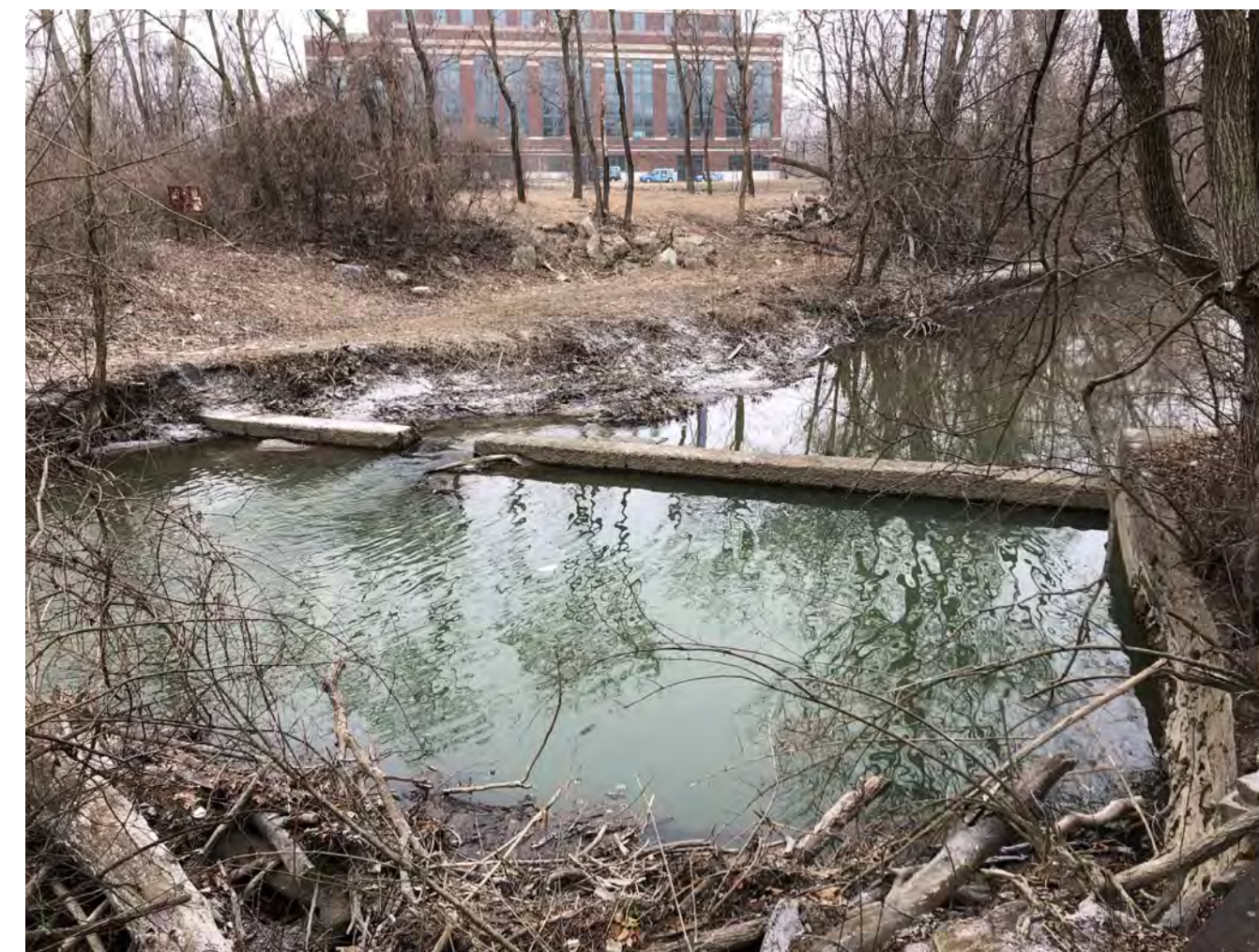
PHOTO TAKEN ON 02/16/2024 LOOKING UPSTREAM AT UPSTREAM DAM FROM EAST BANK
