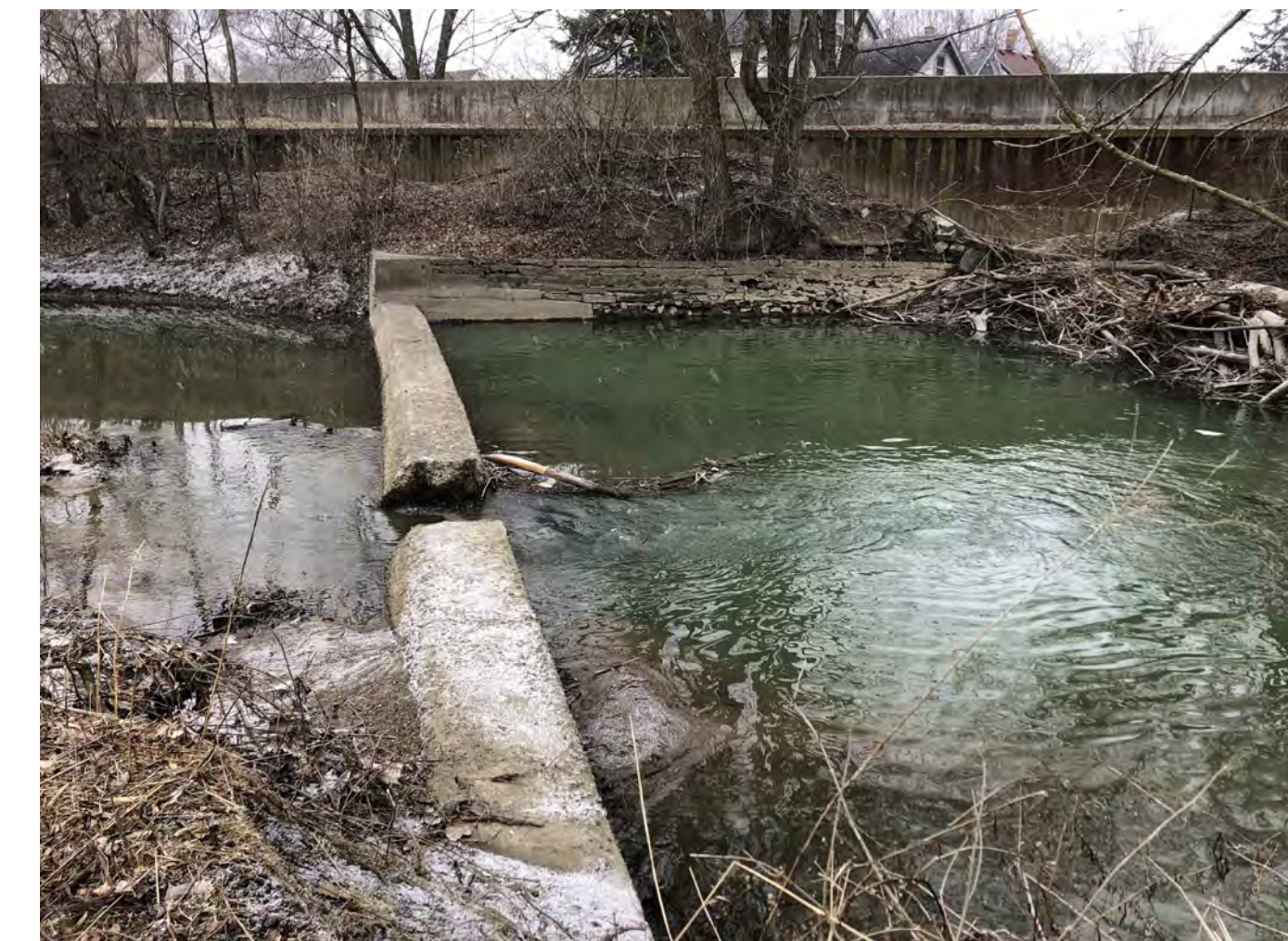
PHOTO TAKEN ON 02/16/2024 ON CREST OF UPSTREAM DAM, LOOKING EAST
