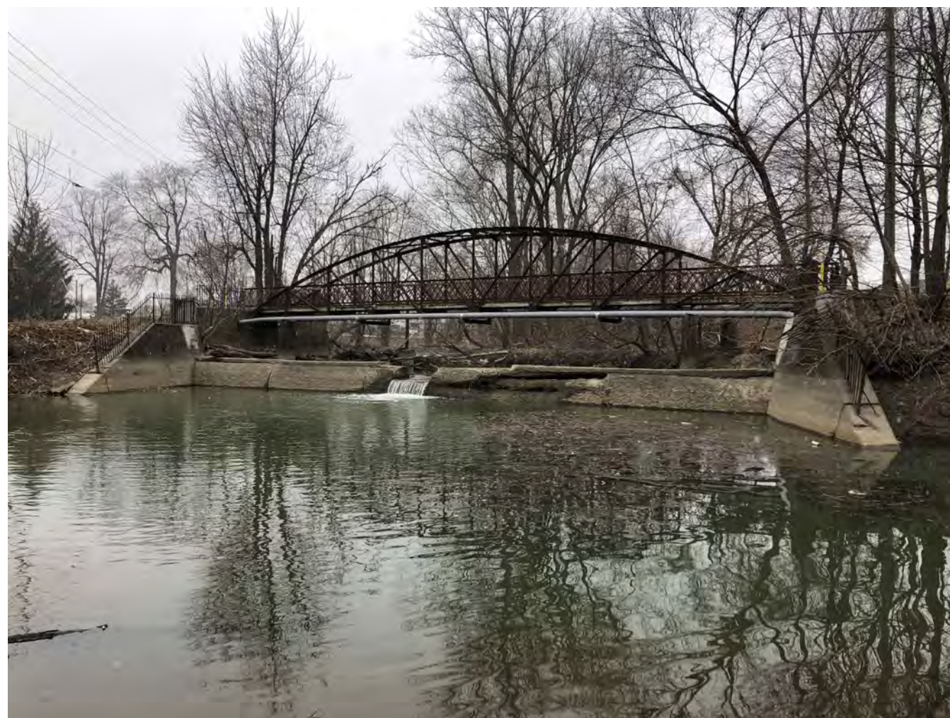
PHOTO TAKEN ON 02/16/2024 LOOKING UPSTREAM AT DOWNSTREAM DAM FROM EAST BANK
