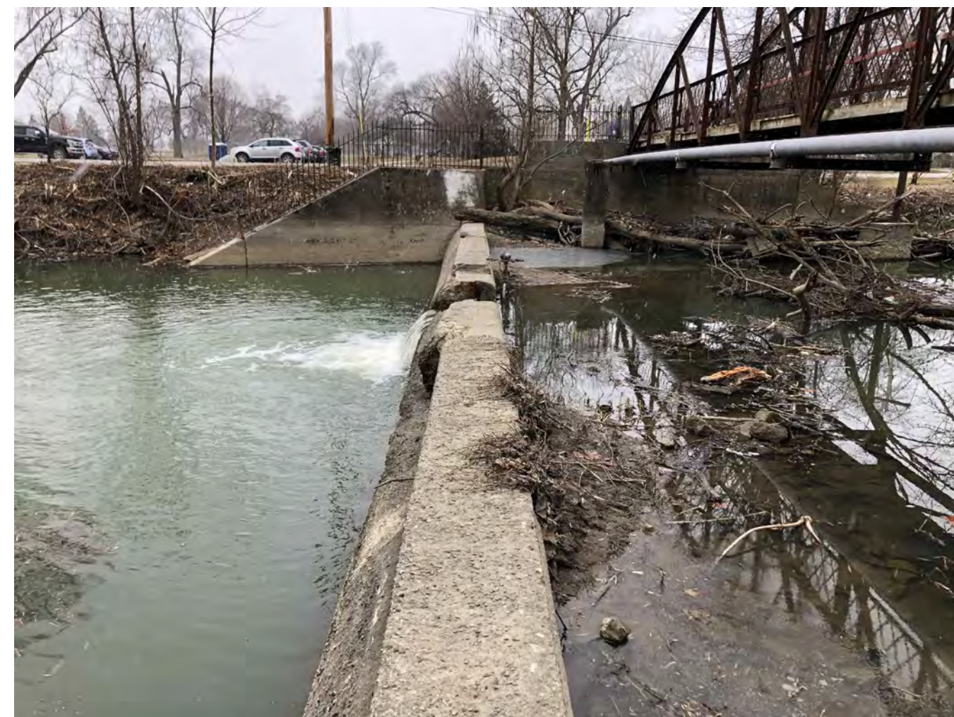
PHOTO TAKEN ON 02/16/2024 ON CREST OF DOWNSTREAM DAM, LOOKING WEST
