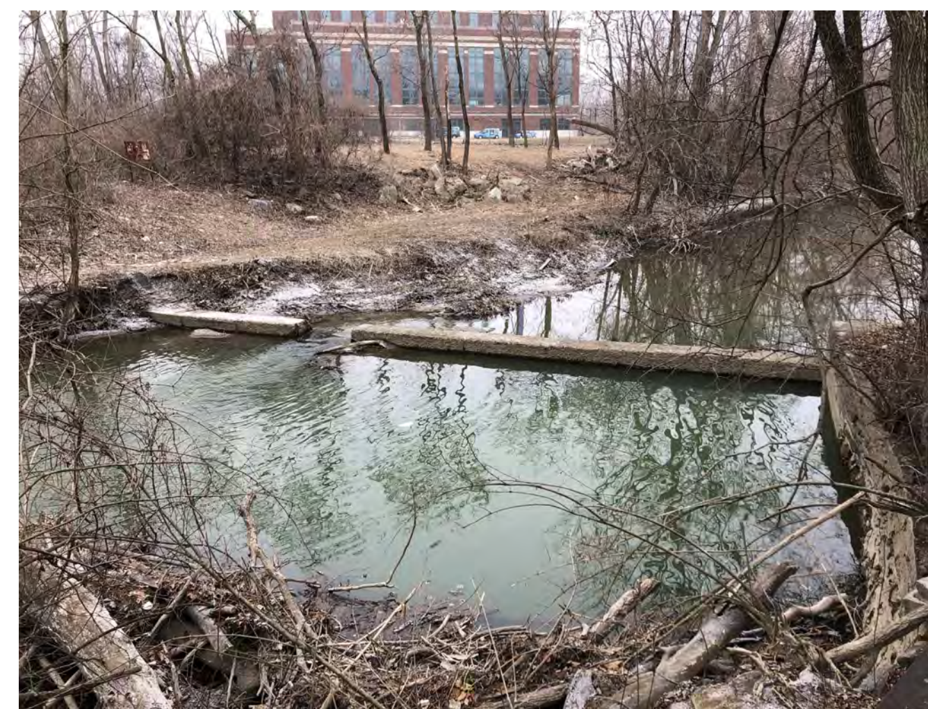
PHOTO TAKEN ON 02/16/2024 LOOKING UPSTREAM AT UPSTREAM DAM FROM EAST BANK
