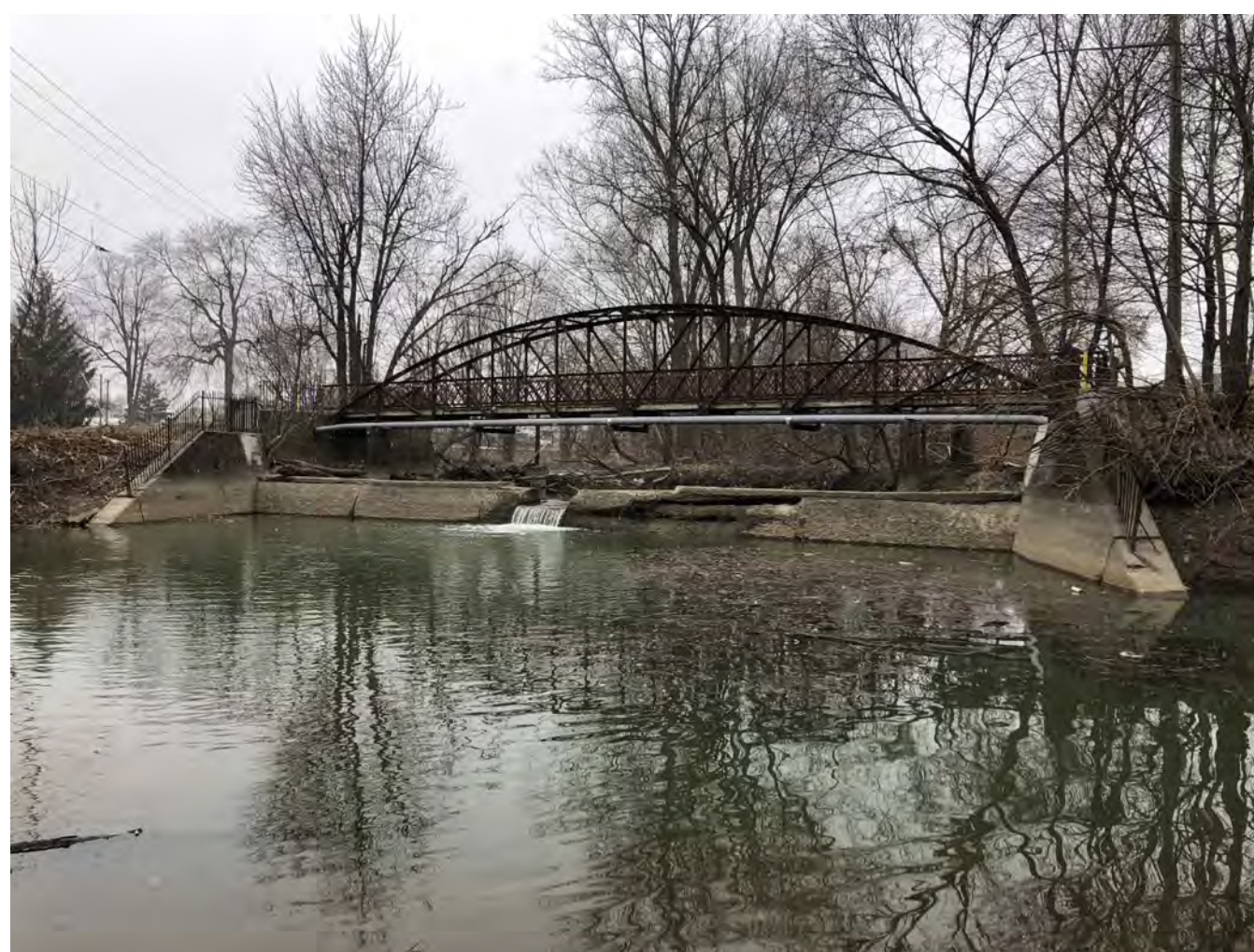
PHOTO TAKEN ON 02/16/2024 LOOKING UPSTREAM AT DOWNSTREAM DAM FROM EAST BANK
