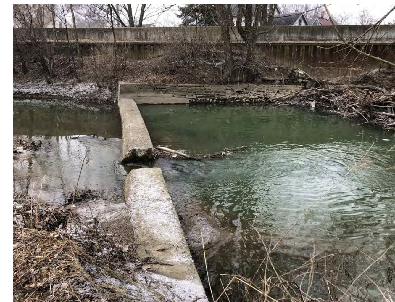
PHOTO TAKEN ON 02/16/2024 ON CREST OF UPSTREAM DAM, LOOKING EAST
