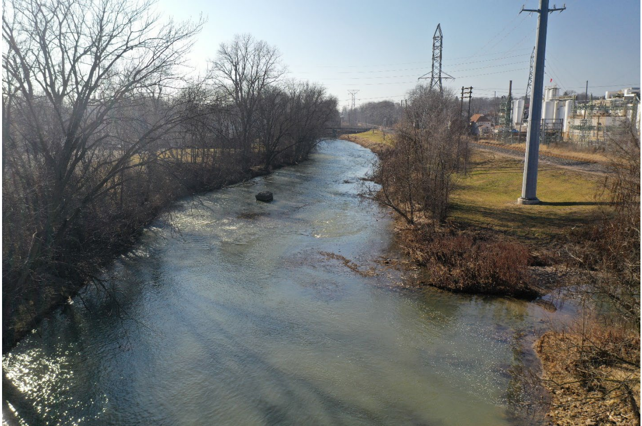
Figure7. Drone picture from the project site looking downstream. Photo taken 5 February 2024. Huntington dam, Huntington Indiana
