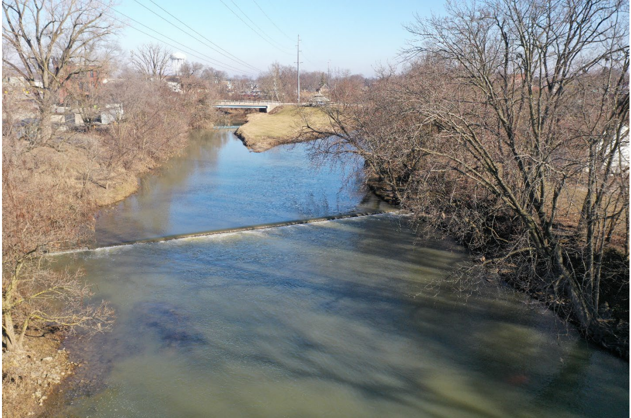
Figure 9. Drone picture from downstream the project site looking upstream. Photo taken 5 February 2024. Huntington dam, Huntington Indiana. The dam is approximately 120-feet long and 4-feet tall and 3-feet wide.
