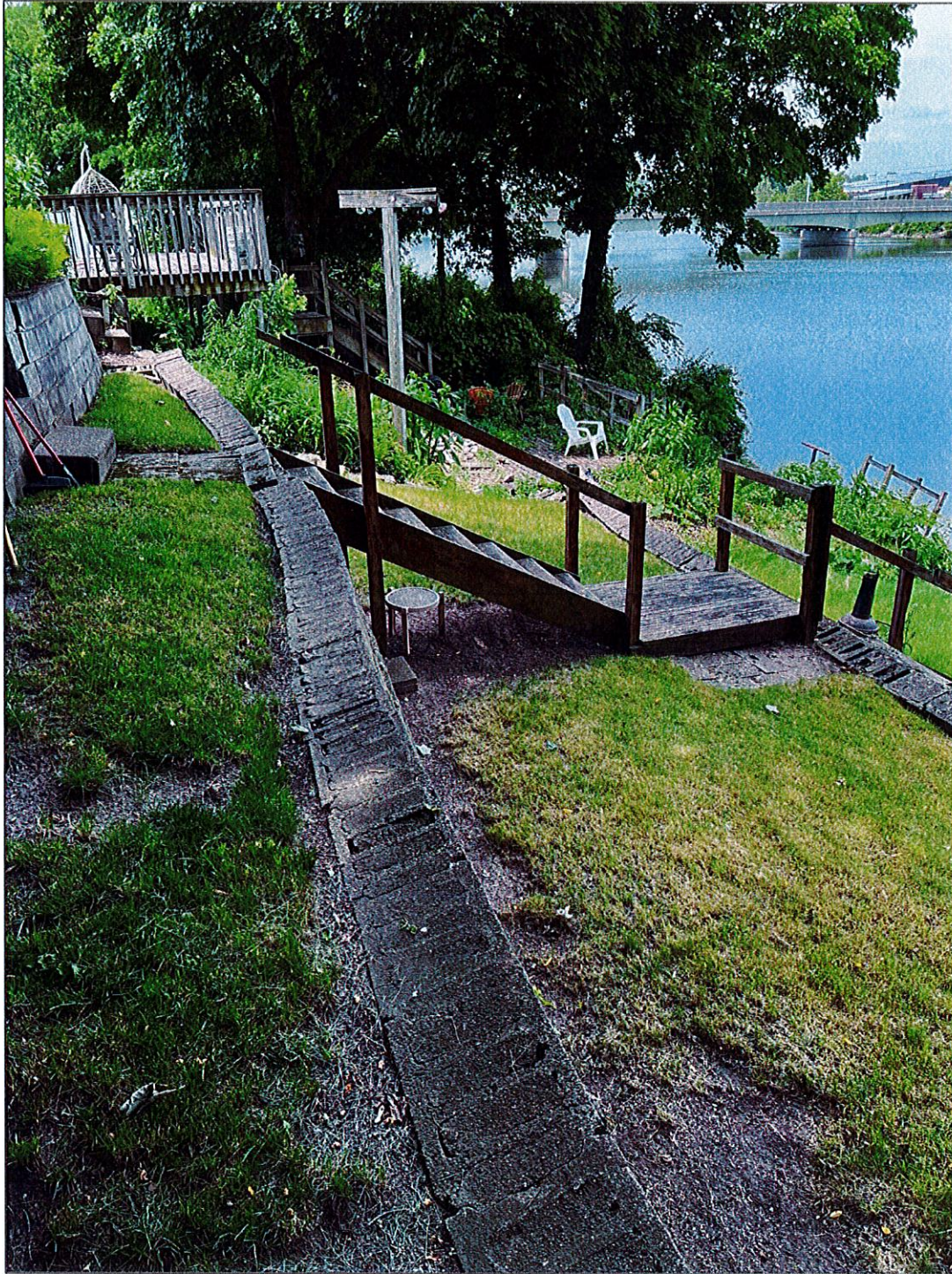
Photograph 3: Existing Embankment Directly West of Proposed Outfall Location
