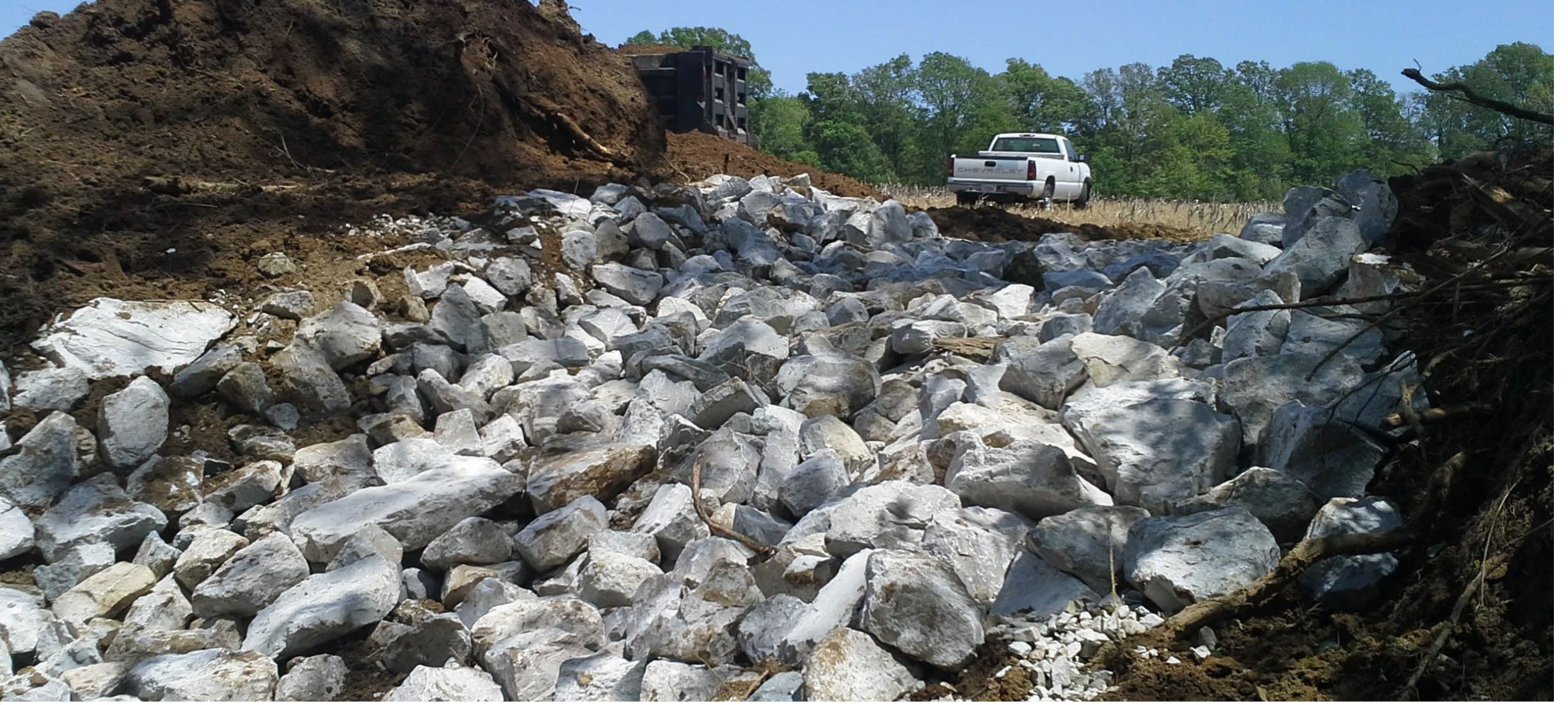
2014- Rock Chute installation at the end of Grassed Waterways
