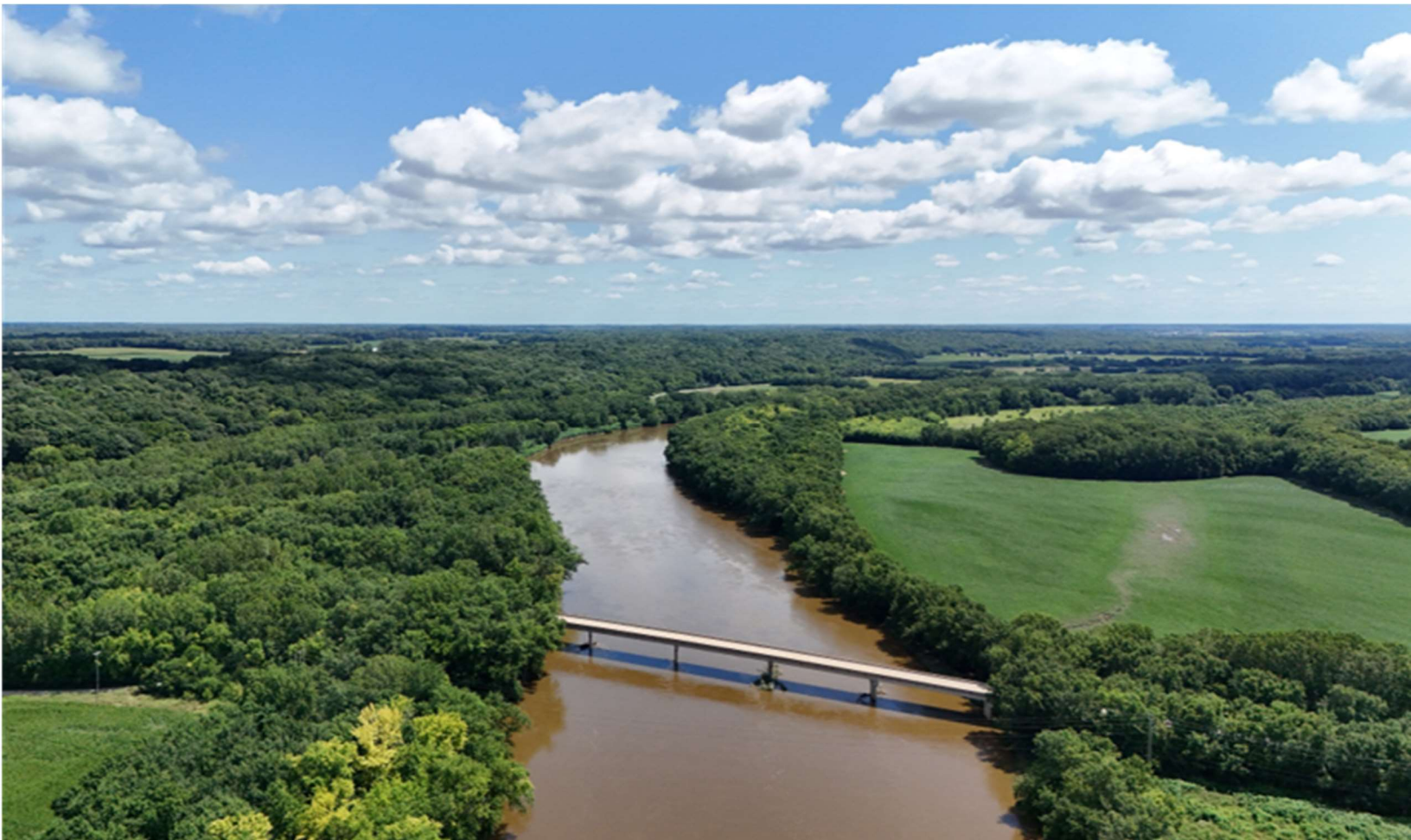
Wabash River – Granville Bridge (IFA, 2024a)
