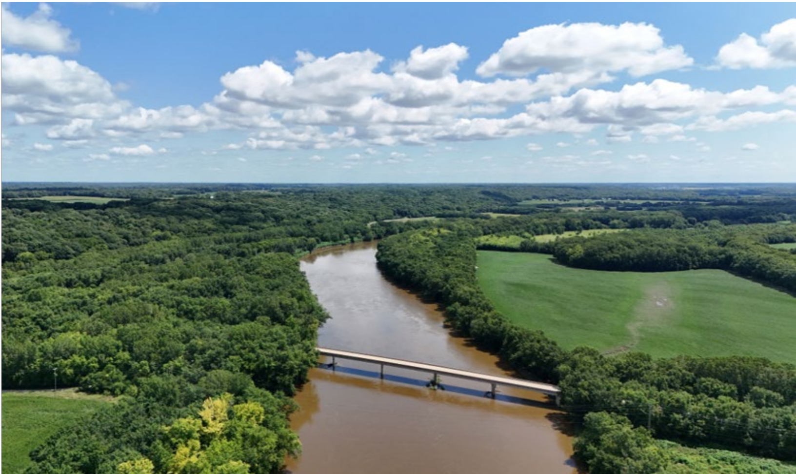
Wabash River – Granville Bridge (IFA, 2024a)
