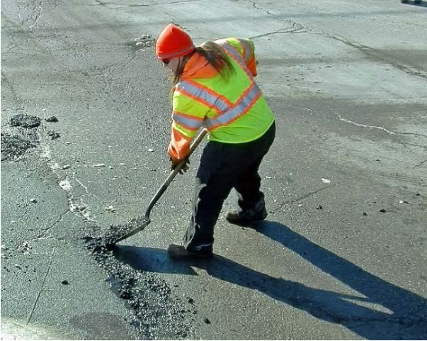
Elkhart Subdistrict Highway Technician Kayla Frick tackles a pothole.
