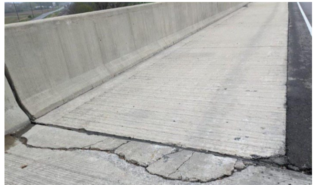
A terminal joint abuts a bridge rail, something that INDOT's Jim Lesh says to avoid in the design process.
