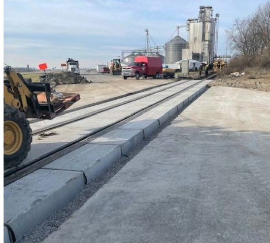
The pavement is removed from State Road 3 (clockwise from top-left photo), new precast concrete sections are delivered, installation of the new crossing begins, and the crossing is nearly complete.
