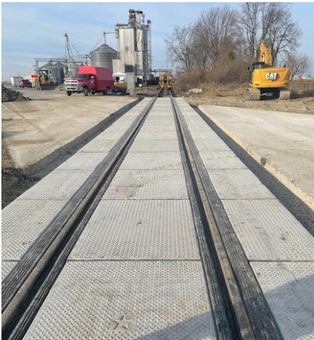
The pavement is removed from State Road 3 (clockwise from top-left photo), new precast concrete sections are delivered, installation of the new crossing begins, and the crossing is nearly complete.
