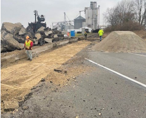
The pavement is removed from State Road 3 (clockwise from top-left photo), new precast concrete sections are delivered, installation of the new crossing begins, and the crossing is nearly complete.
