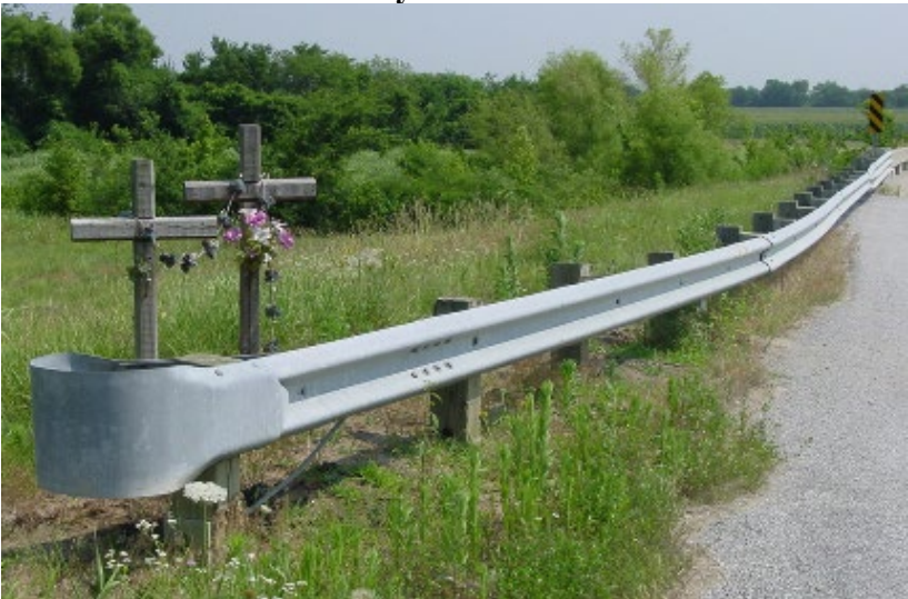
Breakaway Cable Terminal
