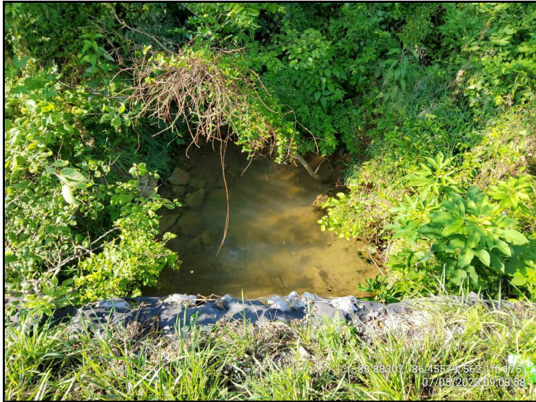
Photograph 37. Taken from SR 58, facing south (downstream) showing the CMP outlet.
