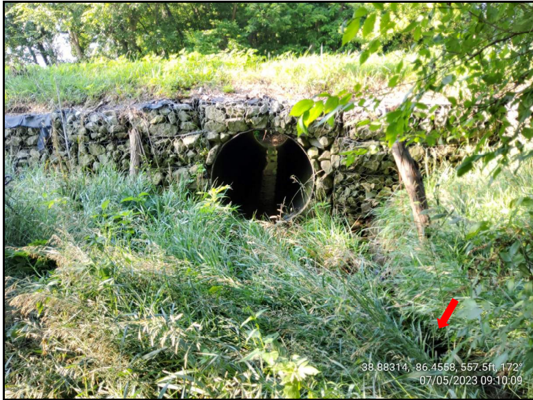
Photograph 41. Taken north of SR 58, facing south showing the CMP inlet and UNT to Leatherwood Creek (red arrow).
