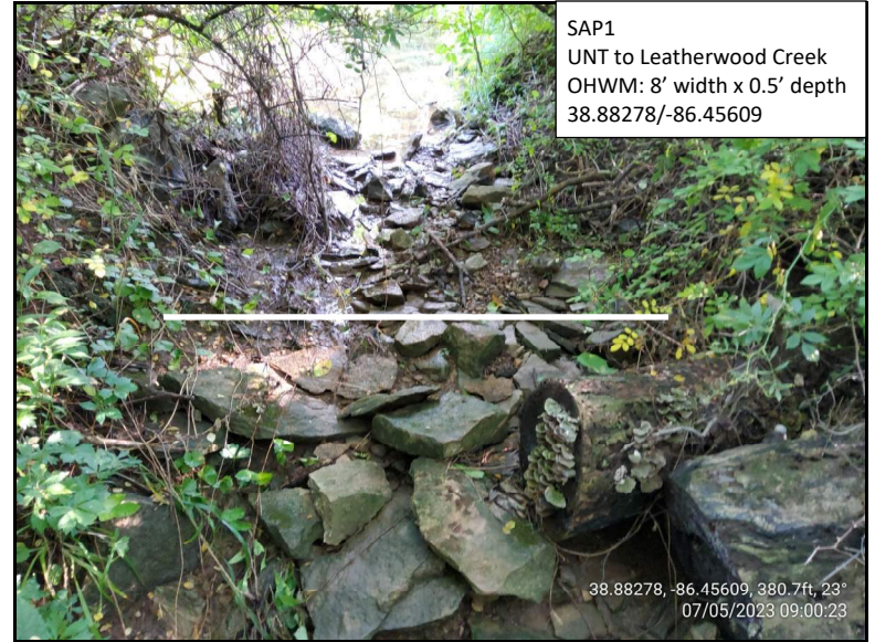
Photograph 38. Taken south of SR 58, facing north-northeast (upstream) in UNT to Leatherwood Creek. White line indicates the OHWM.
