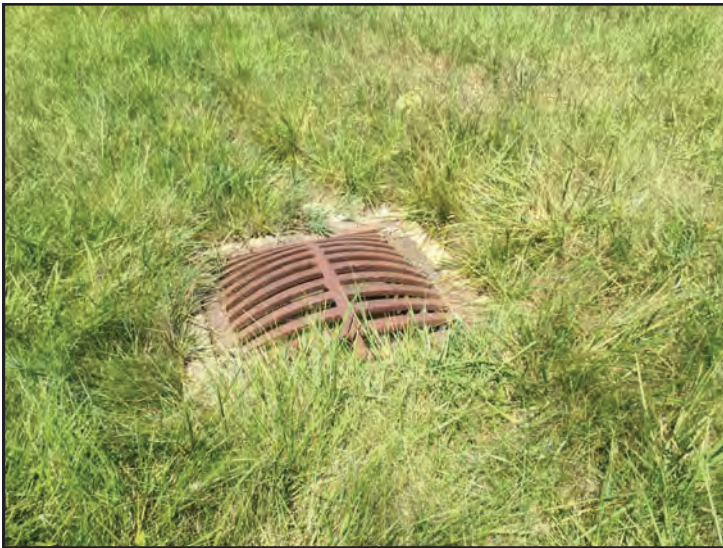
27. View of SD 1 in median of U.S. 41, looking west.
