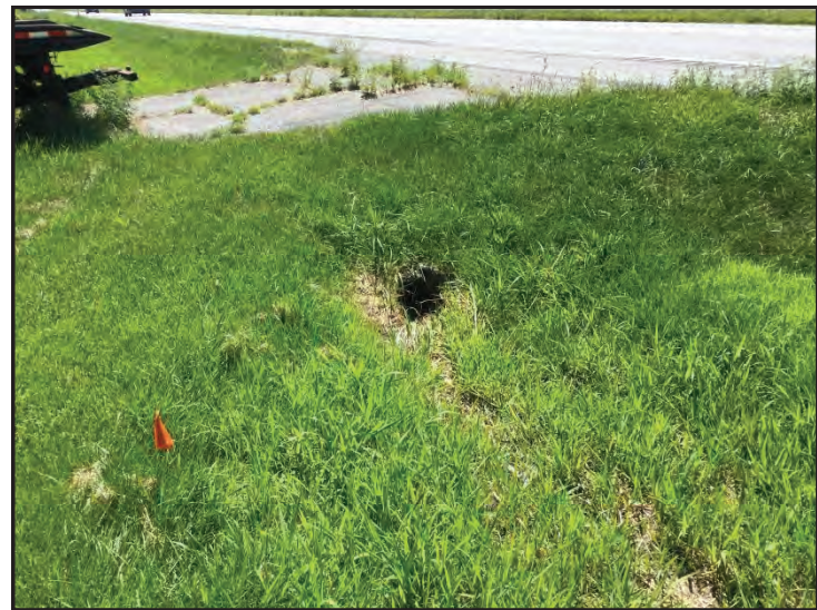
8. View of CV 2 on east side of U.S. 41, looking south.
