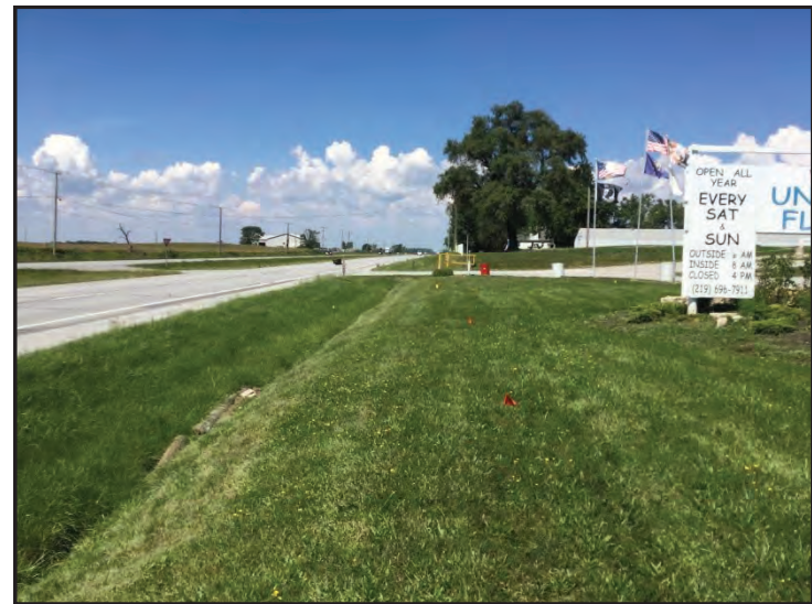
24. View of U.S. 41 ROW and roadside ditch (RSD) 1 on east side of U.S. 41, looking north.
