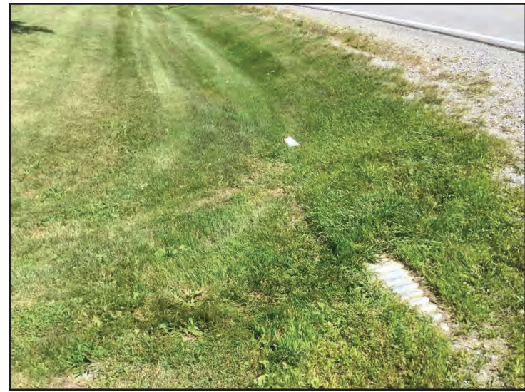
42. View of CV 5 on north side of 151st Ave, looking west.
