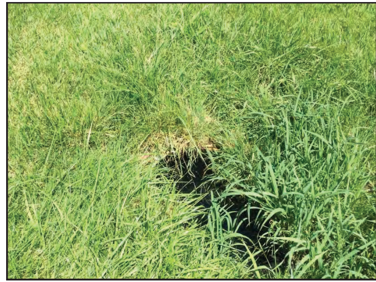
14. View of CV 3 outlet, looking north.
