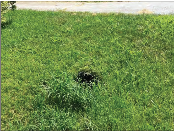
11. View of CV 3, looking south.
