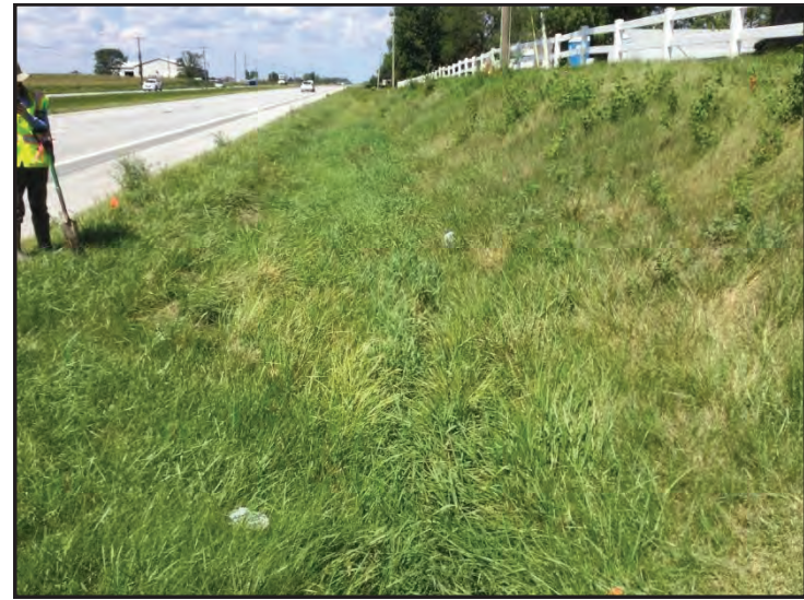
22. View of Wetland A from CV 4, looking north.
