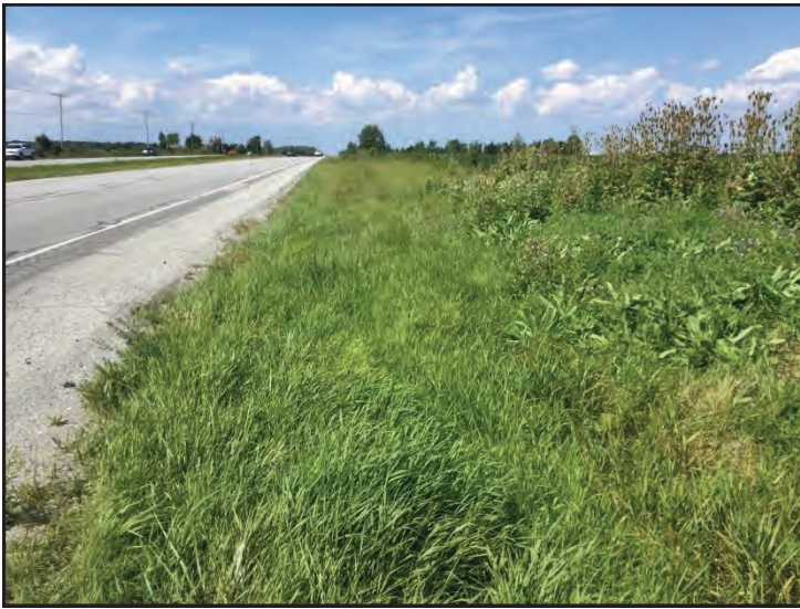
57. View of U.S. 41 ROW from intersection with 151st Ave on east side of U.S. 41, looking north.
