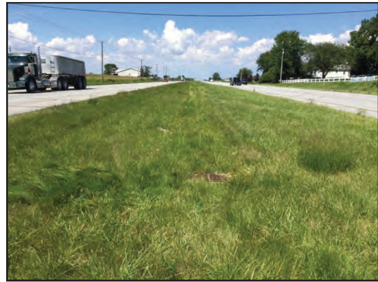
26. View of U.S. 41 median and Storm Drain (SD) 1, looking north.
