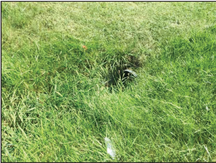
21. View of CV 4 on east side of U.S. 41, looking south.
