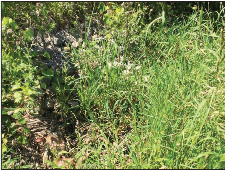
31. View of riprap in Wetland B and surrounding area, looking northwest.
