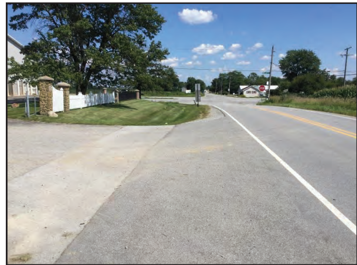
40. View of 151st Ave ROW from north side of 151st Ave and west side of U.S. 41, looking east.
