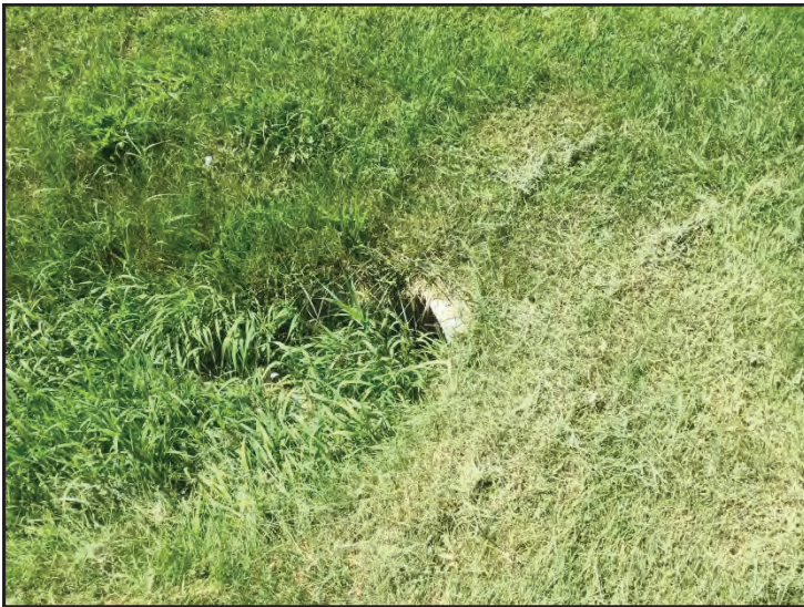
23. View of CV 4, looking north.
