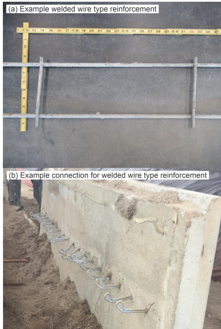
Figure 4. Example of (a) welded wire type MSE wall reinforcement and (b) how it might be connected to facing panels
