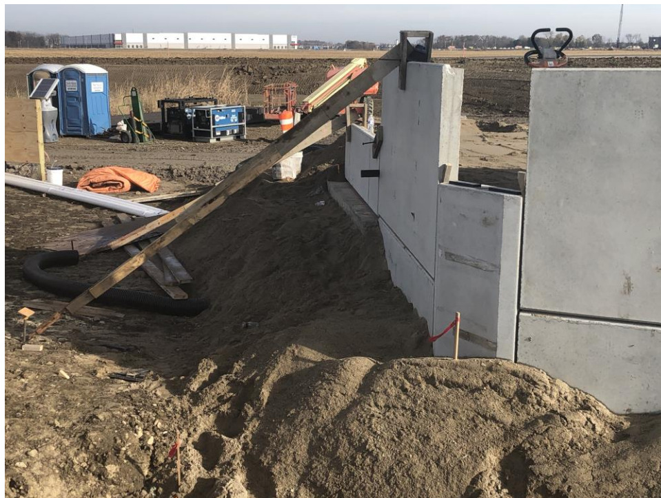
Figure 73. Example bracing of subsequent panel courses
