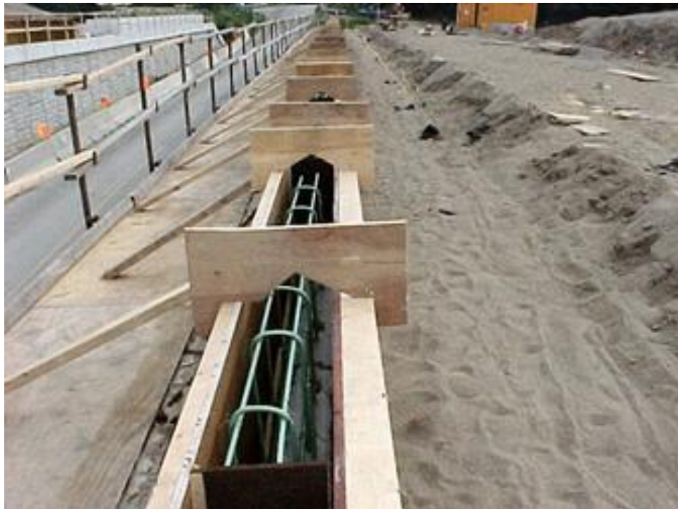
Figure 83. Example of formwork for pouring cast-in-place coping
