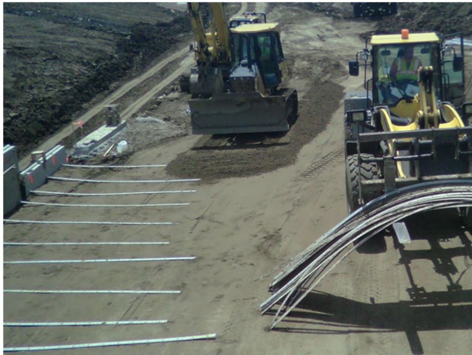
Figure 68. Example of appropriate backfilling over soil reinforcements
