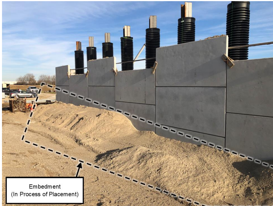
Figure 79. Example wall embedment
