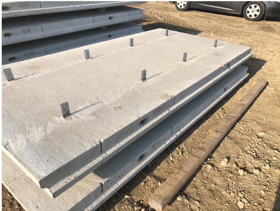
Figure 13. Example MSE wall pre-cast facing panel
