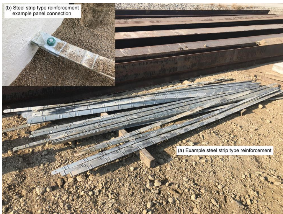
Figure 3. Example of (a) steel strip type MSE reinforcement and (b) how it might be connected to facing panels
