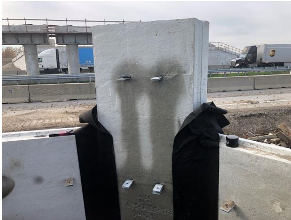
Figure 17. Example corner element installed in an MSE wall
