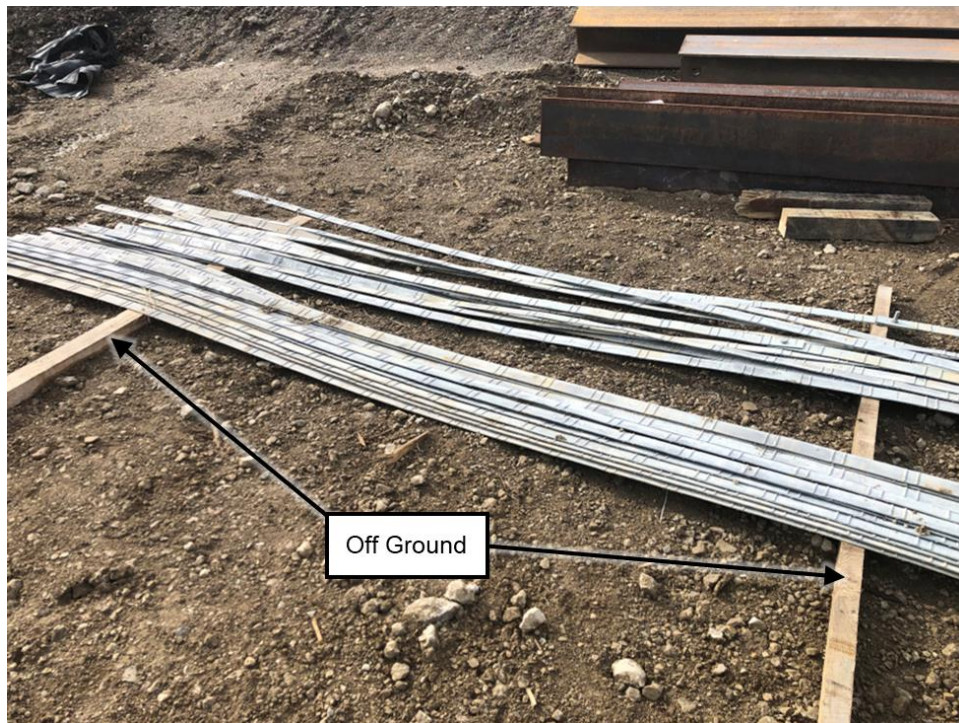
Figure 31. Soil reinforcements stored off of the ground
