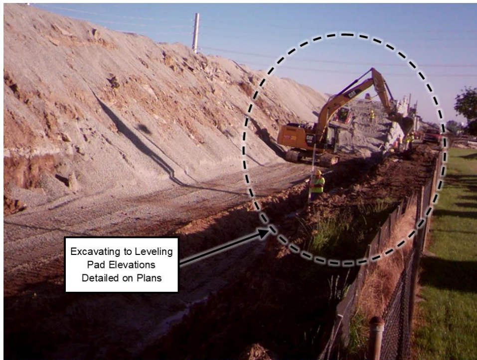
Figure 32. Typical excavation operations for MSE wall foundation preparation
