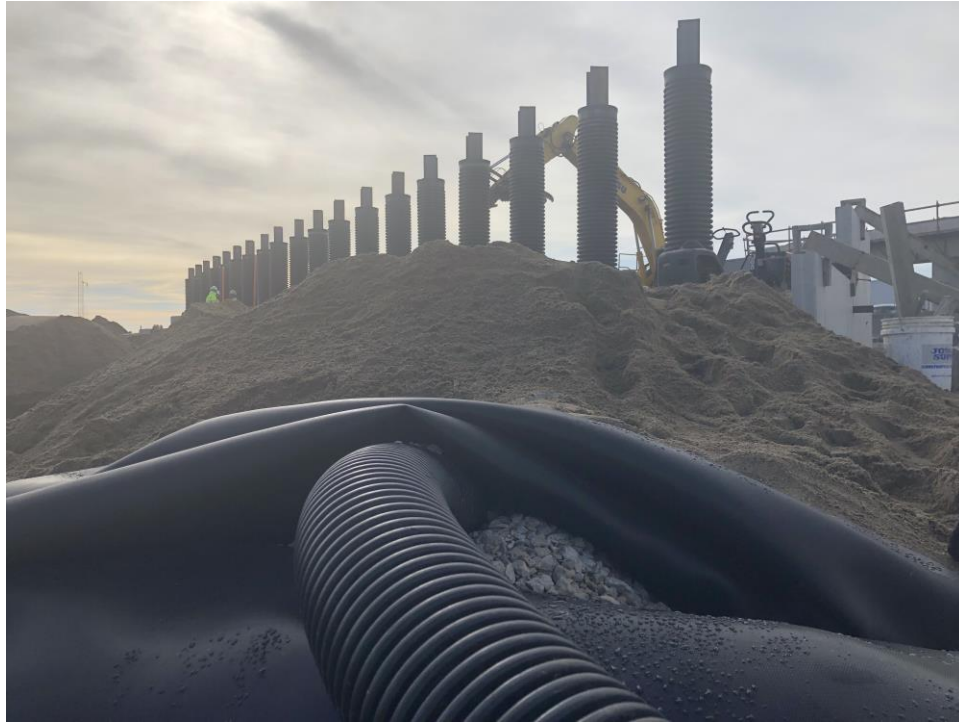
Figure 78. Example internal drainage system
