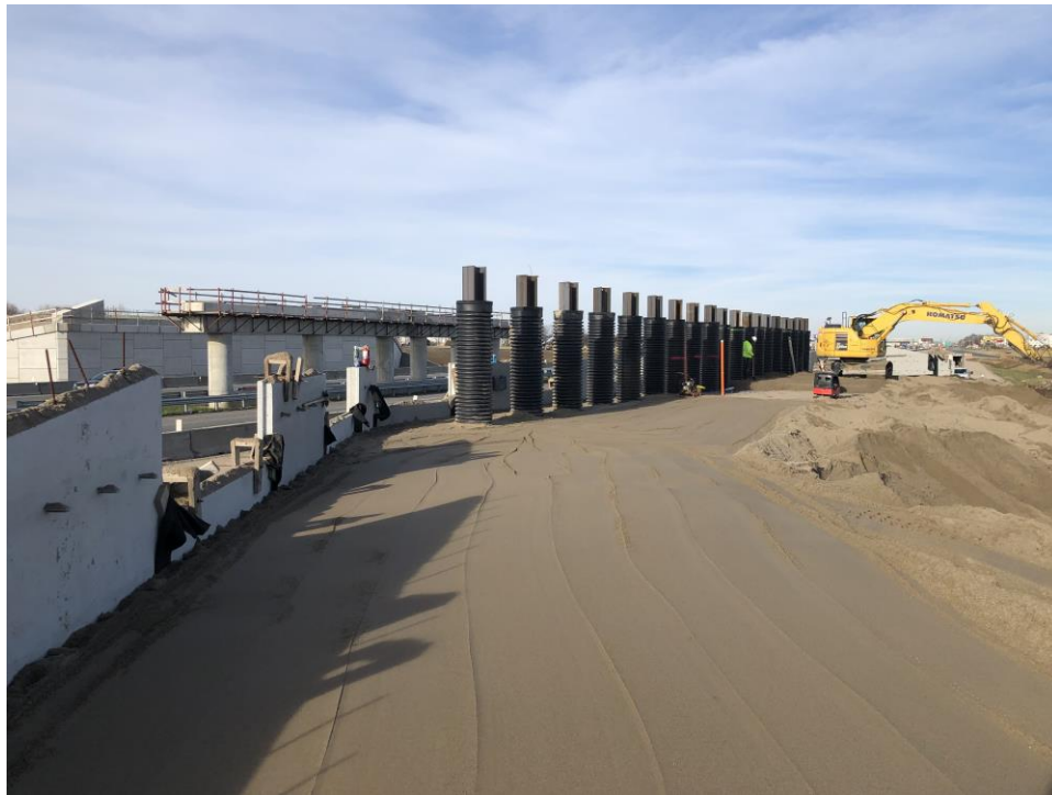
Figure 76. Example structure backfill placement
