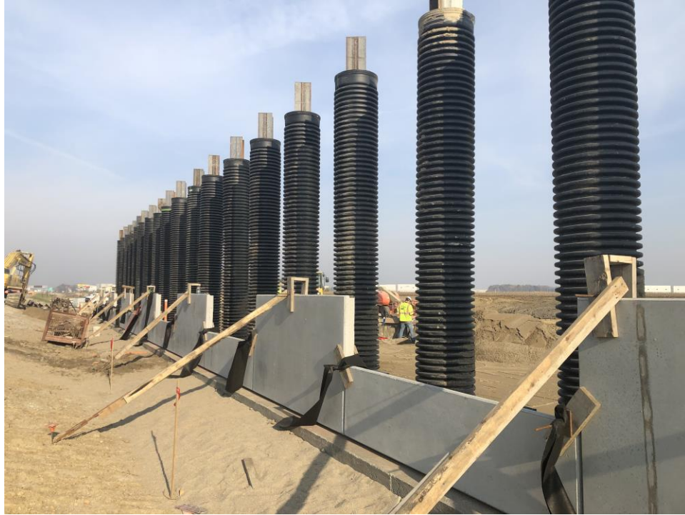
Figure 54. Example of a completed initial course of MSE wall pre-cast panels
