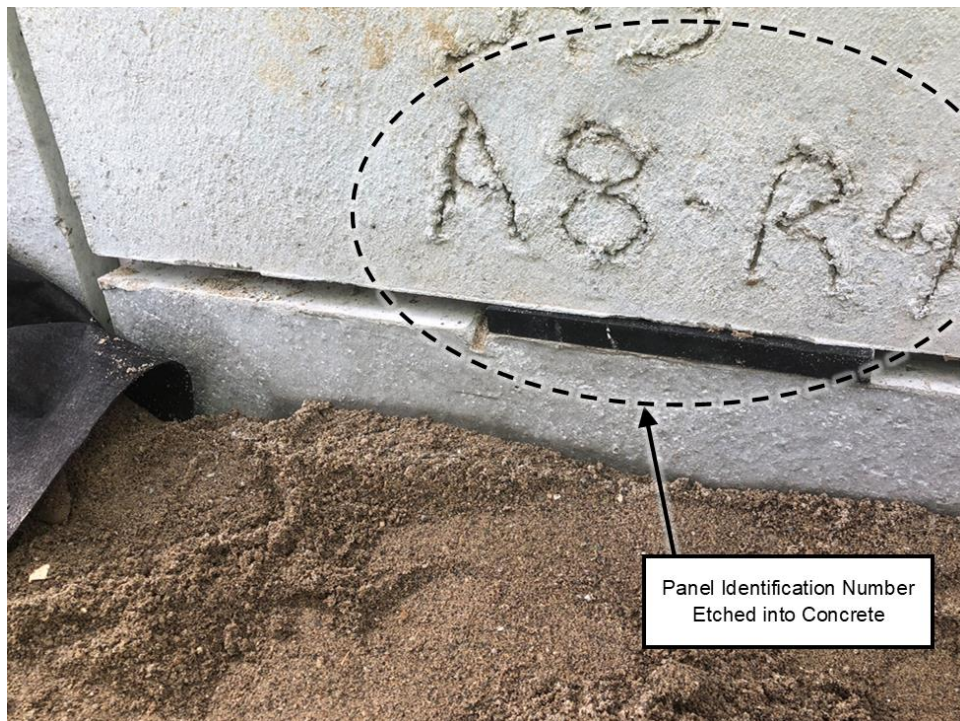
Figure 75. Example panel identification number etched into concrete
