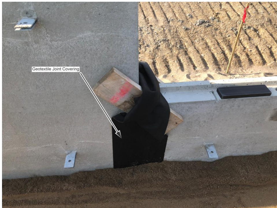
Figure 21. Geotextile joint covering example
