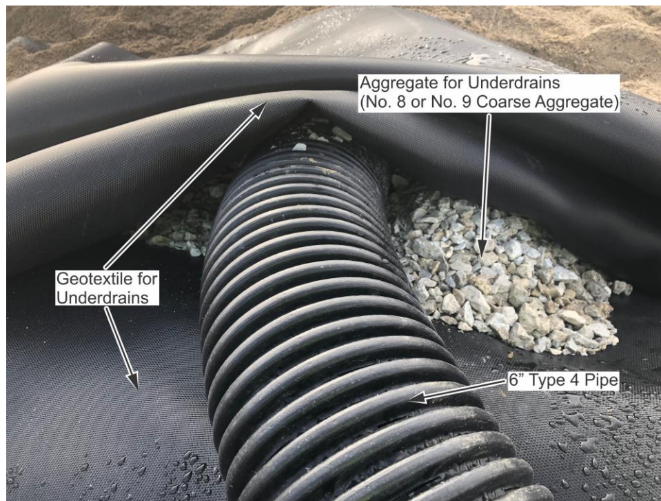
Figure 27. Example MSE wall internal drain
