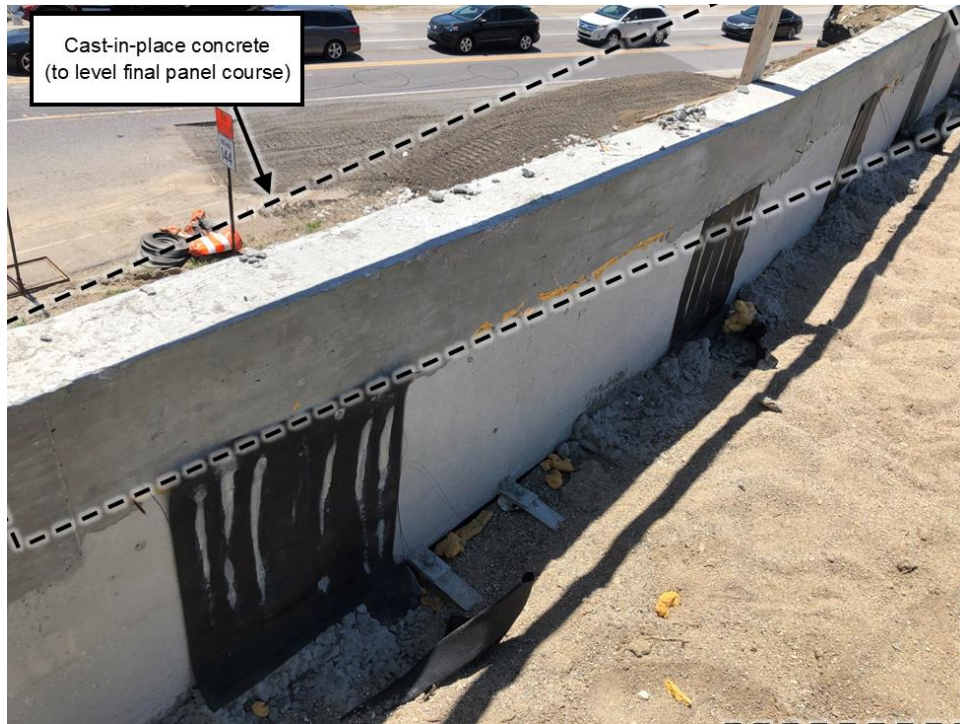
Figure 82. Example of using cast-in-place concrete to flatten and level out the final panel course
