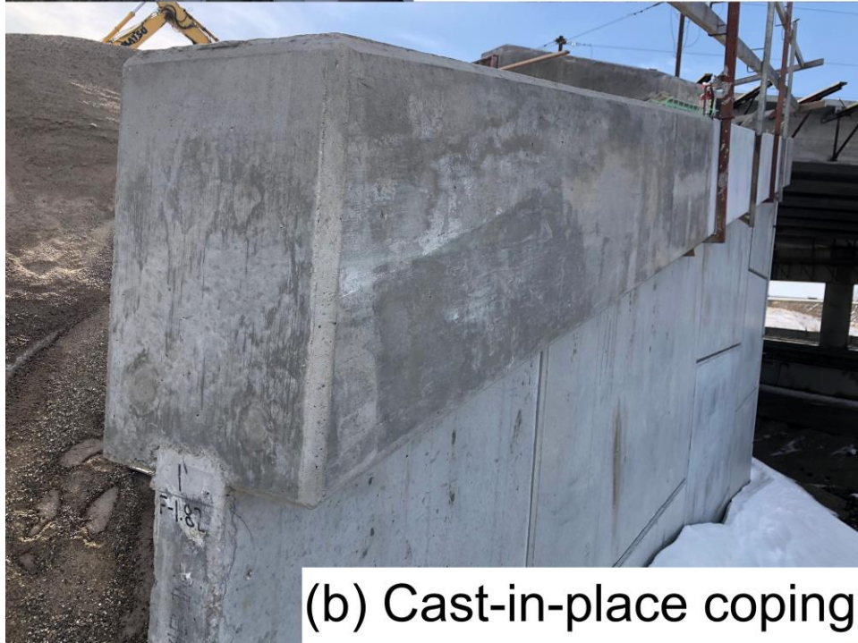
Figure 24. Example MSE wall copings: (a) pre-cast coping and (b) cast-in-place coping
