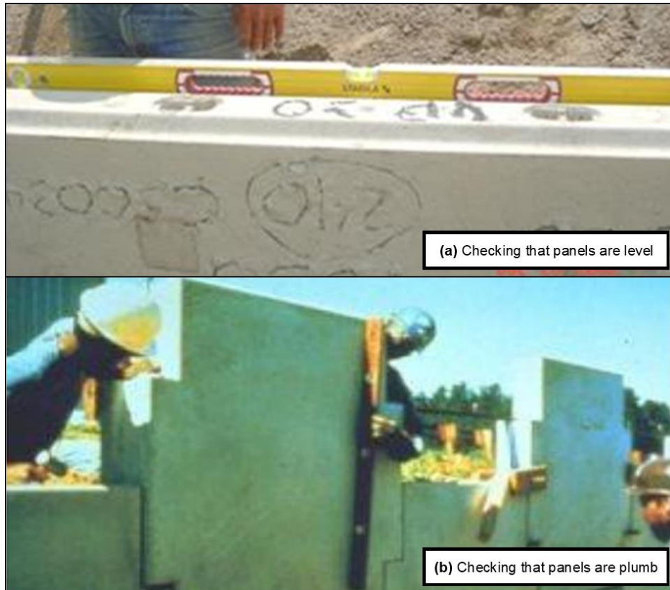
Figure 81. Checking panel alignments
