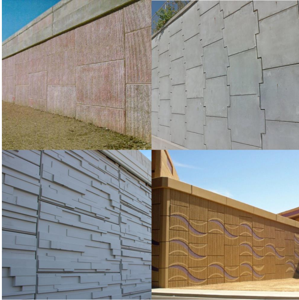
Figure 14. Examples of different MSE wall pre-cast facing panel architectural and textural treatments
