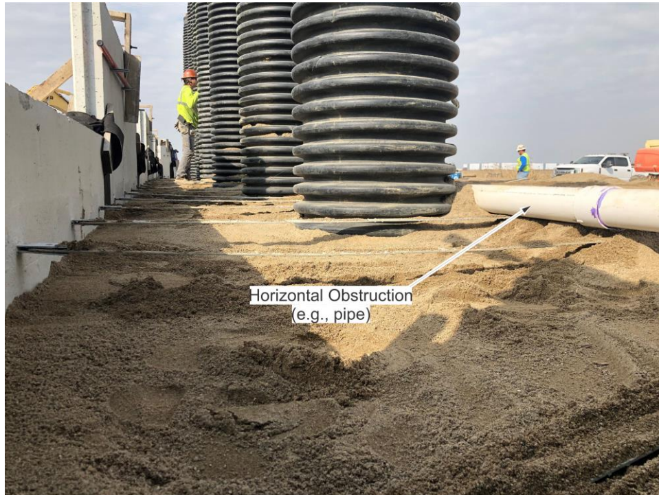
Figure 11. Horizontal obstructions commonly encountered in MSE walls (e.g., pipe)
