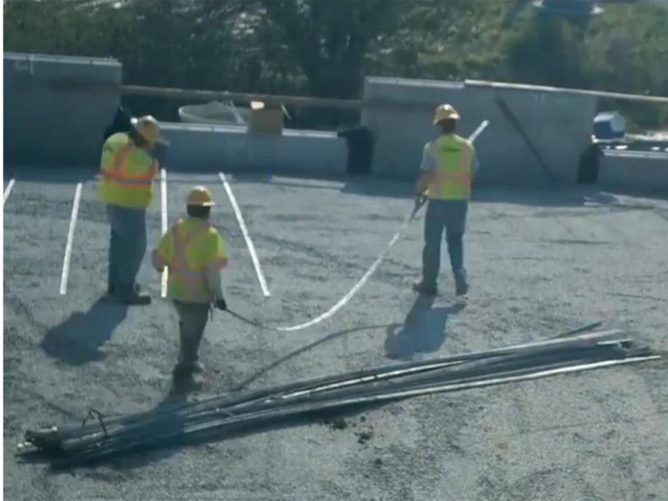
Figure 77. Example soil reinforcement placement
