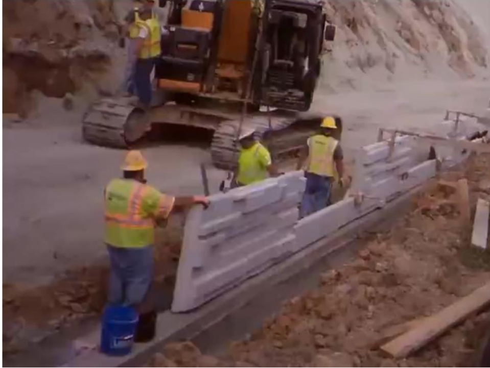
Figure 43. Typical initial course pre-cast panel placement operations
