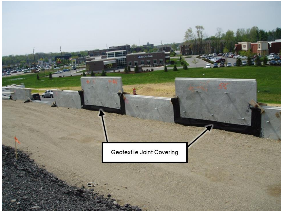
Figure 74. Example of subsequent panel courses joints covered with geotextiles
