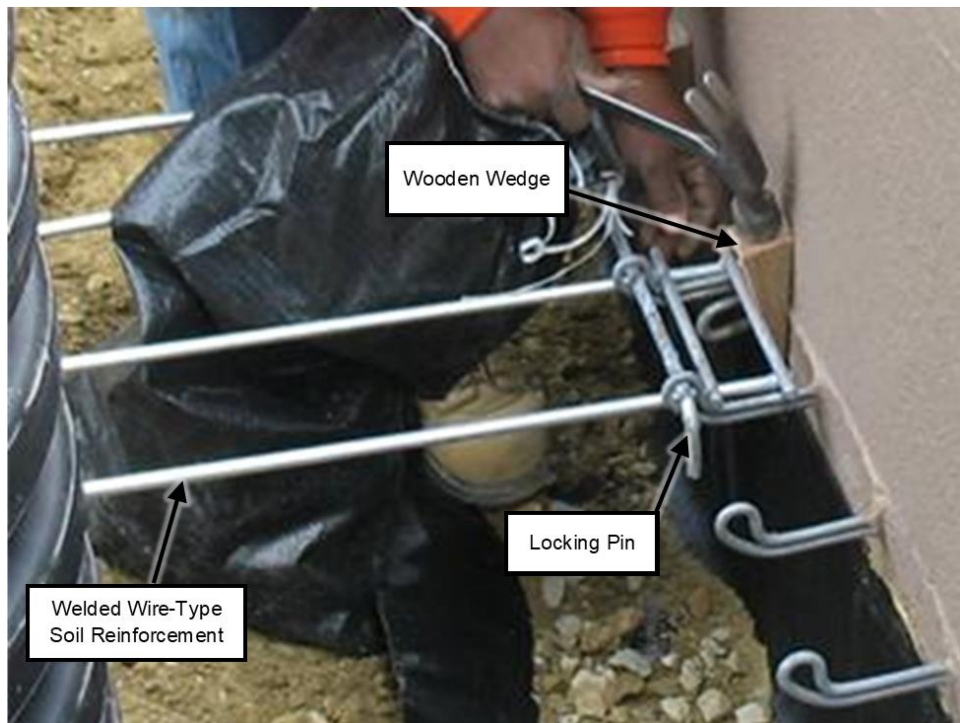
Figure 66. Example connection for weld-wire-type soil reinforcement
