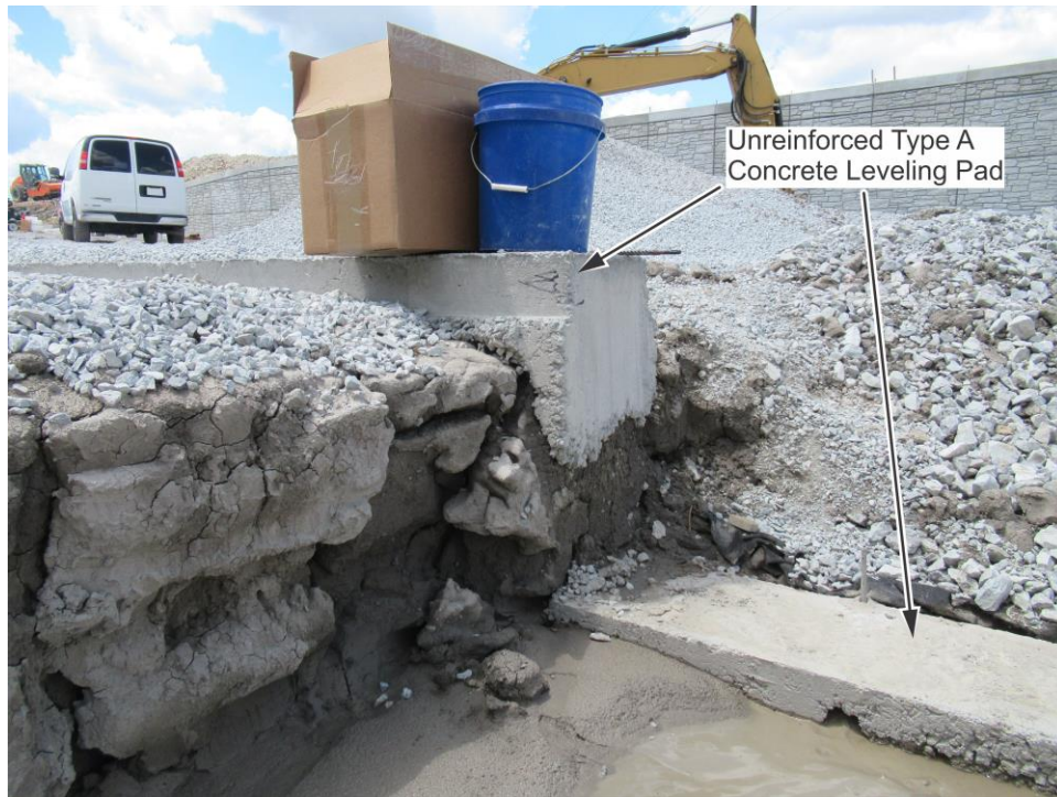
Figure 23. Example MSE wall leveling pad
