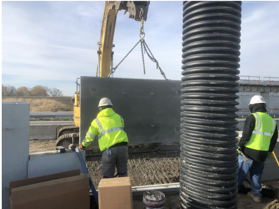
Figure 71. Example placement of subsequent panel course
