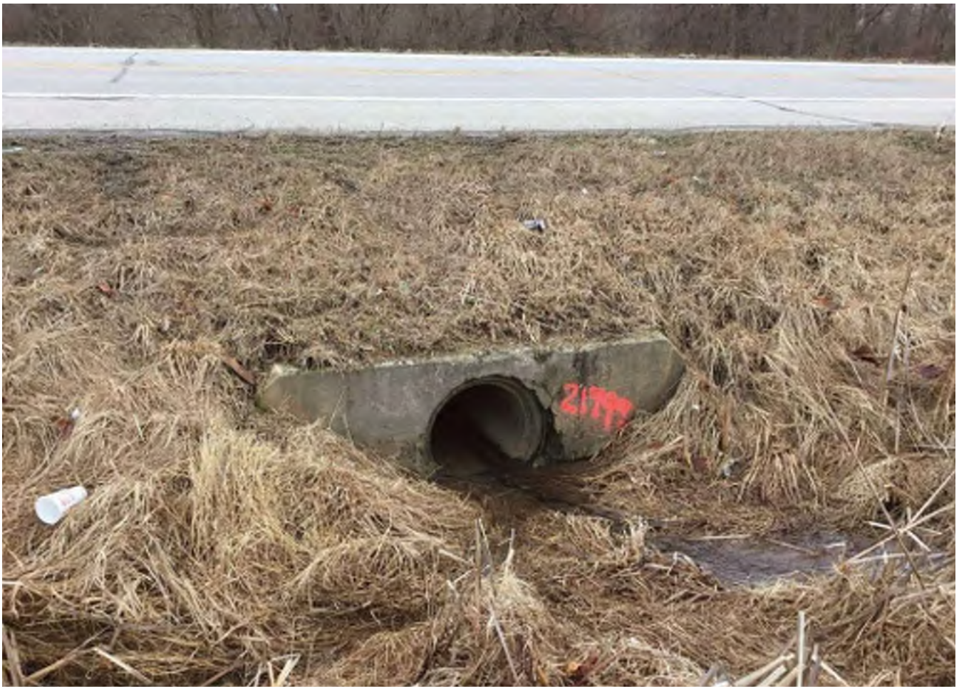
9 Looking south at “Non-contributing” concrete culvert with concrete headwall along SR 46.
