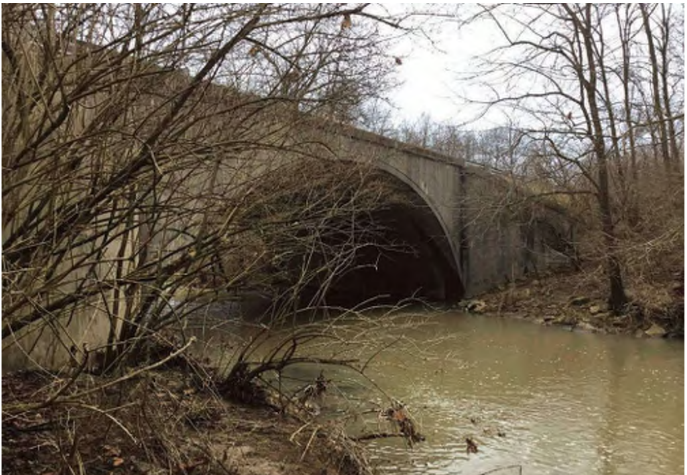
14 Looking northeast at “Contributing” reinforced concrete arched bridge [Bridge No. 046-16-00945 / NBI No. 17400] (RQAW #3) carrying SR 46 (Main Street) over Muddy Fork Sand Creek.
