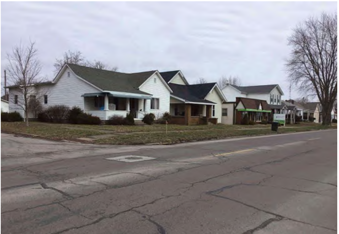
89 Looking northeast at “Non-contributing” houses and buildings along Main Street from the east boundary of the recommended National Register-eligible Greensburg Eastside Residential Historic District.
