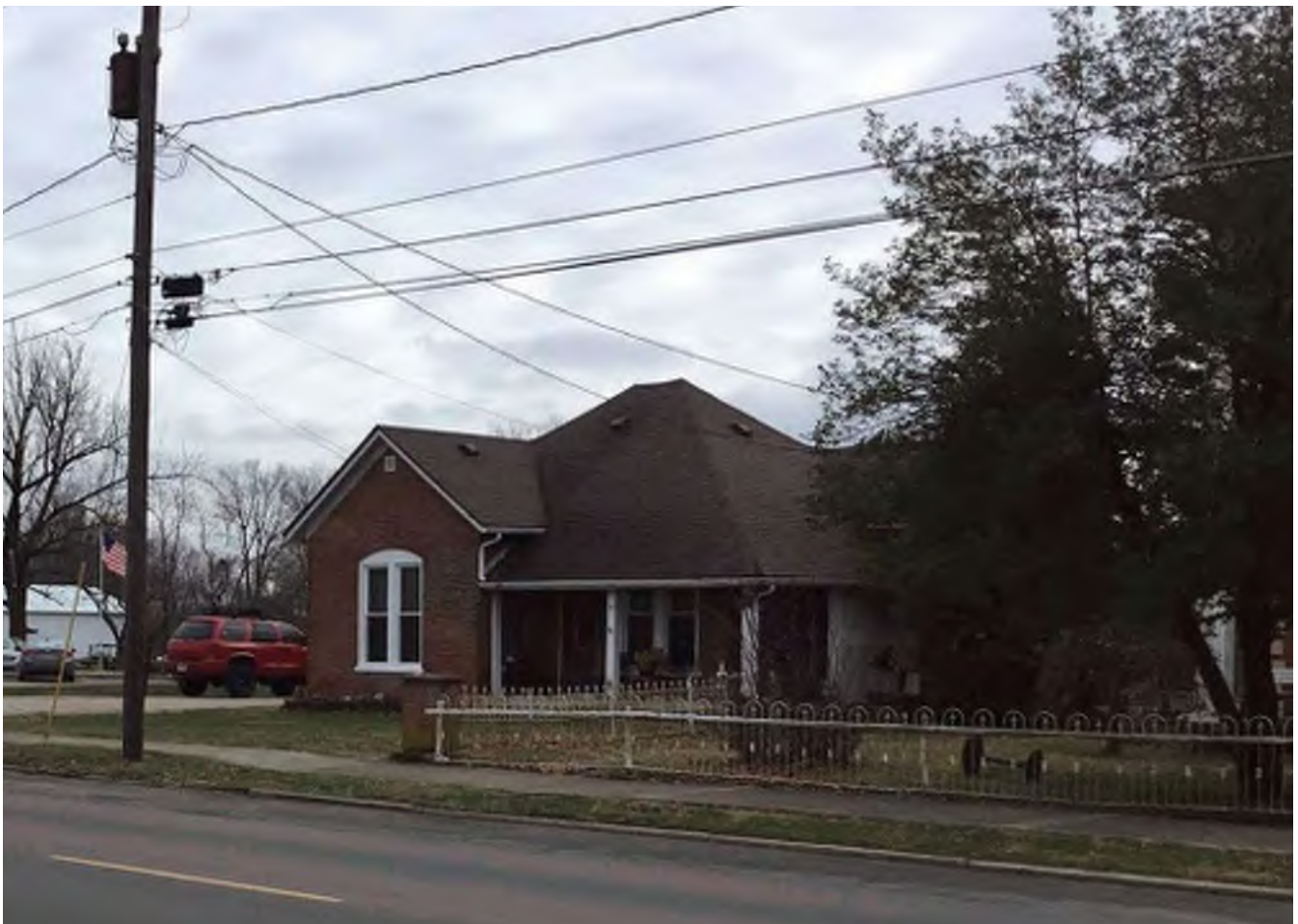
94 Looking southeast at “Contributing” house (RQAW # 12) at 827 E. Main Street.
