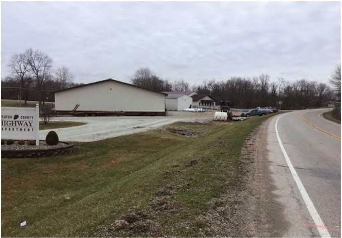
109 Looking southeast at c. 1940 “Non-contributing” office and c. 2000 County Highway buildings at the east end of the APE.
