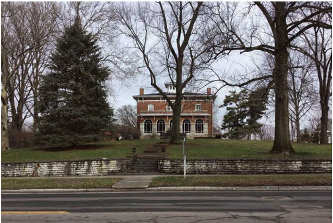
70 Looking north at “Outstanding” Wilderwood House (IHSSI #031-252-23029) at 446 E. Main Street within the recommended National Register-eligible Greensburg Eastside Residential Historic District. Note limestone curbs and limestone retaining wall.
