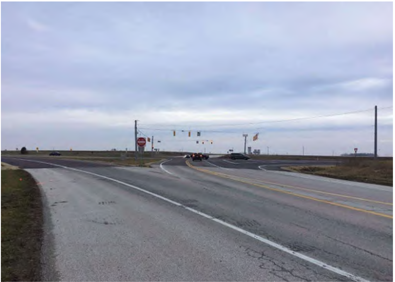
1 Looking northwest towards the western edge of the APE and SR 46/SR 3 intersection.
