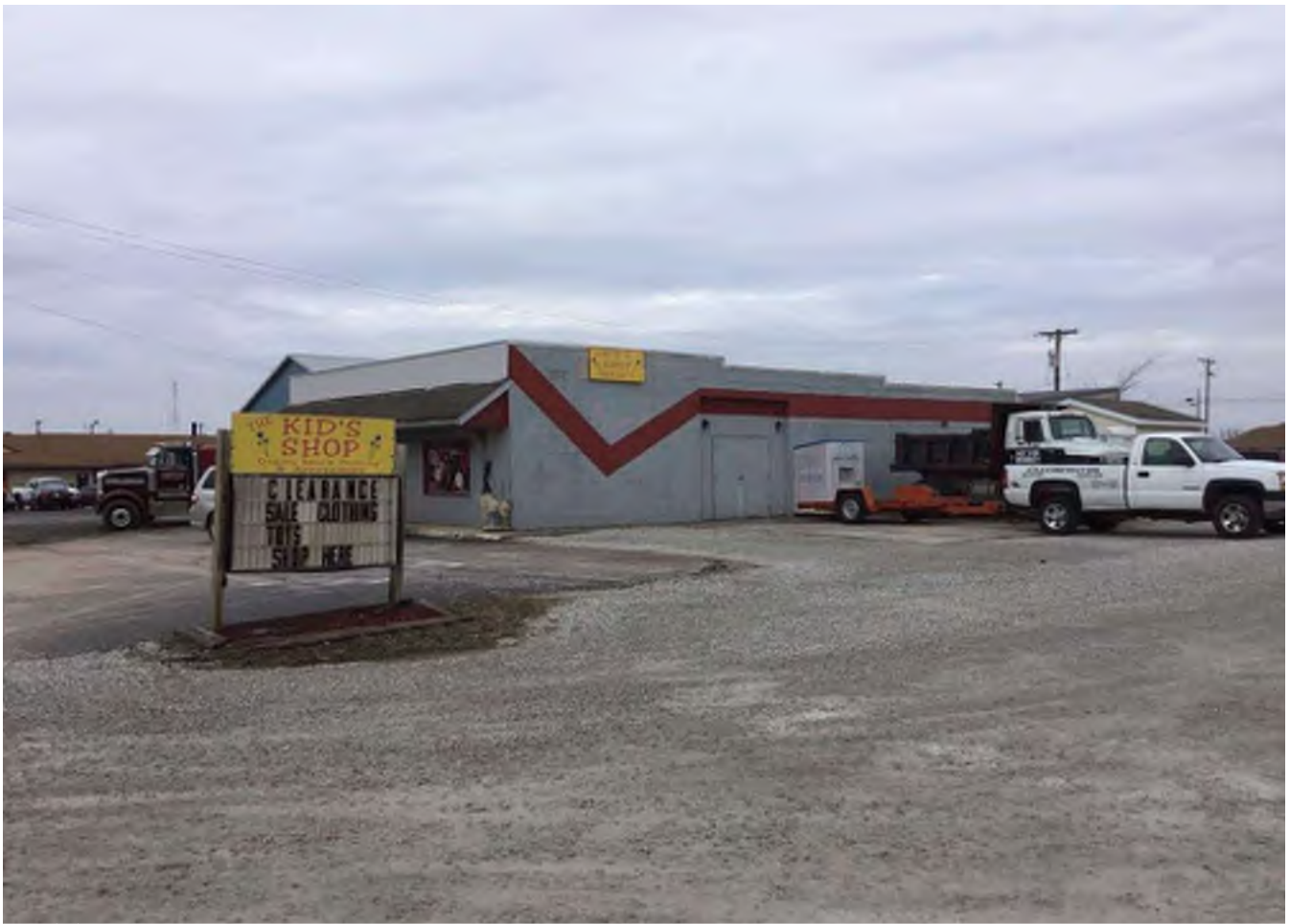
25 Looking northwest at “Non-contributing” c. 1950 CMU block industrial building at 1206 W. Main Street (SR 46).
