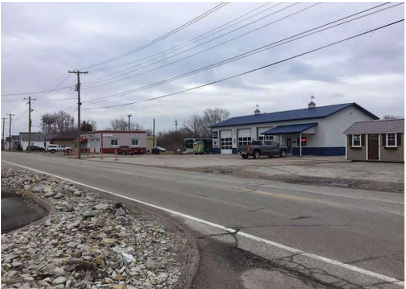
30 Looking southeast at “Non-contributing” buildings along Main Street.
