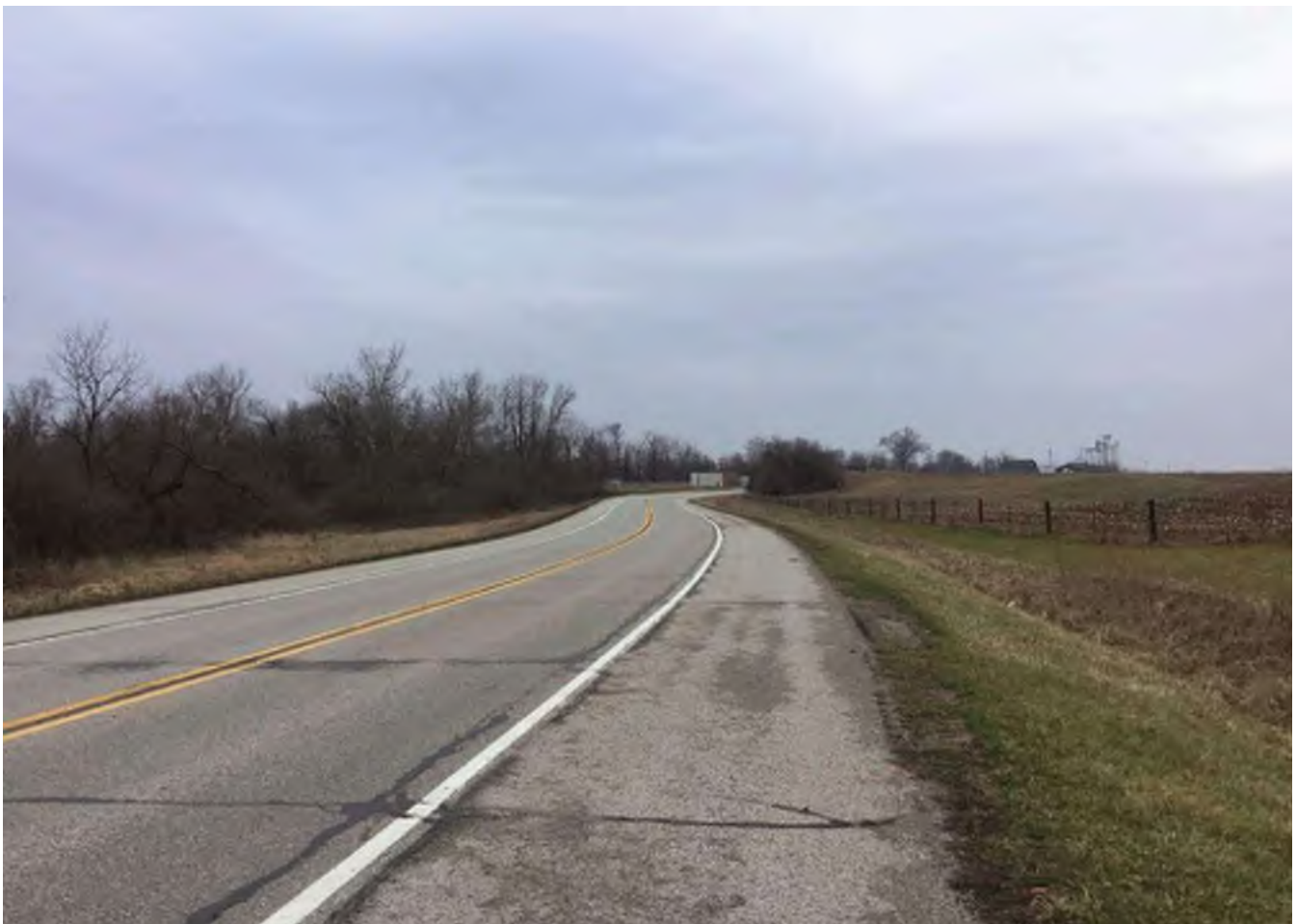
10 Looking west along SR 46.
