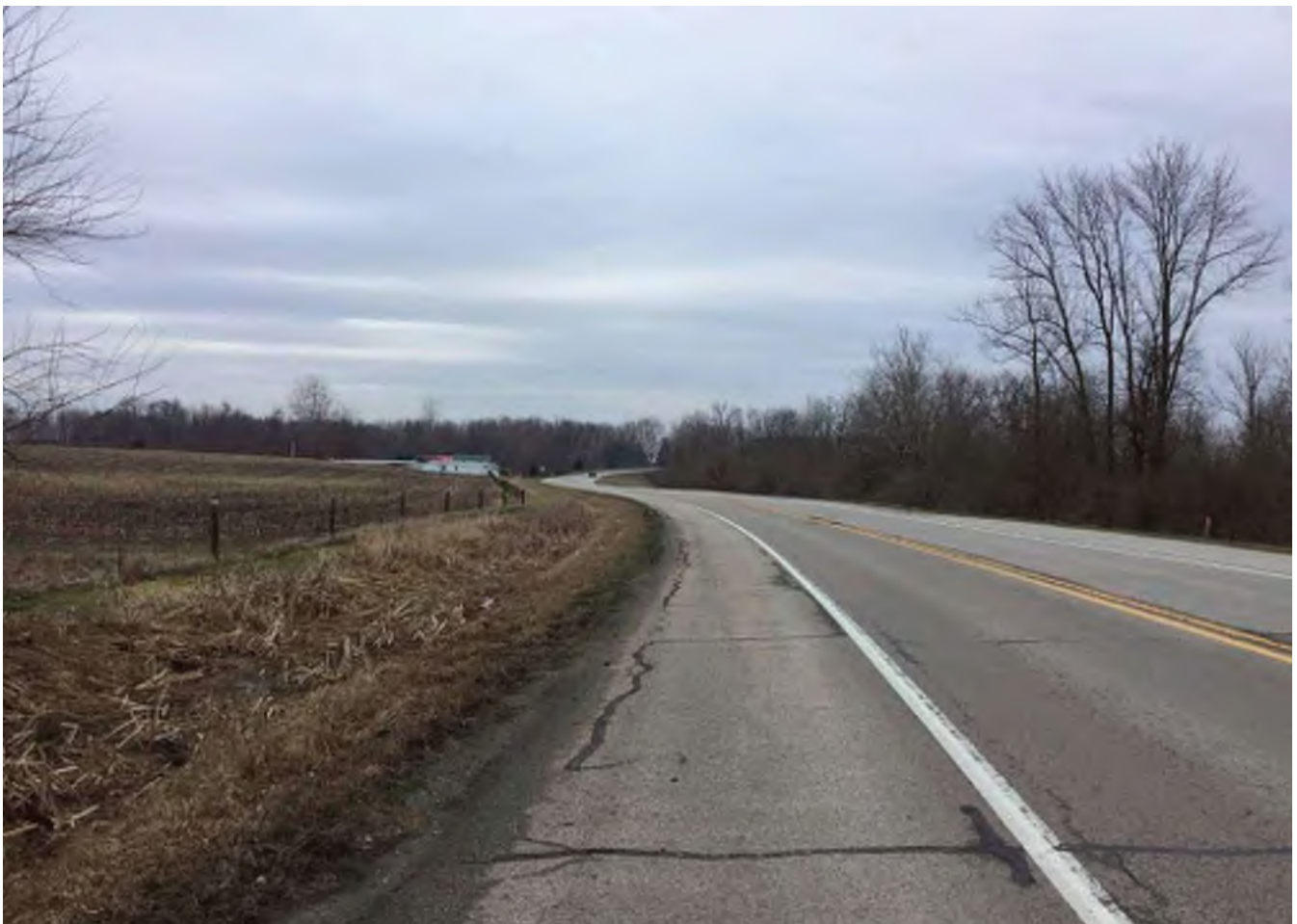
8 Looking east along SR 46.
