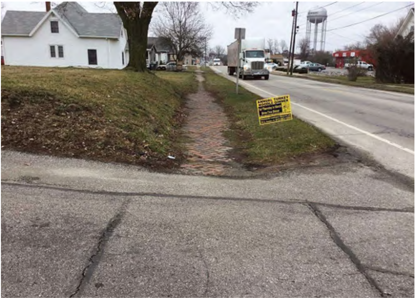
35 Looking east at section of brick sidewalk north of Main Street, east of West Street.
