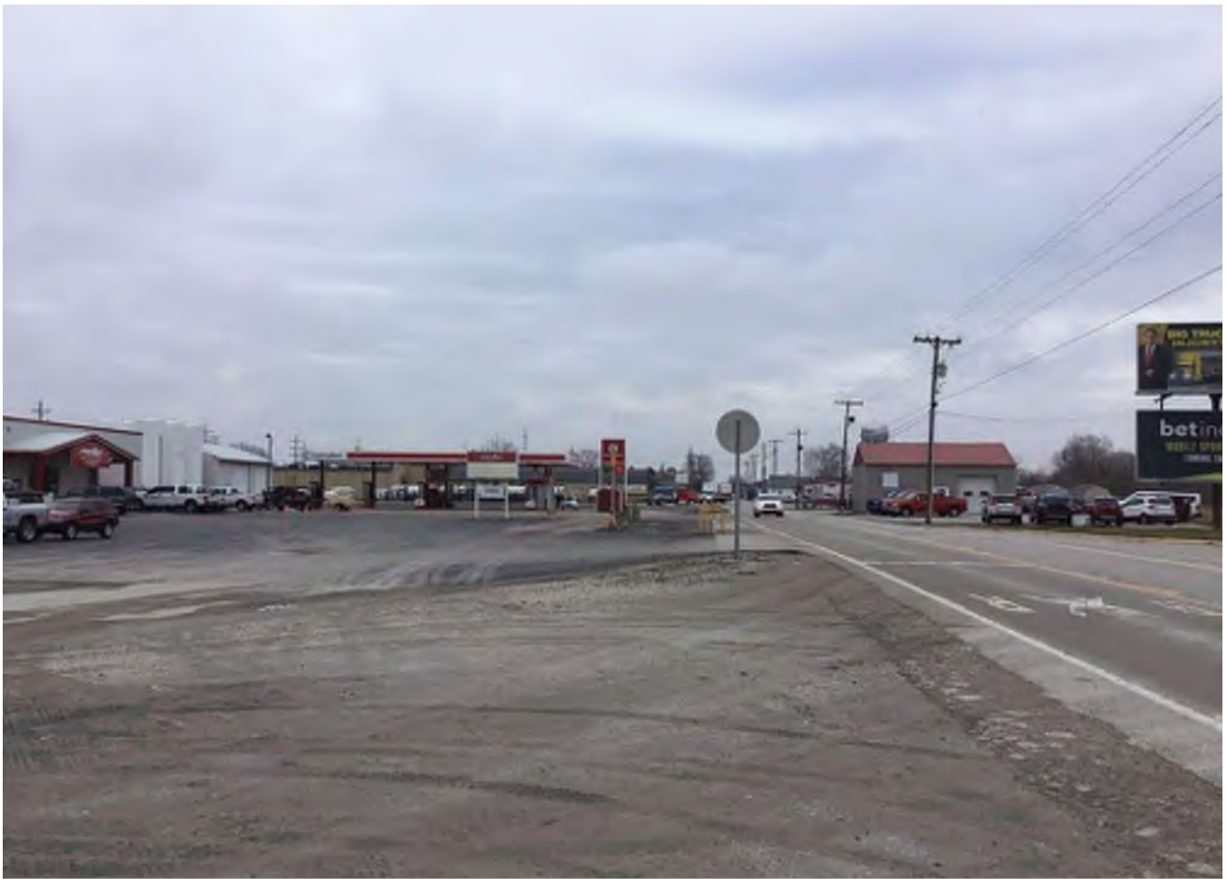
29 Looking east at “Non-contributing” buildings along Main Street.
