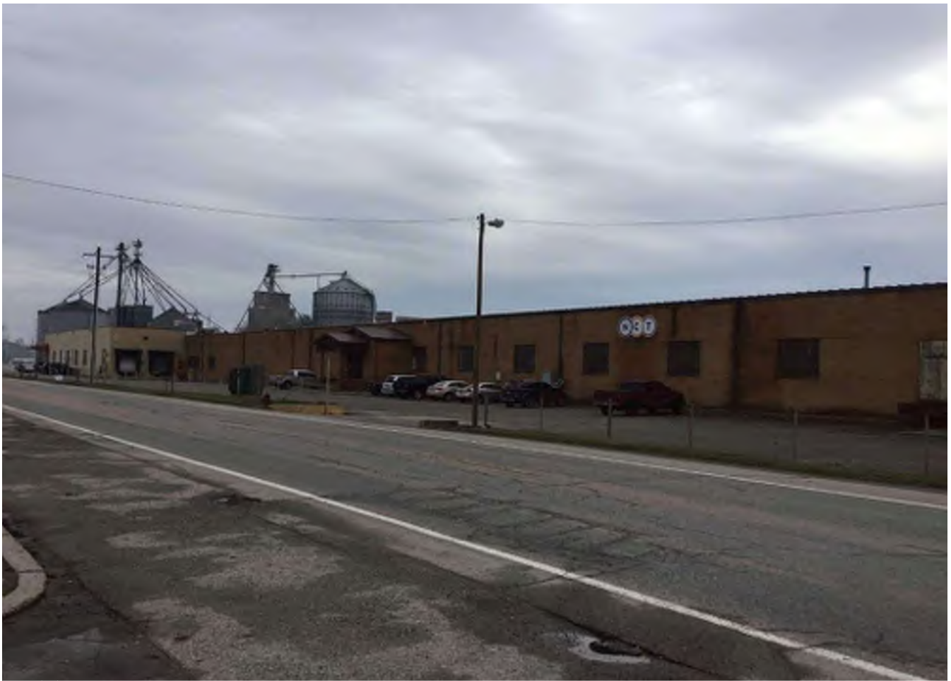
23 Looking south at "Contributing" c. 1958, 1964, and 1971 industrial buildings (RQAW # 6) at 1115 W. Main Street (SR 46).
