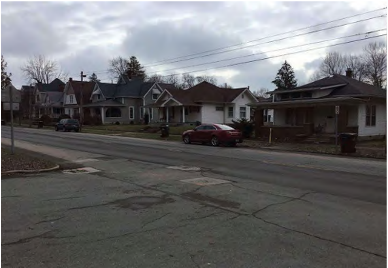
73 Looking southeast across the Main Street / Lathrop Street intersection at “Contributing” and “Non-contributing” houses within the recommended National Register-eligible Greensburg Eastside Residential Historic District.
