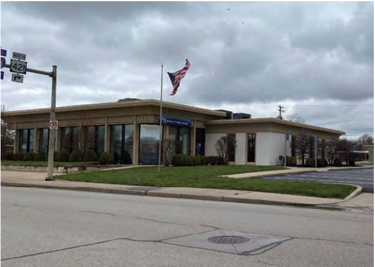
6 Looking northwest at the c. 1973 "Contributing" bank (RQAW #8) within the original APE.
