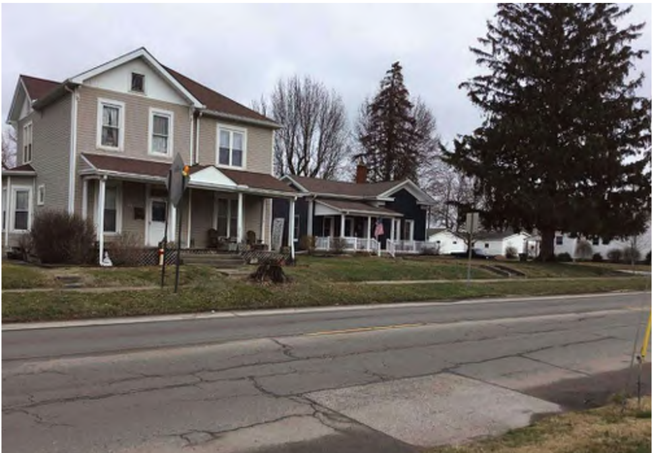
86 Looking northeast at “Contributing” houses at 722 and 730 E. Main Street within the recommended National Register-eligible Greensburg Eastside Residential Historic District.
