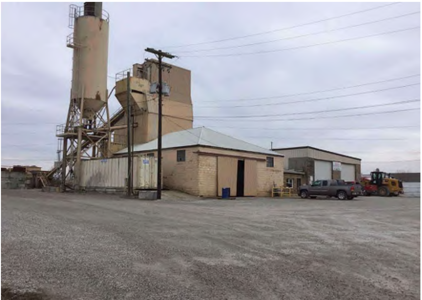
24 Looking south at "Non-contributing" c. 1950 CMU block industrial building at 1100 W. Main Street (SR 46).
