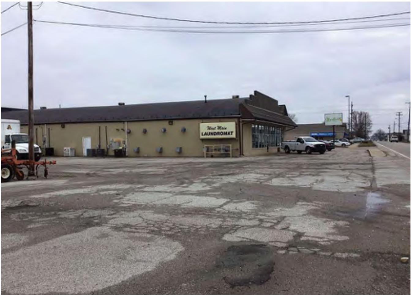
31 Looking northeast at c.1955 "Non-contributing" laundromat building at 736 W. Main Street with altered storefront.
