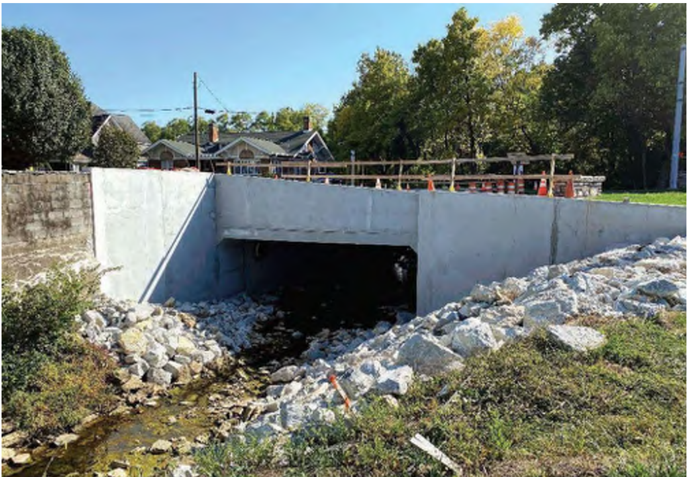
62. October 2020 photo looking southeast at the new concrete bridge within the Greensburg Eastside Residential Historic District. The bridge original stone arch bridge was replaced in the summer of 2020.
