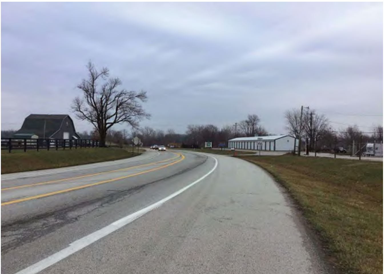
2 Looking east along SR 46 from the west extent of the project.
