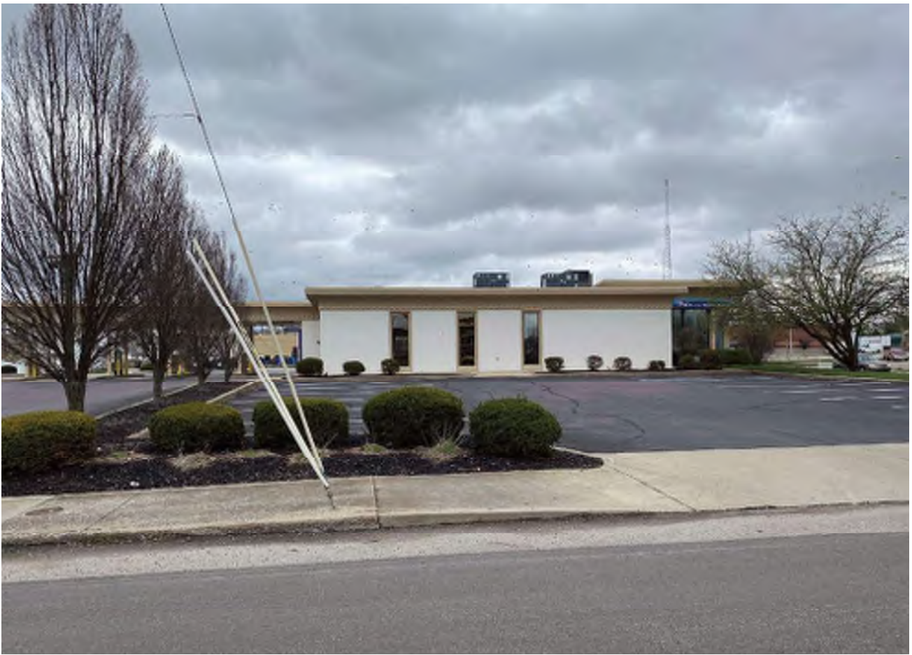
5 Looking east at the c. 1973 "Contributing" bank (RQAW #8) within the original APE.
