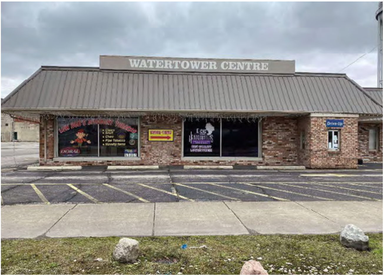
9 Looking south at “Non-contributing” c. 1955 commercial building at 325 W. Main Street.
