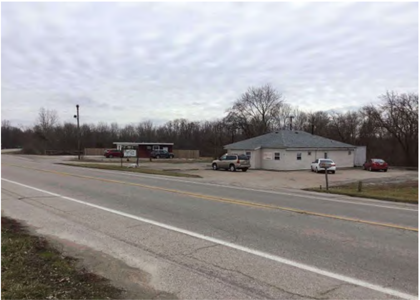
107 Looking southeast at c. 1960 “Non-contributing” commercial buildings along Main Street.
