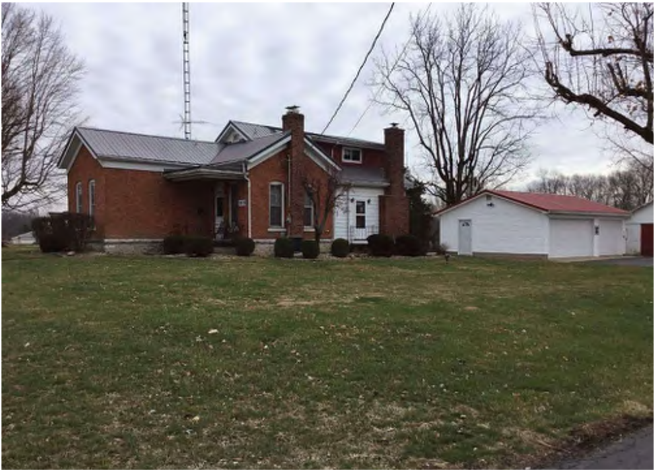
101 Looking southeast at “Contributing” house (IHSSI # 031-252-24066) at 1015 E. Main Street with many alterations.
