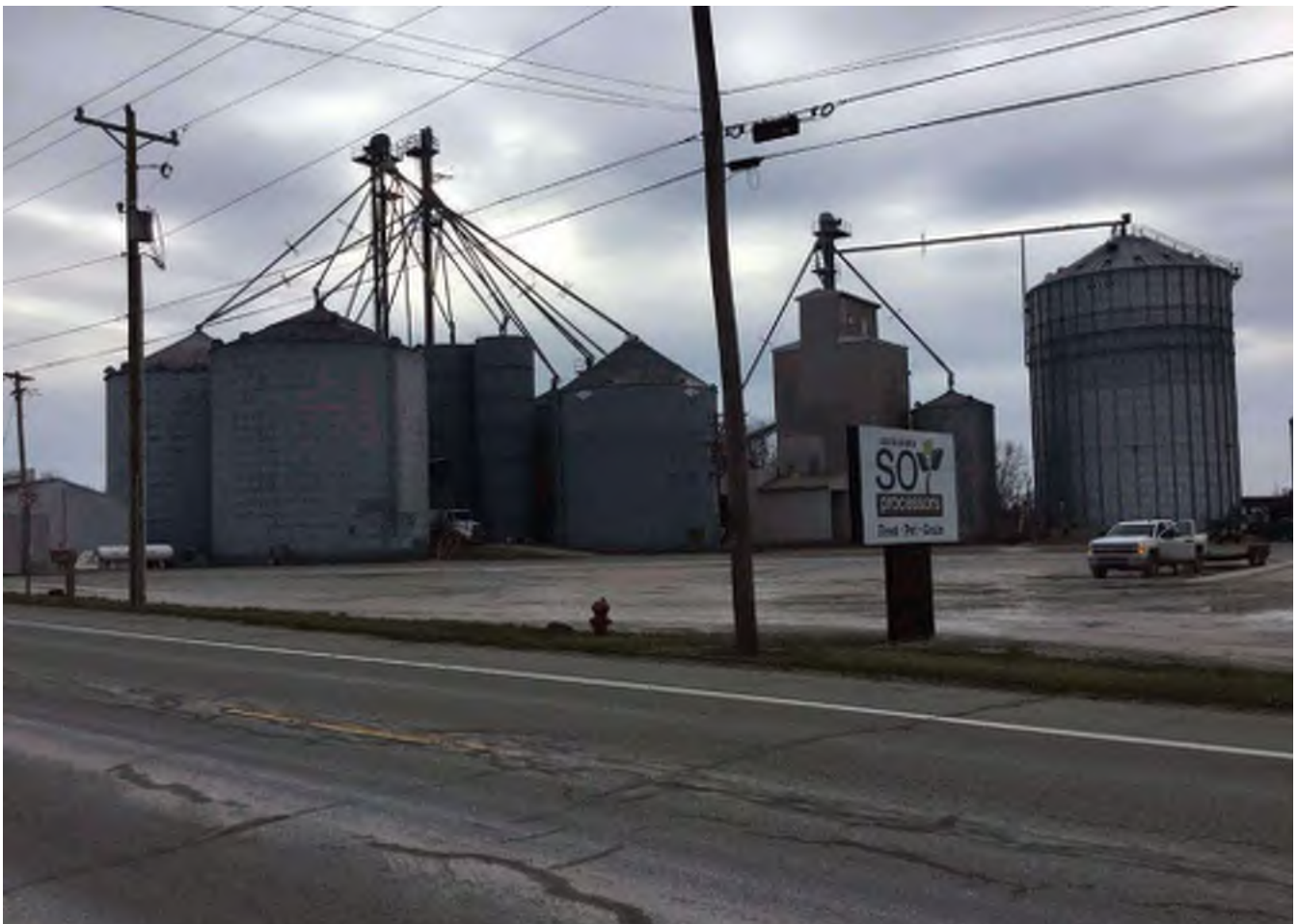
26 Looking southeast at “Contributing” c. 1956 grain elevators (IHSSI # 031-252-24078) at 1015 W. Main Street (SR 46).
