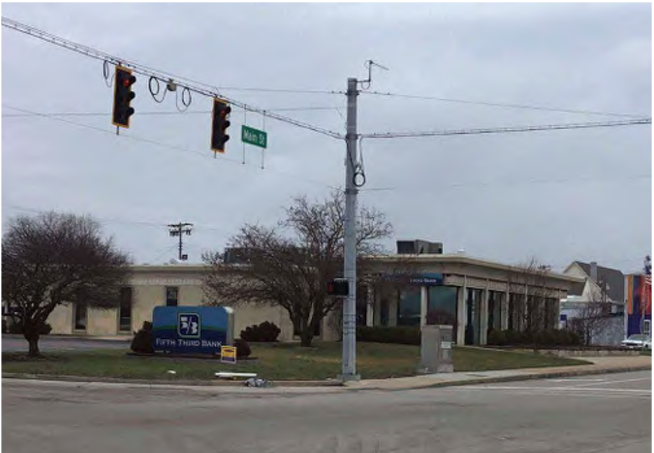
47 Looking northeast across the Main Street (SR 46) and US 421 (Ireland Street) intersection at the c. 1973 “Contributing” bank (RQAW # 8).
