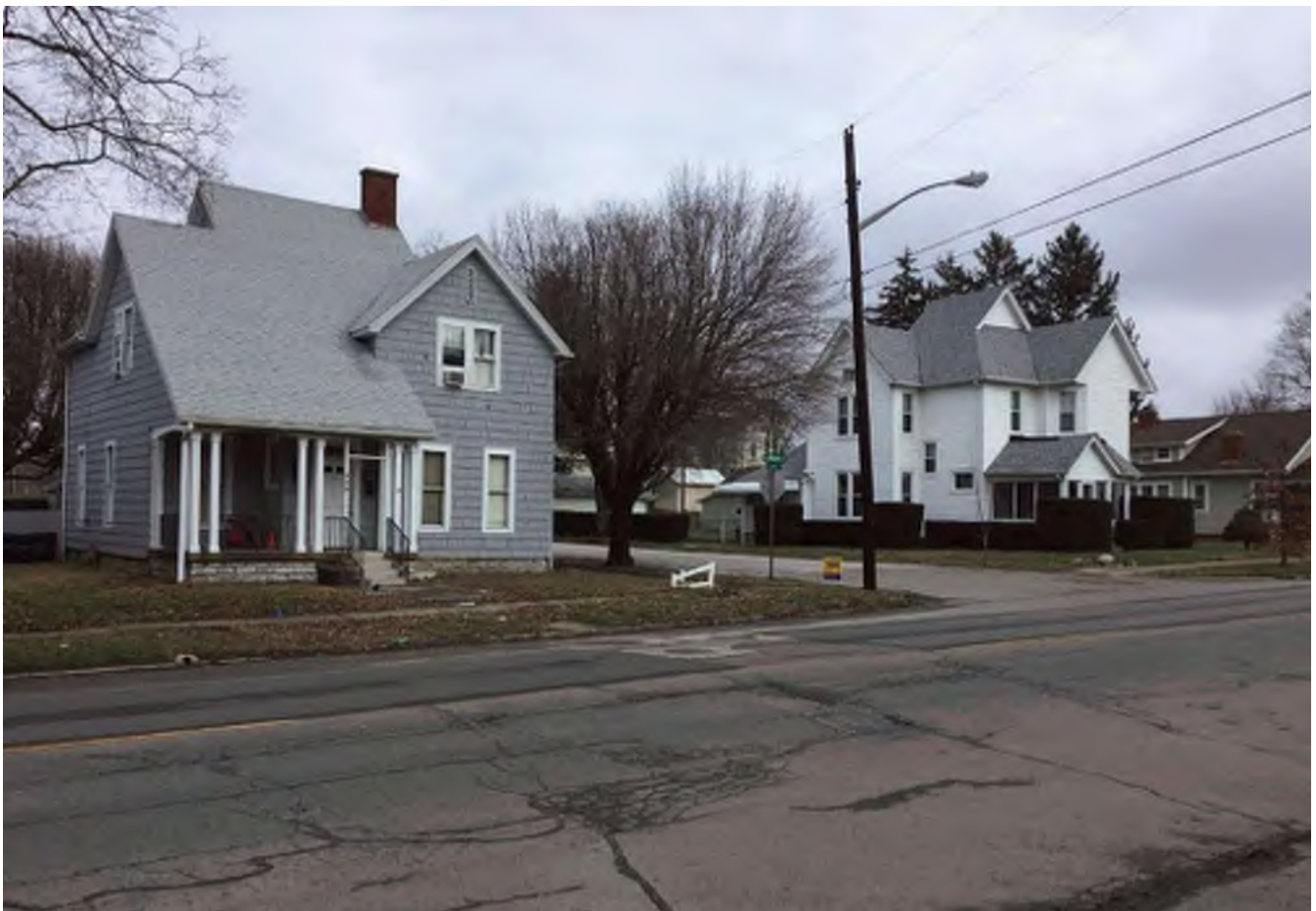
76 Looking northeast at “Contributing” and “Non-contributing” houses at Stewart Street within the recommended National Register-eligible Greensburg Eastside Residential Historic District.
