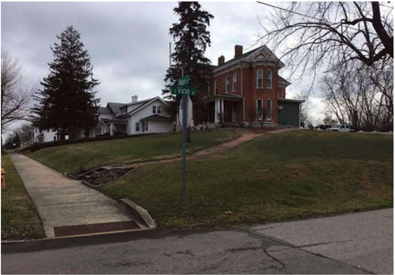
77 Looking southeast across Vine Street at “Notable” and “Contributing” houses within the recommended National Register-eligible Greensburg Eastside Residential Historic District.
