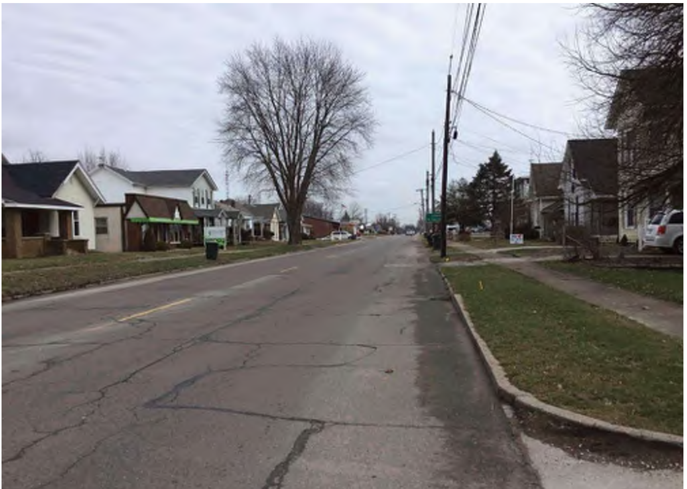
90 Looking east along Main Street.
