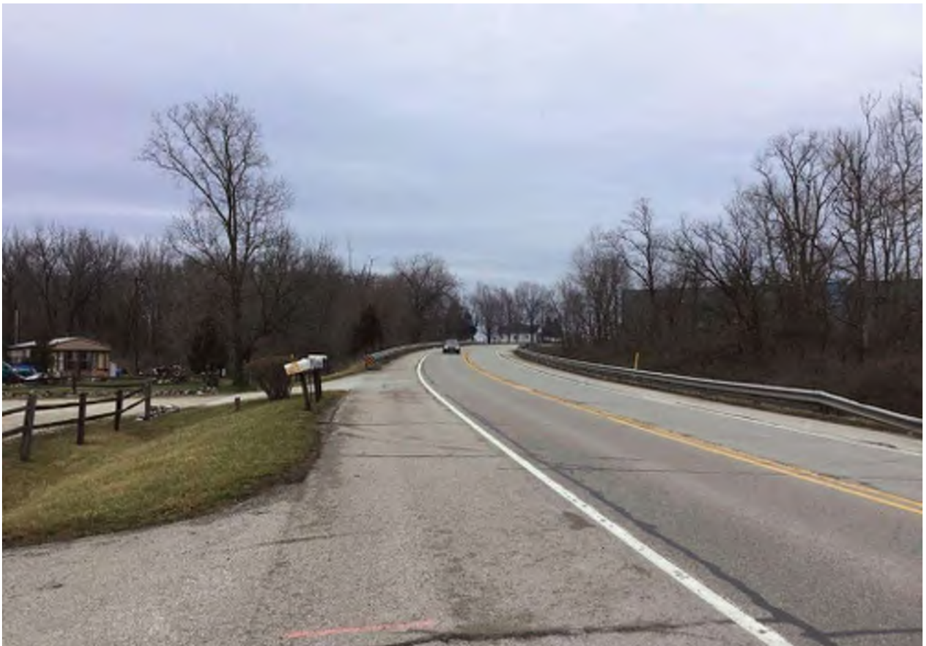
11 Looking east along SR 46 (Main Street) towards bridge over Muddy Fork Sand Creek [Bridge No. 046-16-00945 / NBI No. 17400] (RQAW #3).
