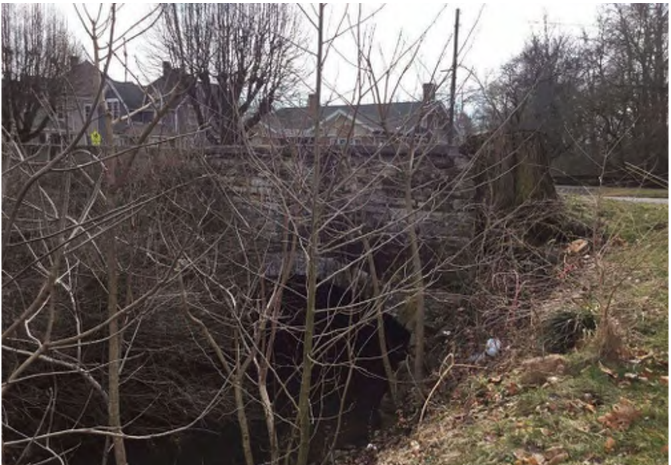
60. February 2020 photo looking southeast at stone arch bridge, a “Contributing” structure to the Greensburg Eastside Residential Historic District. The bridge was replaced in the summer of 2020.
