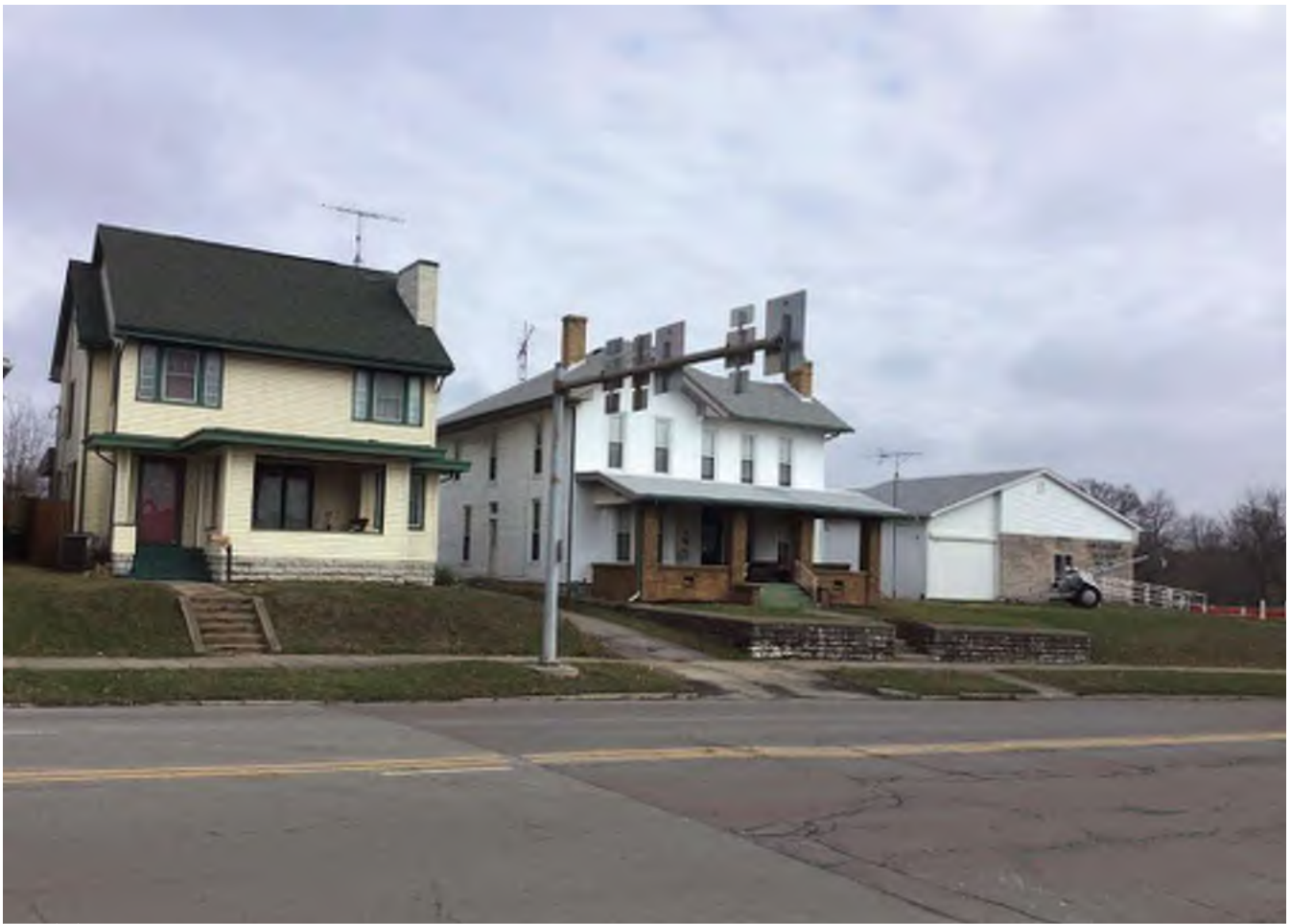
53 Looking northeast at “Non-contributing” buildings at 316, 322, and 326 E. Main Street with alterations.
