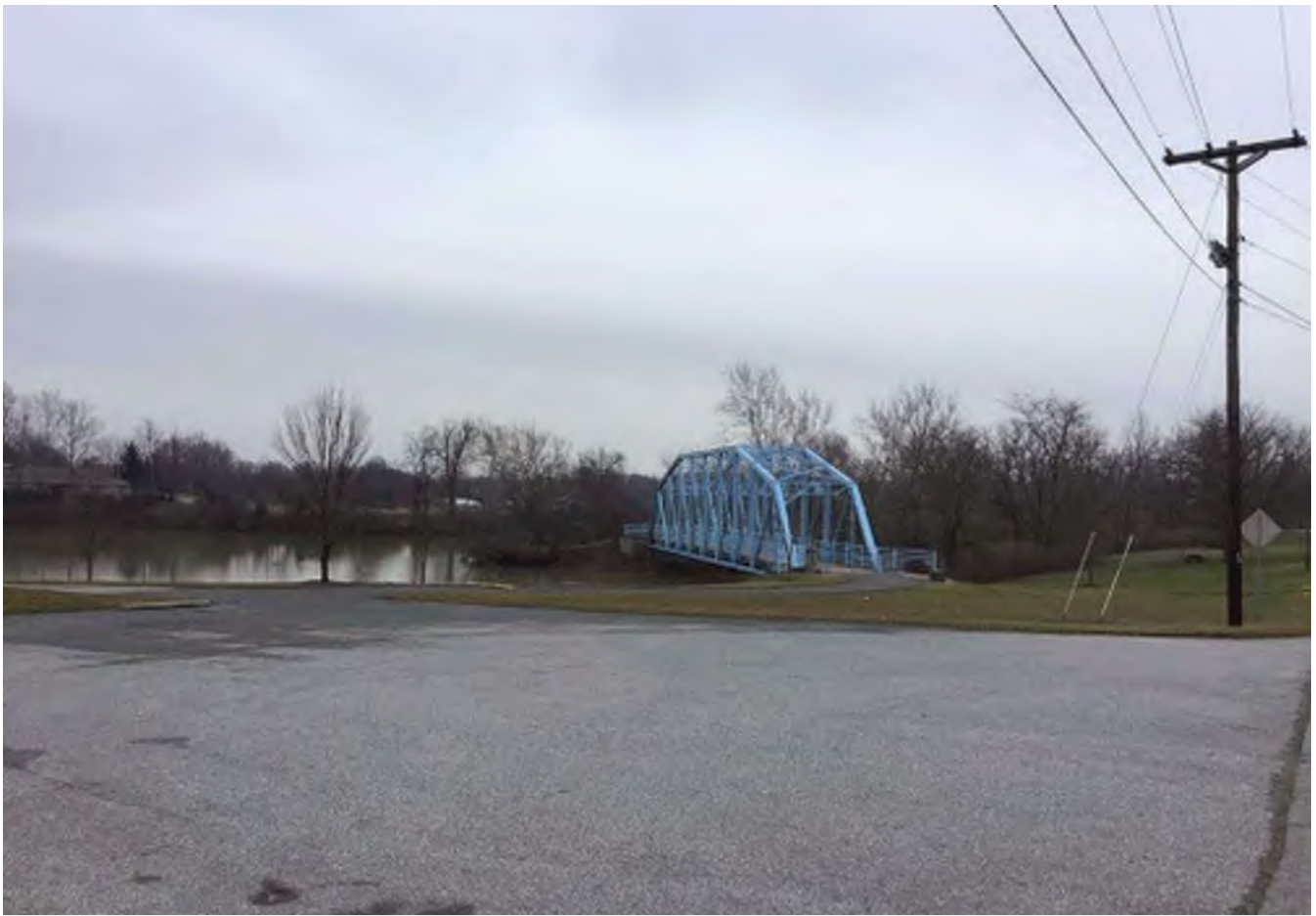
5 Looking southeast outside of the APE at the 1915 pedestrian steel truss “Boyd Bridge” (Decatur County Bridge 140, NBI 1600116) relocated in 2006 over Muddy Fork of Sand Creek in Decatur County Park at 1650 W. Park Rd.
