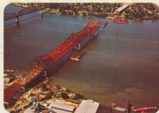
JOHN FITZGERALD KENNEDY MEMORIAL BRIDGE UNDER CONSTRUCTION AT JEFFERSONVILLE
