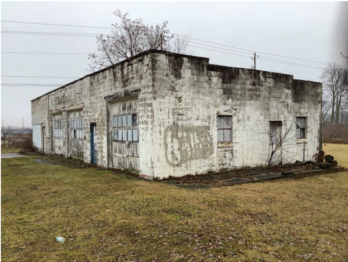
4. Looking SE at Lochmueller #1 (Contributing, 1940 service station)
