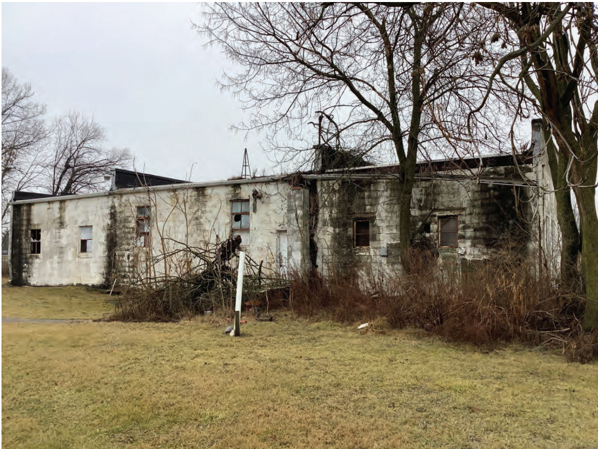
6. Looking NW at Lochmueller #1 (Contributing, 1940 service station)
