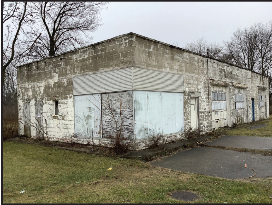
Figure 3: Looking SW at facade and east elevation of building.
