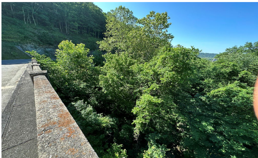
Photo 7: Facing southeast from the center of Park Road the bridge.
