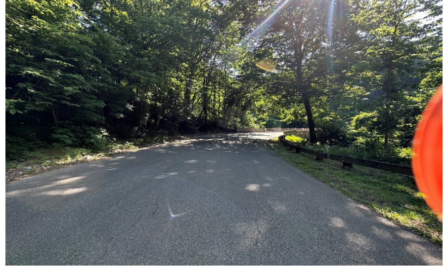
Photo 2: Facing northeast toward Park Road west of the bridge.
