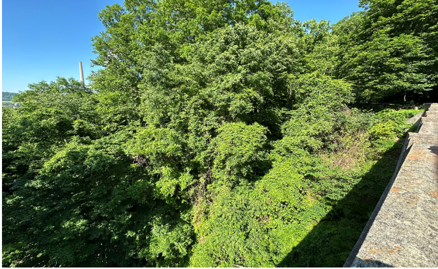
Photo 9: Facing southwest looking at the steep slopes from the center of the bridge.
