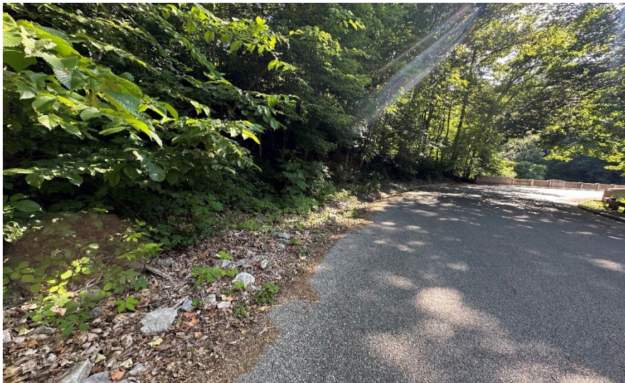
Photo 3: Facing northeast on Park Road west of the bridge.
