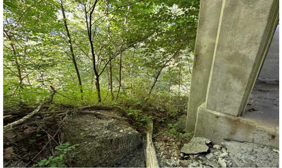
Photo 28: Facing southwest from beneath the bridge.
