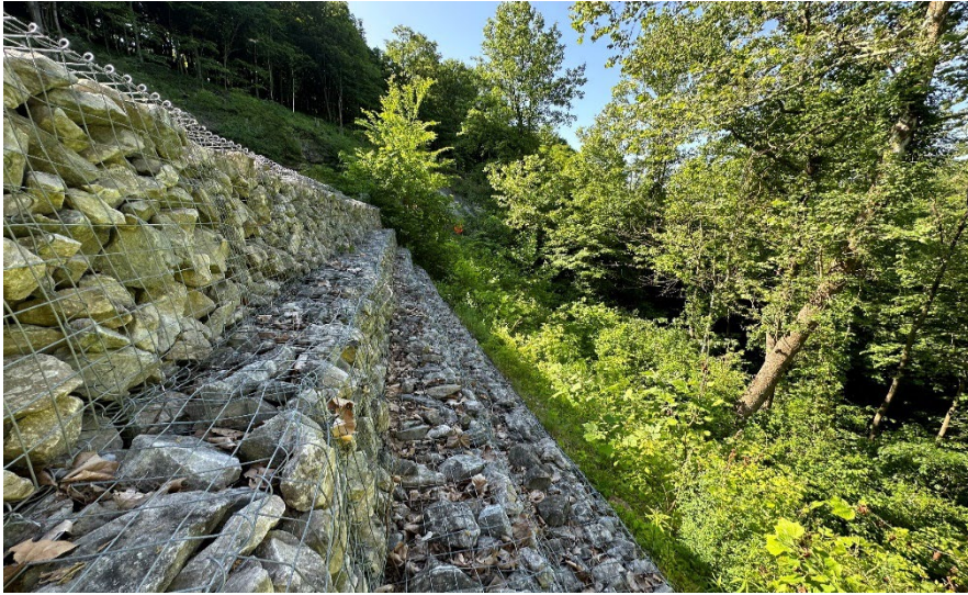
Photo 21: Facing south toward riprap lined slopes southeast of the bridge.
