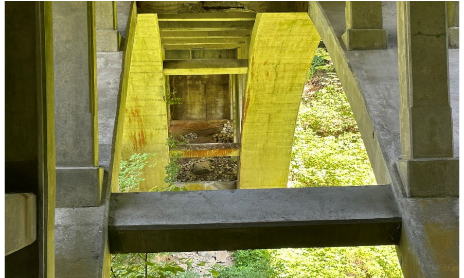
Photo 24: Facing northwest from beneath the bridge.
