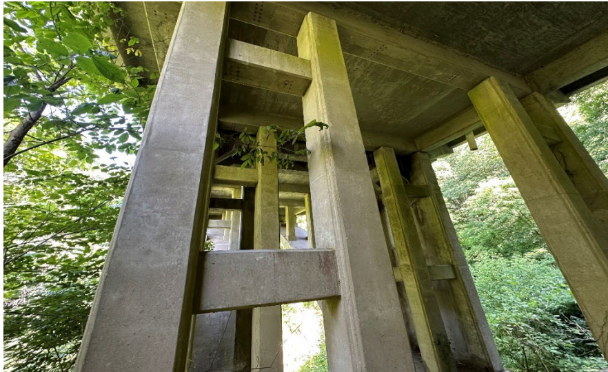
Photo 23: Facing northwest looking up at the bridge beneath Park Road.
