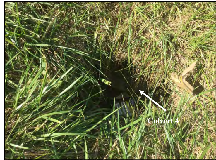
24. View of Culvert 4, looking southwest.
