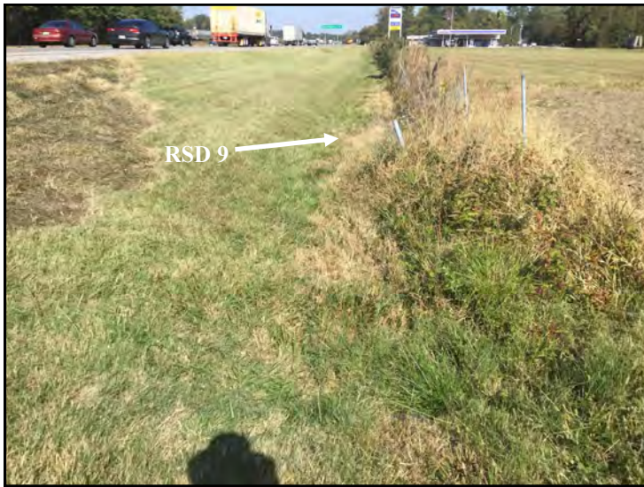
65. View of RSD 9 from Culvert 13 at southern PSL, looking northwest.
