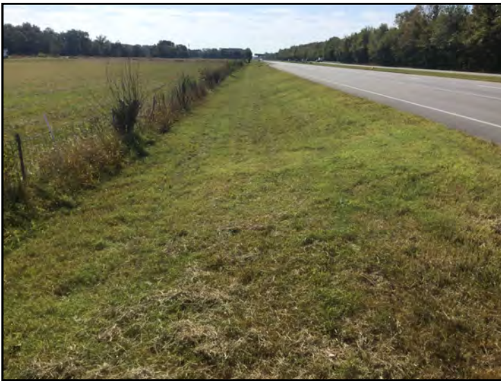
53. View of U.S. 41 ROW, looking southeast.
