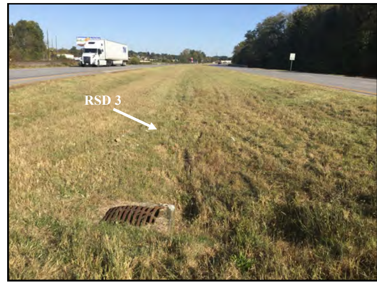
22. View of Culvert 3 and RSD 3, looking northwest.
