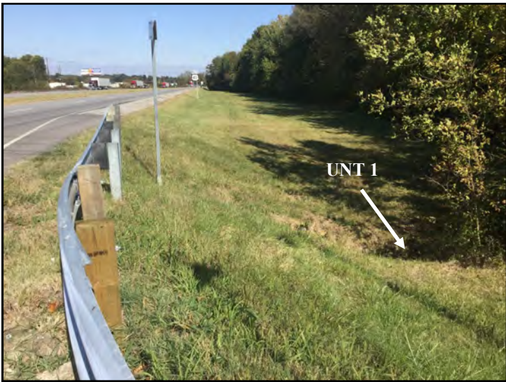
37. View of UNT 1 and U.S. 41 right-of-way (ROW), looking northwest.
