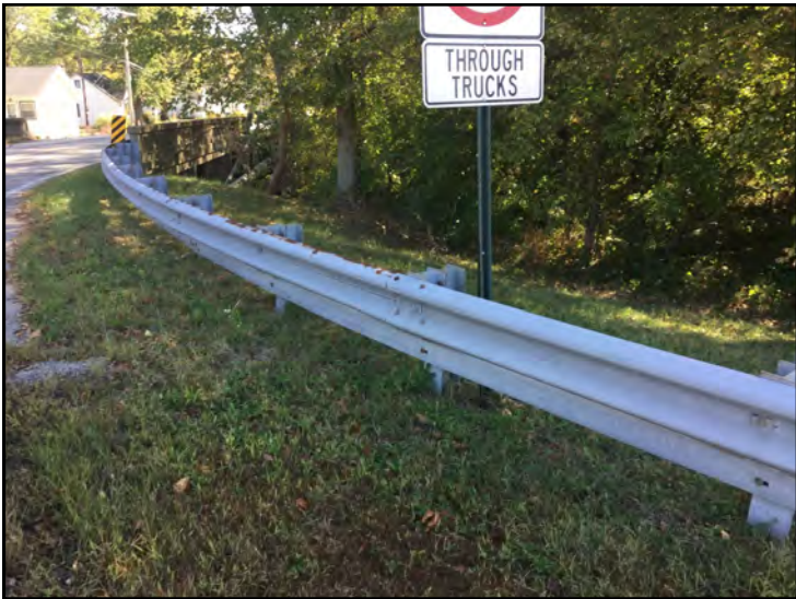
39. View of Hillsdale Rd. ROW, looking northeast.
