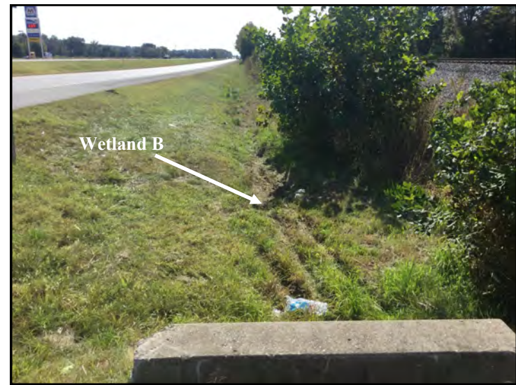
42. View of Wetland B from Culvert 6, looking southeast.
