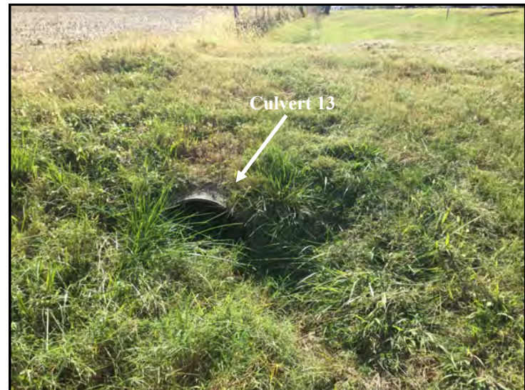
64. View of Culvert 13, looking southeast.
