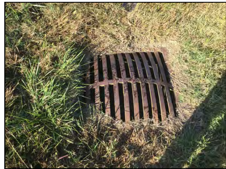
34. View of Culvert 7.
