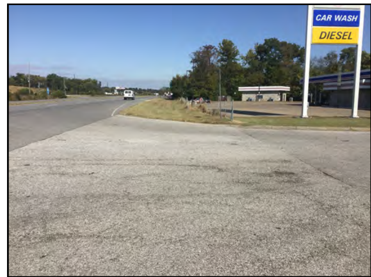
52. View of U.S. 41 ROW, looking northwest.
