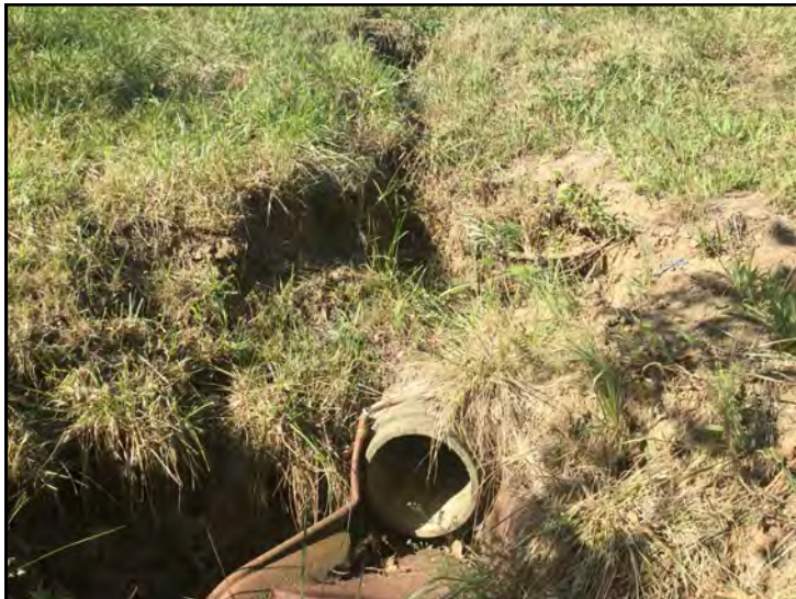
35. View of Culvert 8, looking southwest.
