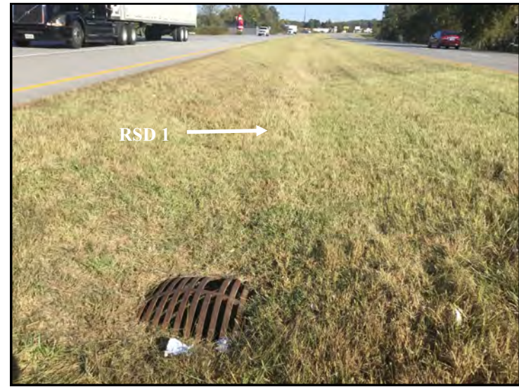
2. View of Culvert 1 and RSD 1, looking northwest.
