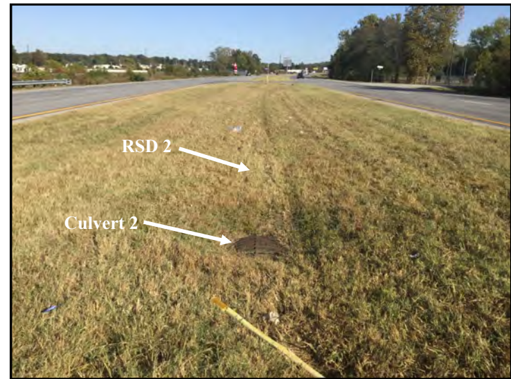
4. View of Culvert 2 and RSD 2, looking northwest.
