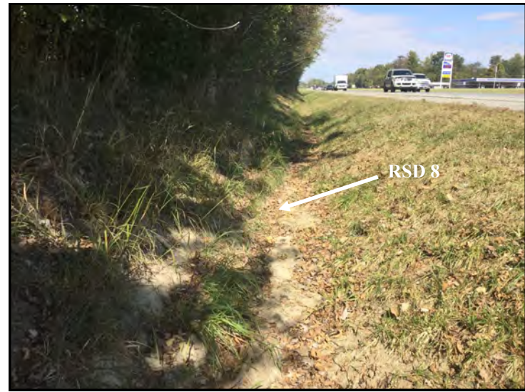
62. View of RSD 8 from southern PSL, looking northwest.
