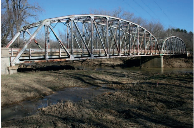
Historic structures require consultation with various stakeholders.
