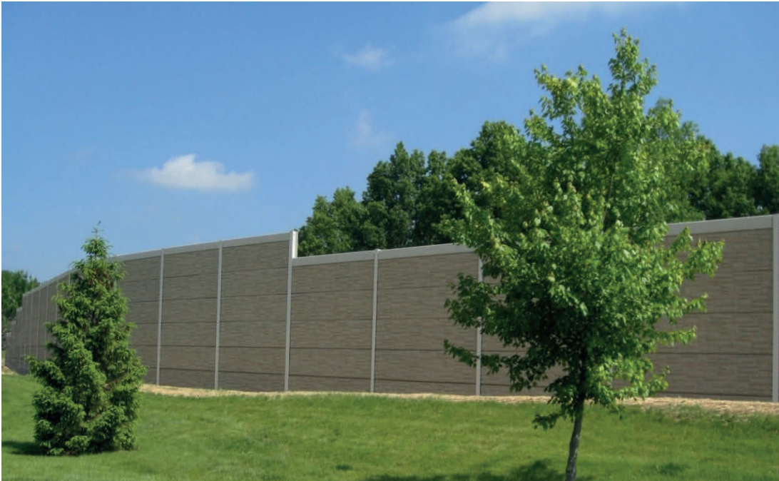
An example of a noise barrier.
