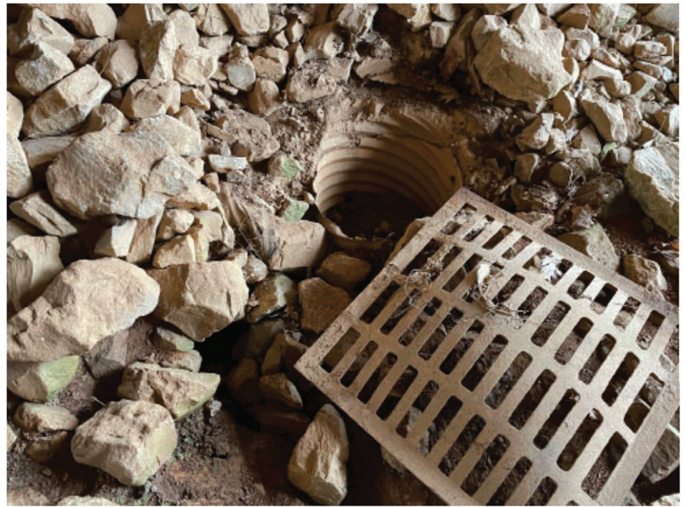
14. Looking north to Swallet 1 with grate removed, beneath bridge carrying SR 64
