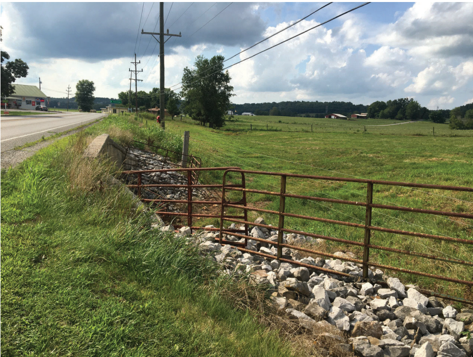
15. Looking west to SR 64 bridge
