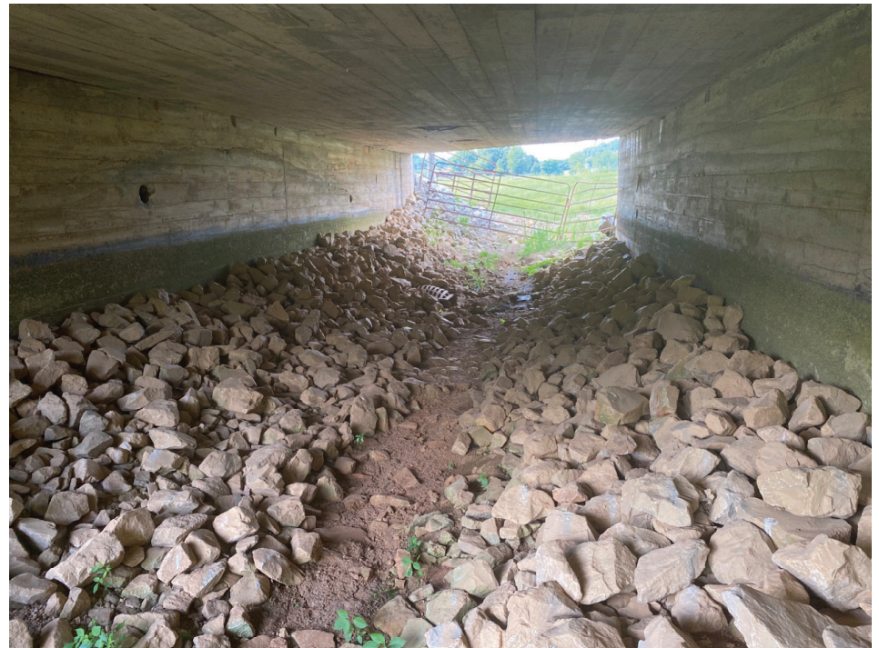
12. Looking north to space beneath bridge carrying SR 64
