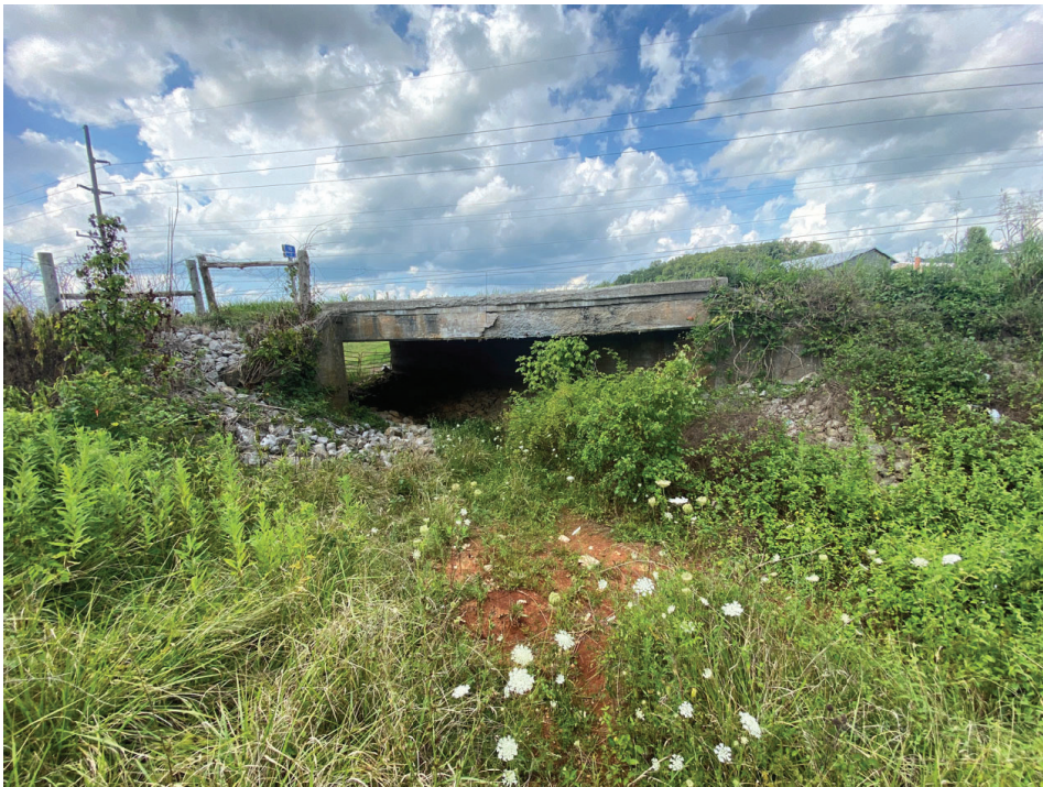
9. Looking north to bridge carrying SR 64
