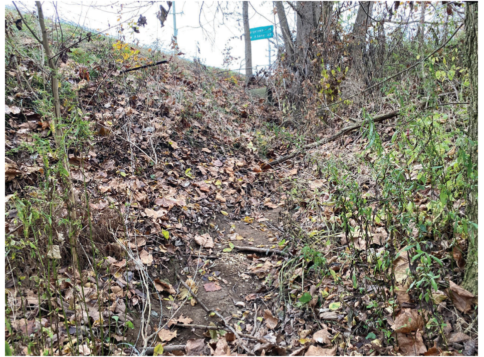
2. Looking southeast upslope to culvert outlet
