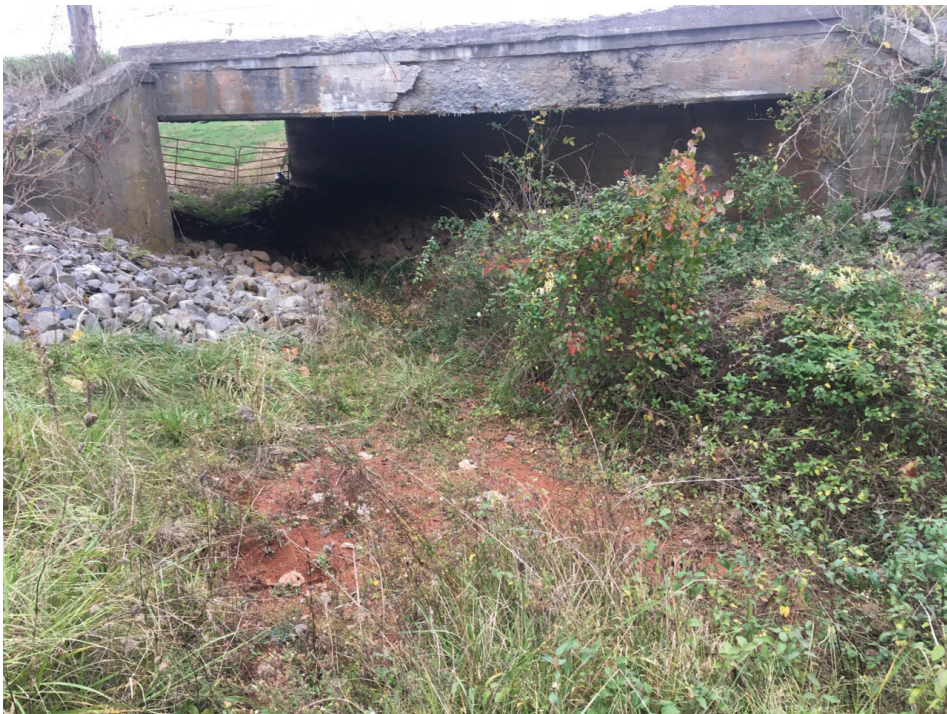
7. Looking north to underside of SR 64 bridge
