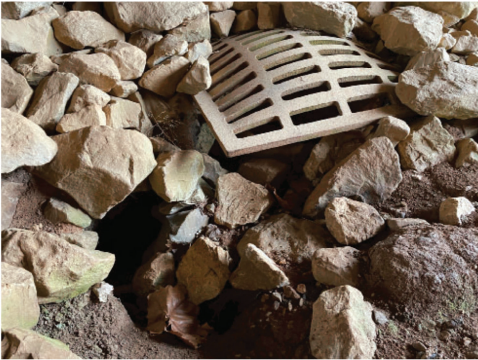
13. Looking north to Swallet 1, beneath bridge carrying SR 64
