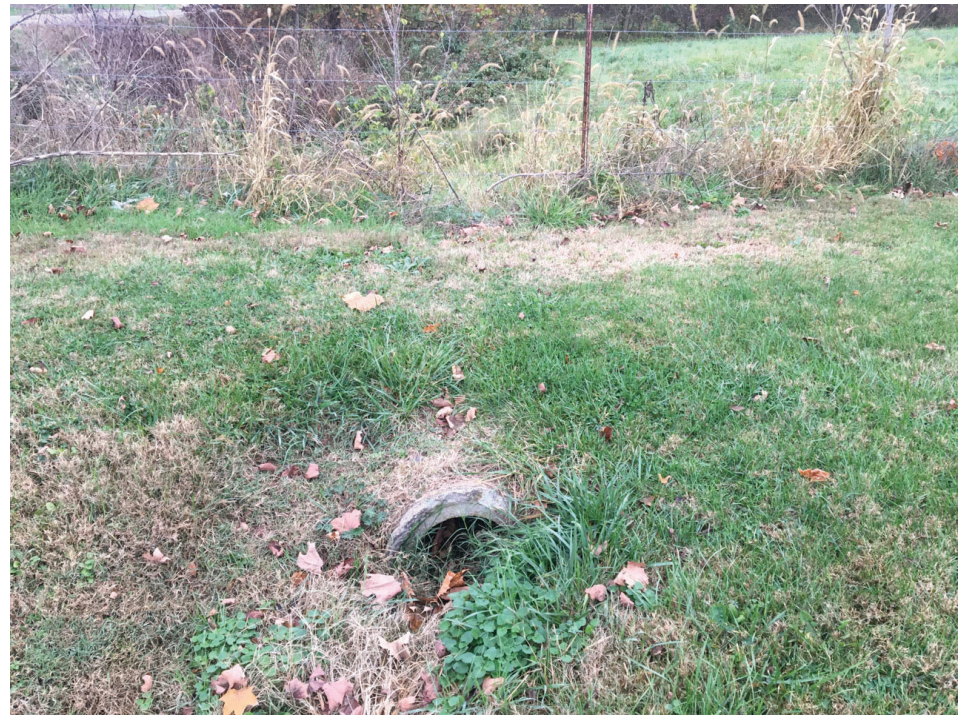
10. Facing small structure on south side of SR 64
