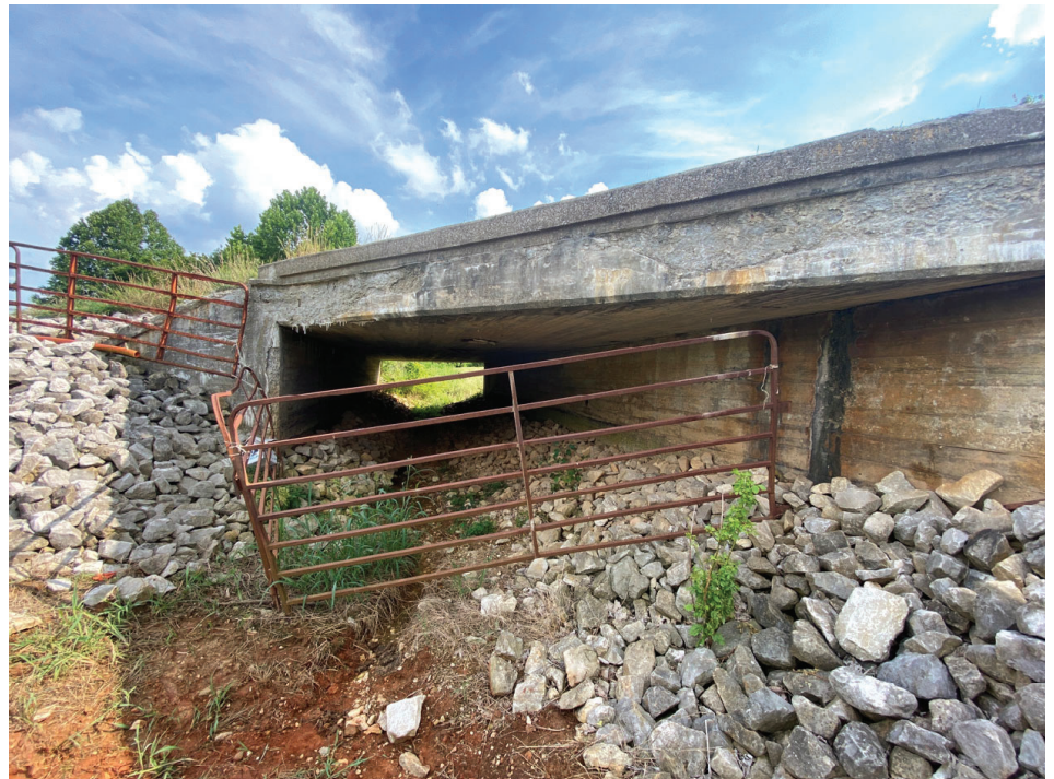
16. Looking south beneath SR 64 bridge
