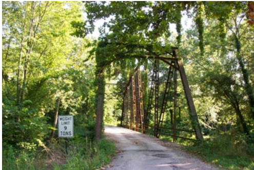
Pike 20005-Bridge No. 81, view southwest.
