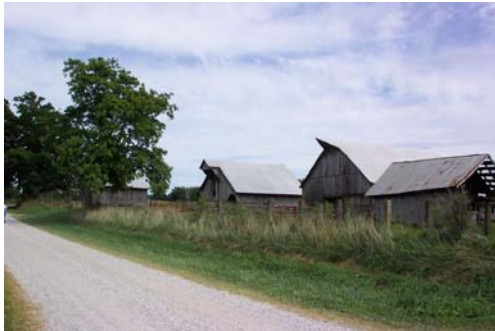
Daviess 35001-Chapman-Allison Farmstead, view southeast.
