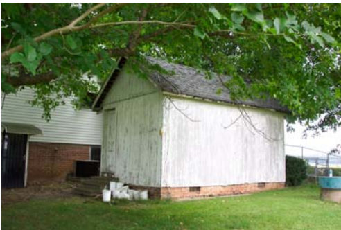
Pike 20001-Well house, view northeast.
