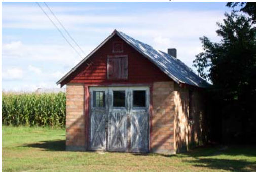
Daviess 30037-tile block garage, view northwest.
