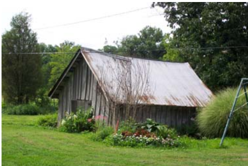
Daviess 35001-East shed, view northwest.
