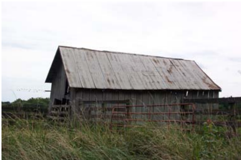
Daviess 35001-Front-gabled outbuilding, view southwest.
