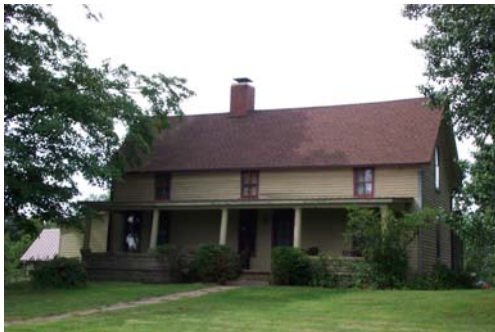
Daviess 35001-House, view northwest.
