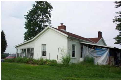
Daviess 30030-House, view southwest showing north porch.
