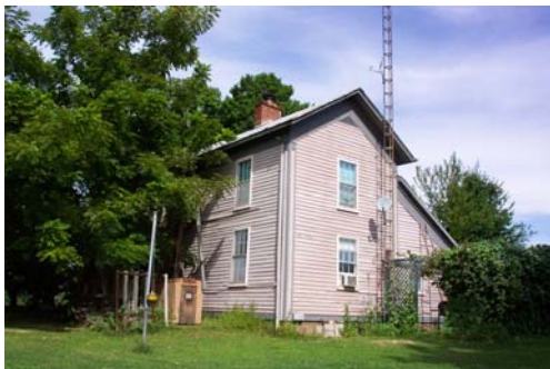
Pike 05011-House, view northwest.
