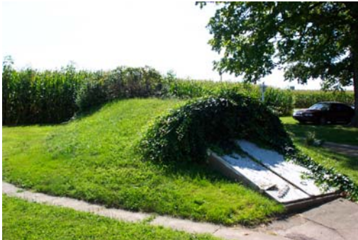
Daviess 30037-storm cellar, view southeast.
