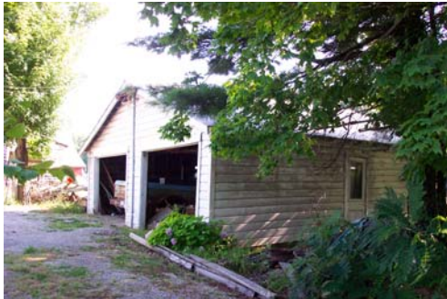
Gibson 30005-Garage, view southeast.
