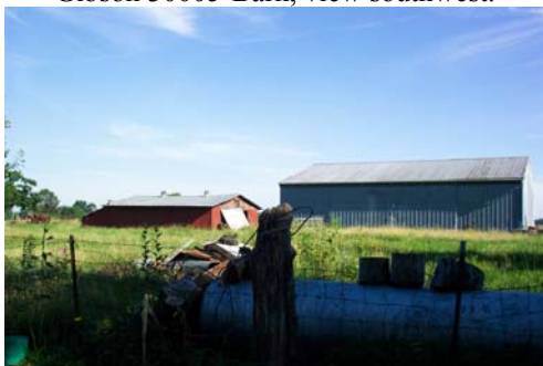
Gibson 30005-Pole barn and hog house, view southeast.
