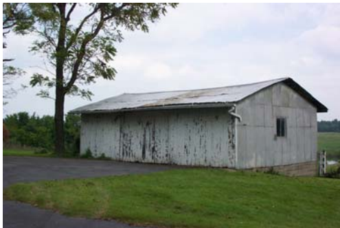
Pike 20001-Garage, view northeast.
