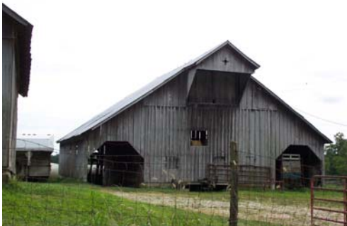
Daviess 35001-Three-portal barn, view southwest.
