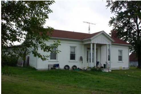
Daviess 30030-House, view southeast.
