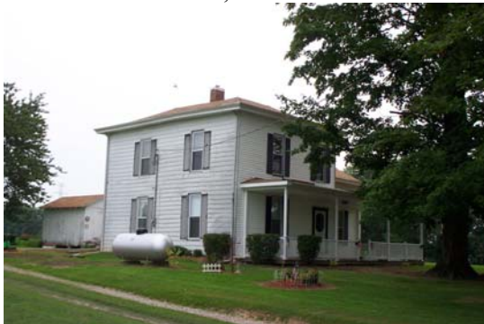
Pike 05010-House, view northeast.
