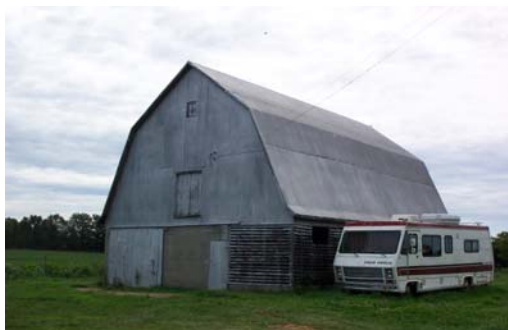
Pike 05004-Barn, view southeast.
