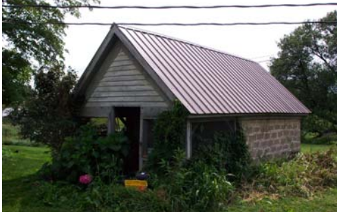
Daviess 35001-Concrete block outbuilding, view southwest.
