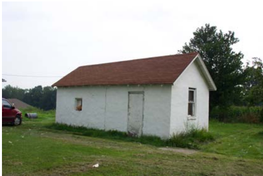
Daviess 30030-Summer kitchen, view northeast.
