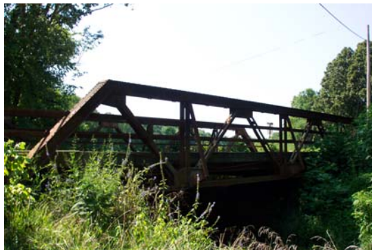
Pike 05002-Bridge, view northwest.
