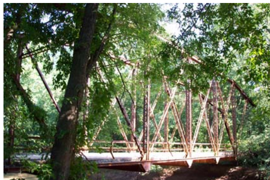
Pike 20006-Bridge, view southwest.
