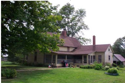
Daviess 35001-House, view southwest.
