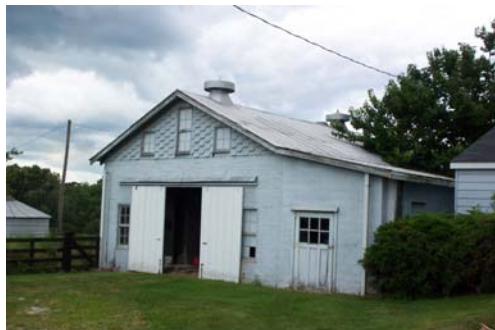
Daviess 35007-Garage/workshop, view southwest.
