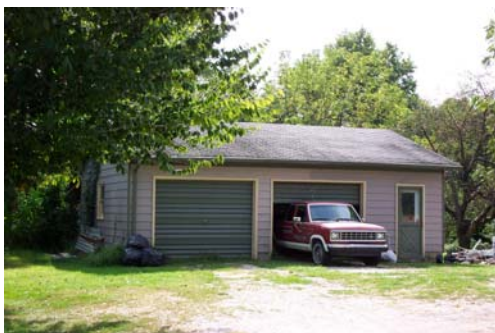
Pike 05011-Garage, view east.
