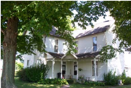
Daviess 30037-house, view northwest.
