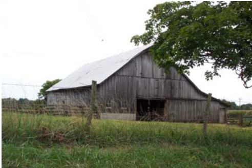
Daviess 35001-Transverse frame barn, view southwest.
