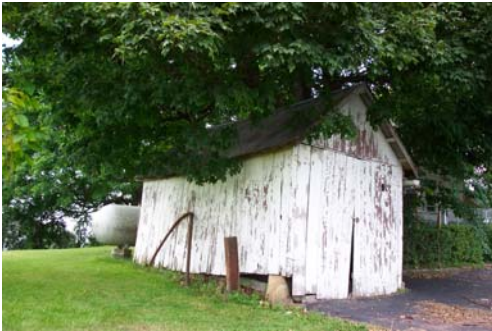
Pike 20001-Shed, view northwest.
