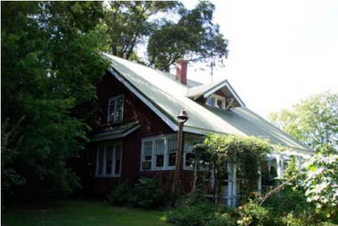
Pike 05005-House, view northwest.
