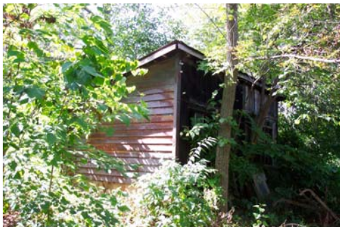
Pike 05005-Brooder house, view northwest.
