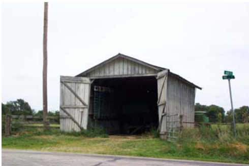
Daviess 35001-Machine shed, view northeast.
