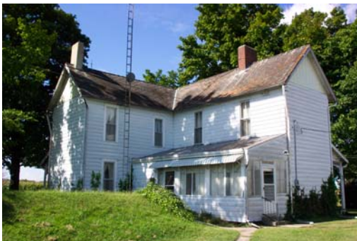
Daviess 30037-house, view southwest.
