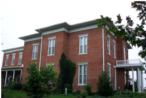
Pike 05006-House, view south.
