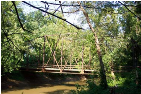
Pike 20005-Bridge No. 81, view northeast.
