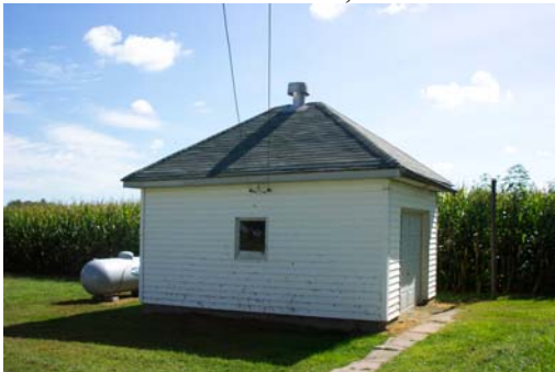
Daviess 30037-wood-frame garage, view northeast.
