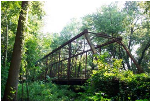
Pike 20005-Bridge No. 246, view southwest.
