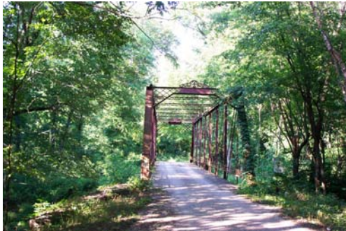
Pike 20005-Bridge No. 246 and County Road 300 West, view northeast.
