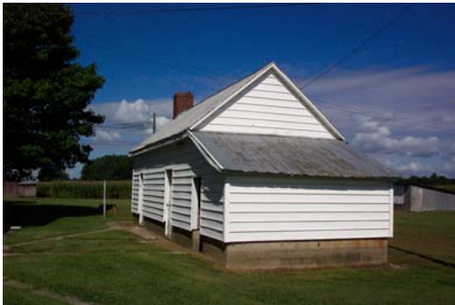
Daviess 30037-summer kitchen, view northwest.
