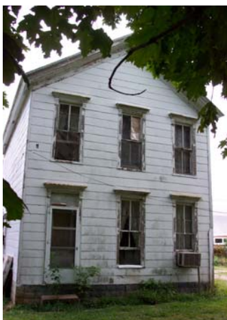
Pike 05004-House, façade, view east.
