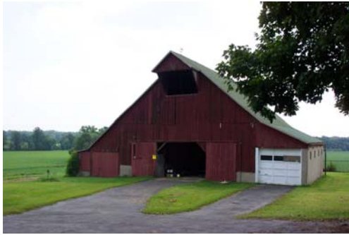
Pike 20001-Three-portal barn, view southeast.
