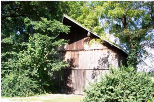
Pike 05005-Transverse frame barn, view east.
