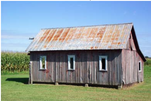
Davie's 30037-workshop, view northwest.
