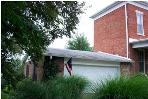
Pike 05006-House, garage, view west.
