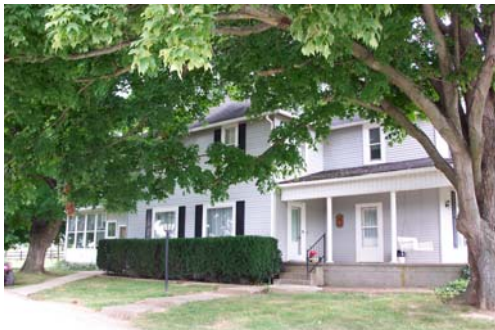
Daviess 35007-House, view northwest.
