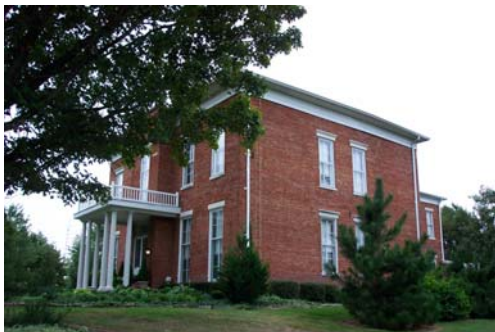
Pike 05006-House, view east.
