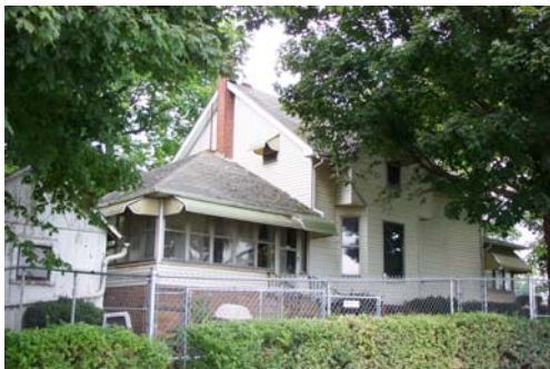
Pike 20001-House, view northwest.
