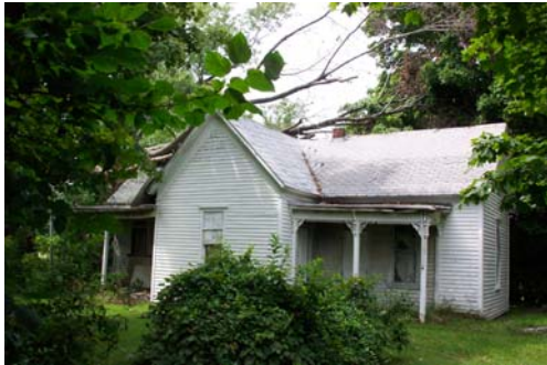
Pike 20009-House, view northwest.
