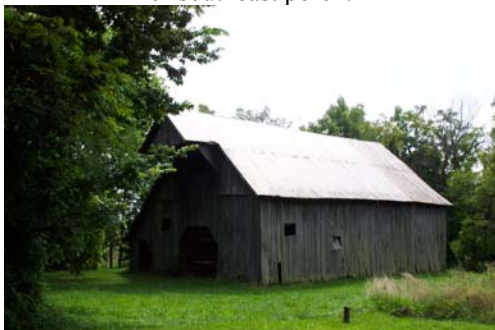
Pike 20009-Transverse frame barn, view southwest.
