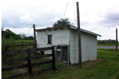
Daviess 35007-North hog house, view northwest.
