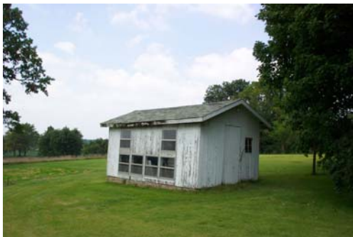
Pike 20001-North poultry house, view northwest.
