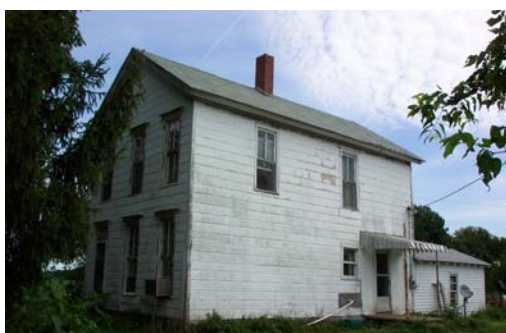
Pike 05004-House, view northeast.
