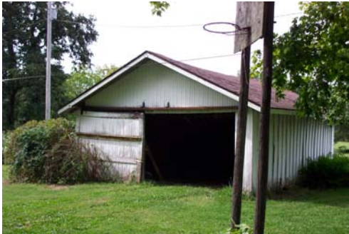
Daviess 35001-Garage, view northwest.
