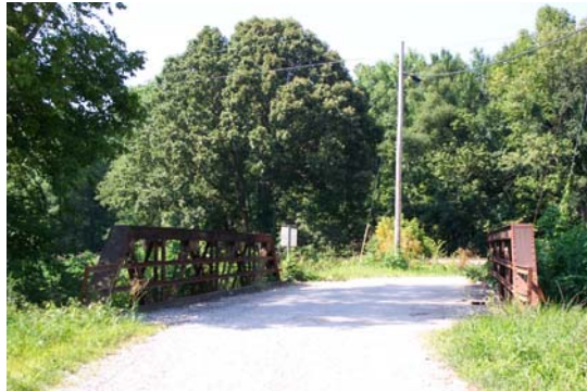
Pike 05002-Bridge, view northeast.
