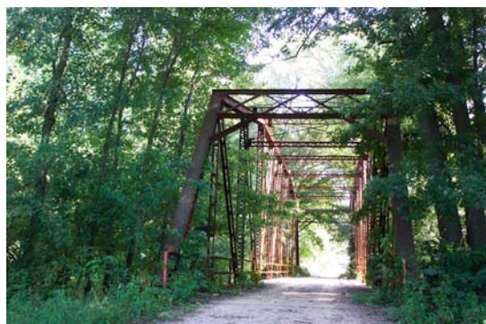
Pike 20006-Bridge, view south.
