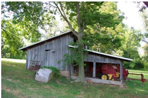
Pike 05005-North poultry house, view north.
