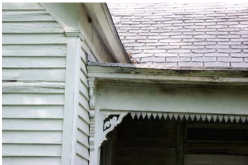
Pike 20009-House, detail of cornerboard and trim of southeast porch.
