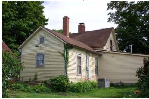
Daviess 35001-House, kitchen ell and addition, view southeast.
