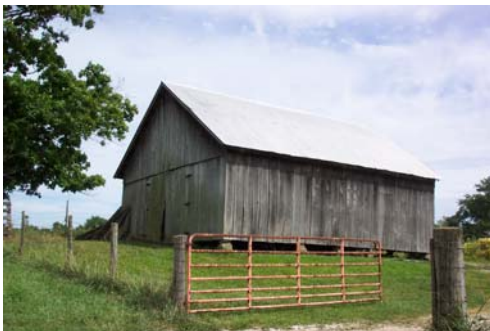
Daviess 35001-Granary, view southeast.
