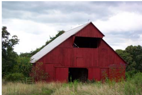
Daviess 35007-Barn, view southwest.
