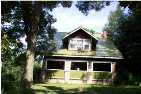
Pike 05005-House, view east.
