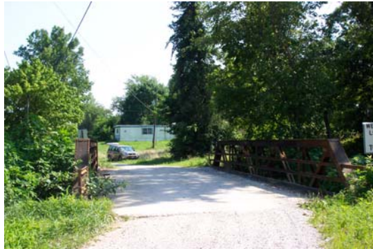
Pike 05002-Bridge, view southwest.
