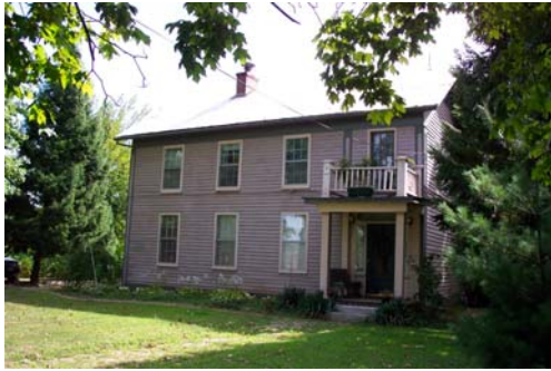
Pike 05011-House, view northeast.
