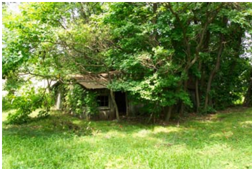
Pike 20009-Outbuilding, view northeast.
