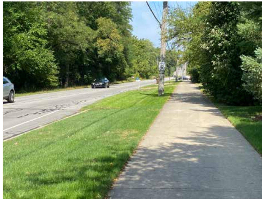
Lakewood Link in Valparaiso. This is an example of a sidepath along a major street, in this case Campbell Street leading to a major park. This would eventually be incorporated into the Dunes Kankakee Regional Trail
