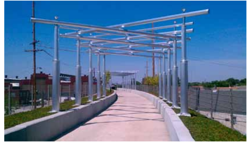
George Lake Bridge. Photo by Mitch Barloga.
