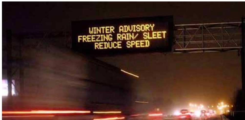
Example of an electronic alert sign on westbound Borman Expressway. Photo from INDOT.
