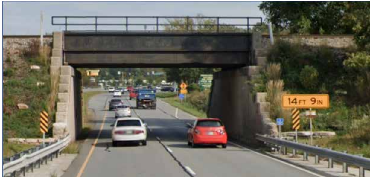
Figure 4-60: Eastbound Bridge View
