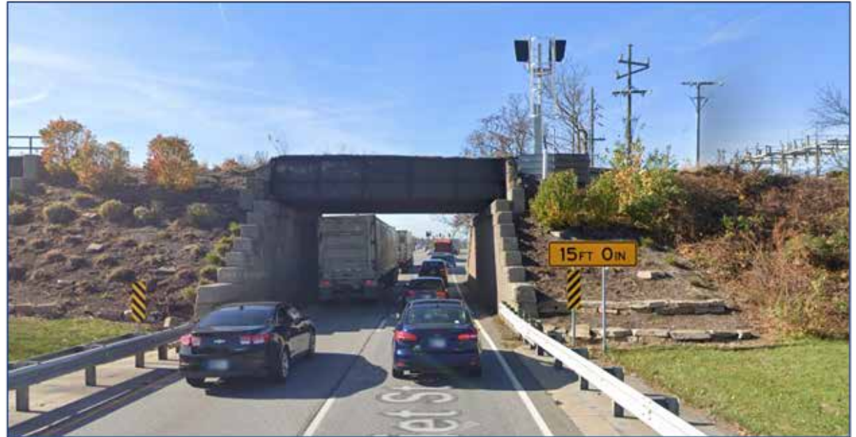
Figure 4-61: Westbound Bridge View
