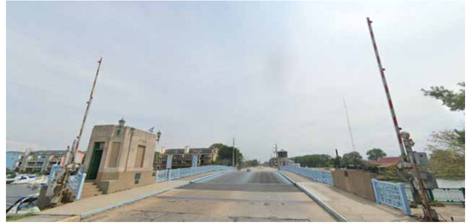
Figure 4-27: Franklin Street Movable Bridge
