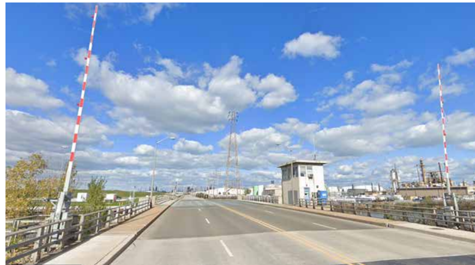
Figure 4-26: Indianapolis Boulevard Movable Bridge
