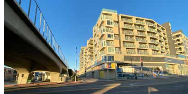
Transit oriented development outside of a city center. Along the Expo Line light rail in Los Angeles.
