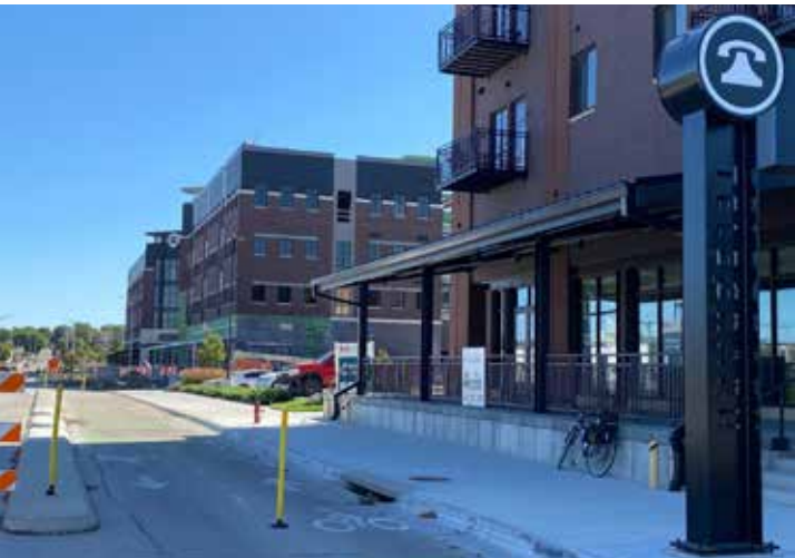
Trails and Development. From top: Trail-oriented development along the Midtown Greenway in Minneapolis; New construction underway
